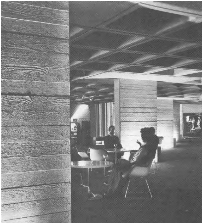
Figure 7.6 (courtesy the Cement and Concrete Association)
