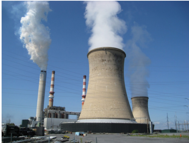
Figure 3-5: Natural draft (hyperbolic) towers.
