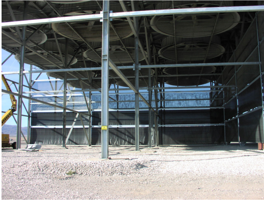
Figure 3-16. Porous windscreen under an ACC.
