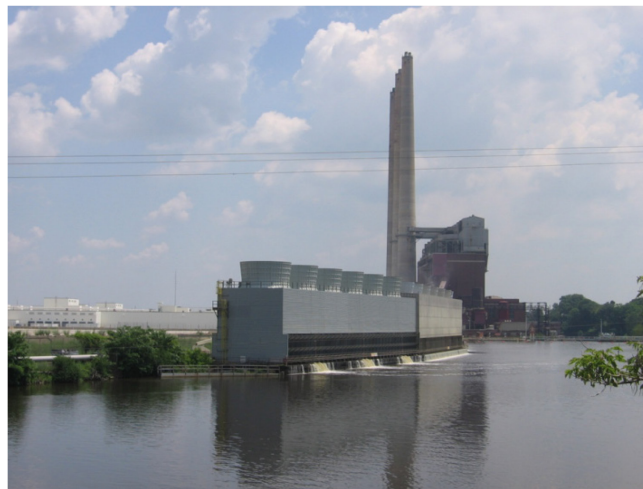
Figure 3-2: Once-through cooling system with helper cooling towers.
