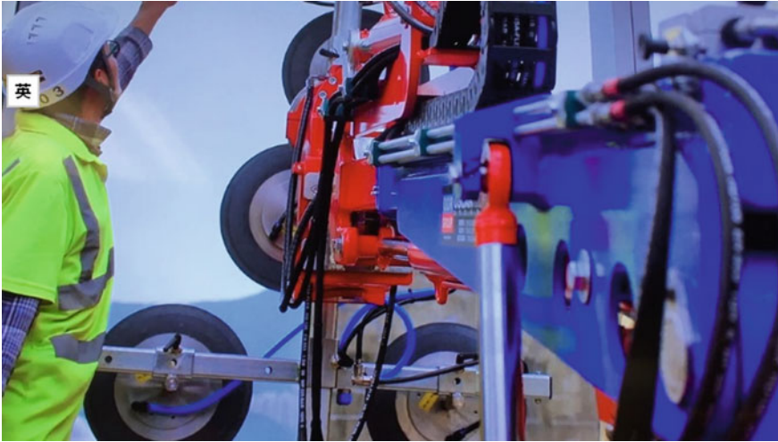
Fig. 13 Large window panels are installed with the help of robots (author's photo)
