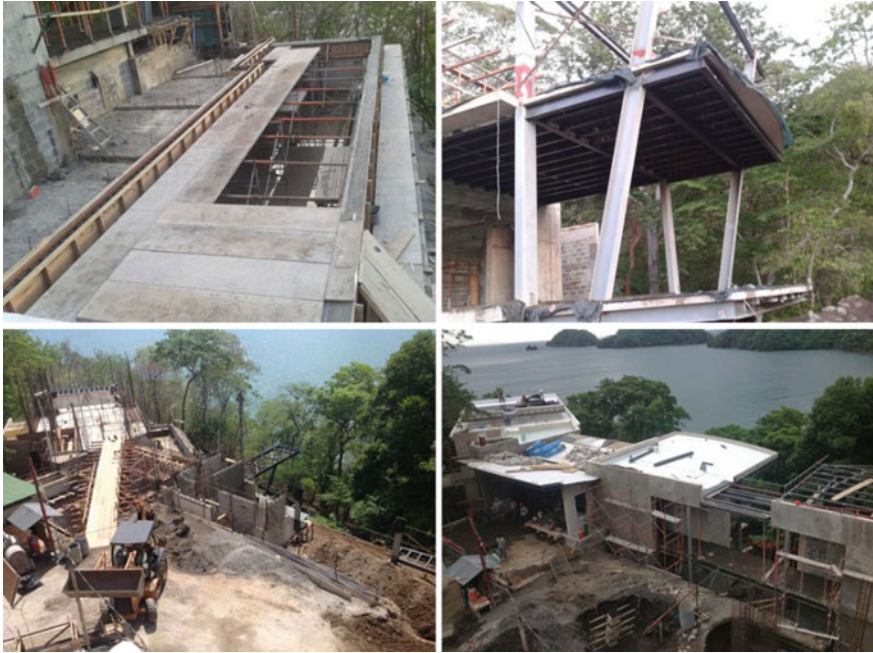
Fig. 18 Construction of the building in progress (Graphisoft 2016)
