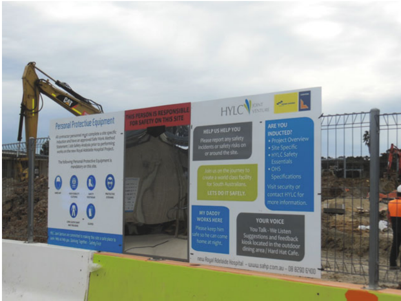
Fig. 11 Poster advocating personal protective equipment at the Royal Adelaide Hospital construction site (author's photo)
