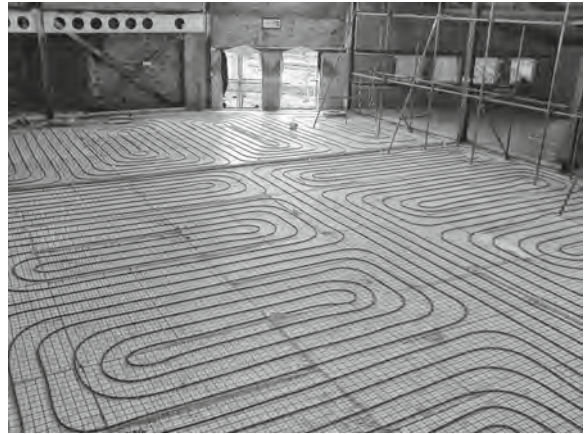
Figure 24.15 Underfloor heating system
