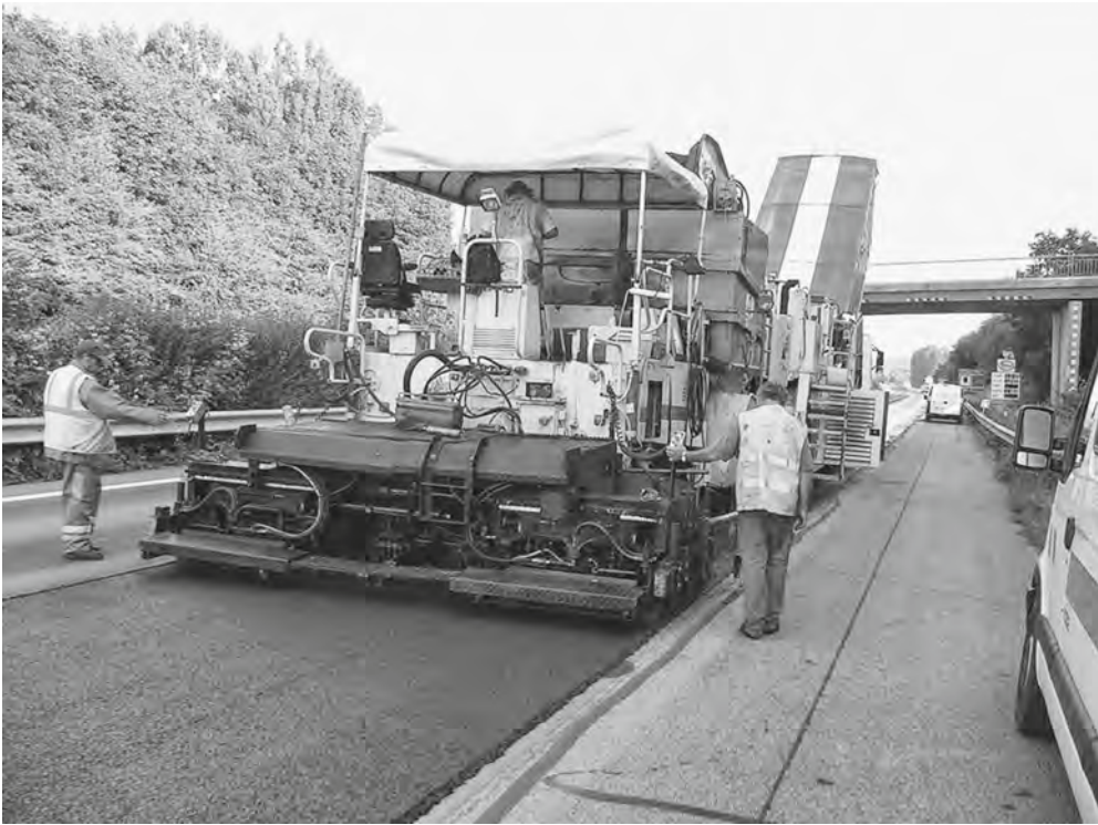
Figure 34.32 An EME2 paving operation
