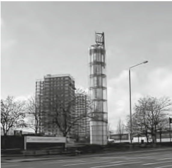
Figure 2.8 The aluminium Thames Water Tower, London
