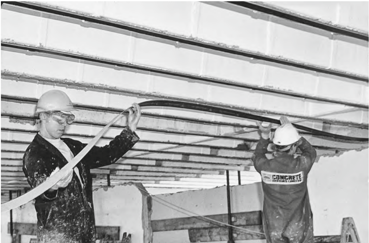
Figure 31.1 Application of an FRP strengthening plate to concrete (courtesy Sika Ltd)
