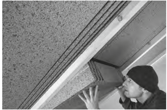
Figure 24.12 Retrofitting insulation in a pitched roof
