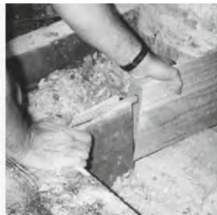
Figure 31.3 Timber beam-end repairs using FRP rods (courtesy Rotafix Ltd)
