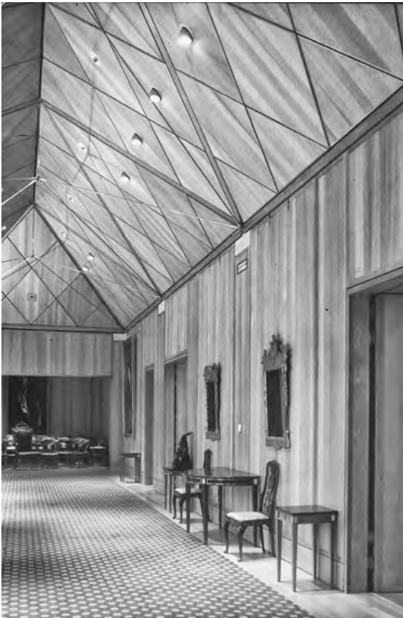
Figure 33.1 Haberdashers' Hall (London) has consistency because both roof trusses and finishes are surfaced in American white oak (Hopkins Architects, Engineer: Arup). © Arup
