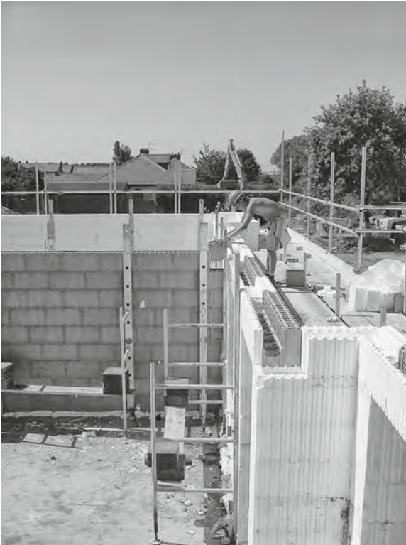
Figure 24.10 An ICF product in construction
