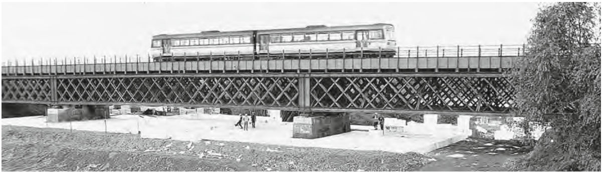
Figure 24.20 Rail embankment during construction with EPS to replace a deteriorating steel bridge
