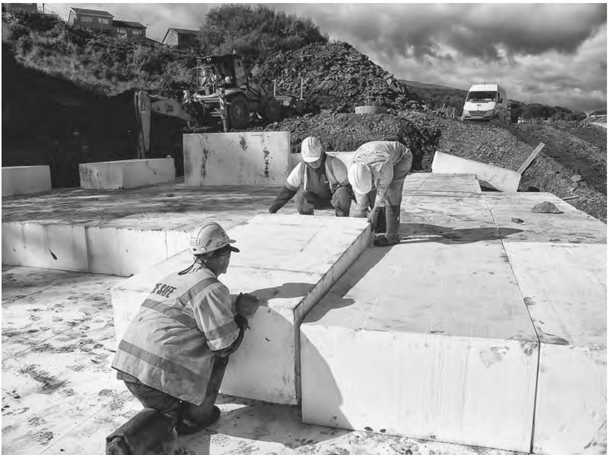
Figure 24.19 Placing EPS blocks in a road foundation
