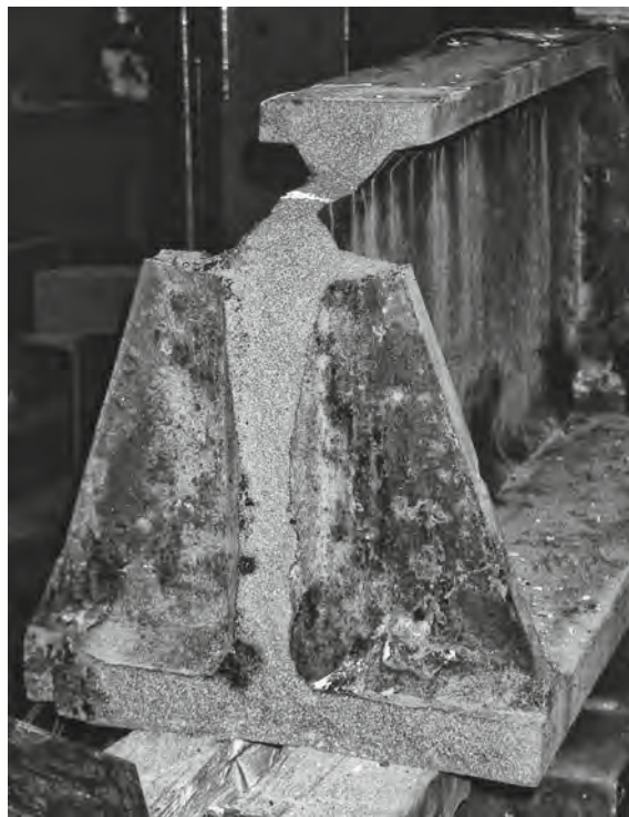
Figure 5.4 Fractured surface of cast iron beam after test to failure, showing dark patches of moulding sand in the grey cast iron matrix
