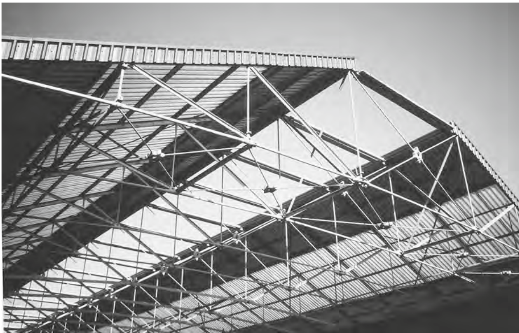
Figure 6.7 Huddersfield Station roof of 1850 – delicate wrought iron trussing
