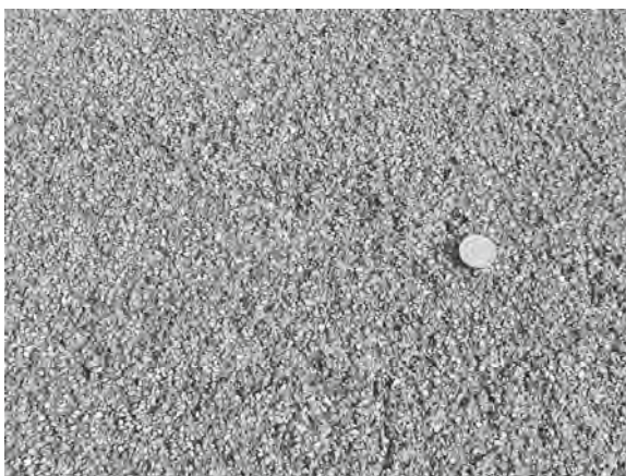
Figure 34.19 Clause 924 High Friction Surfing
