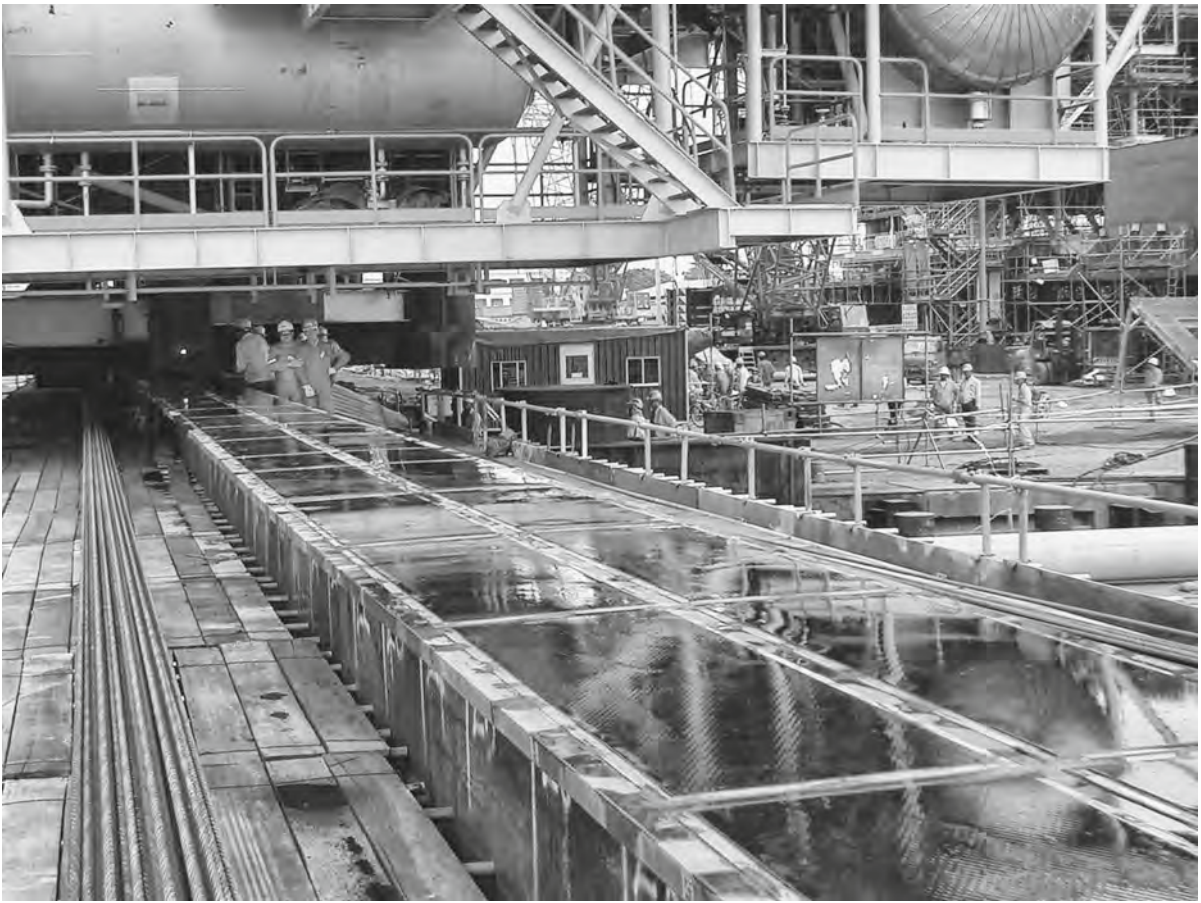
Figure 25.4 Heavy-duty PTFE skidway system (courtesy of Fluorocarbon Co. Ltd)
