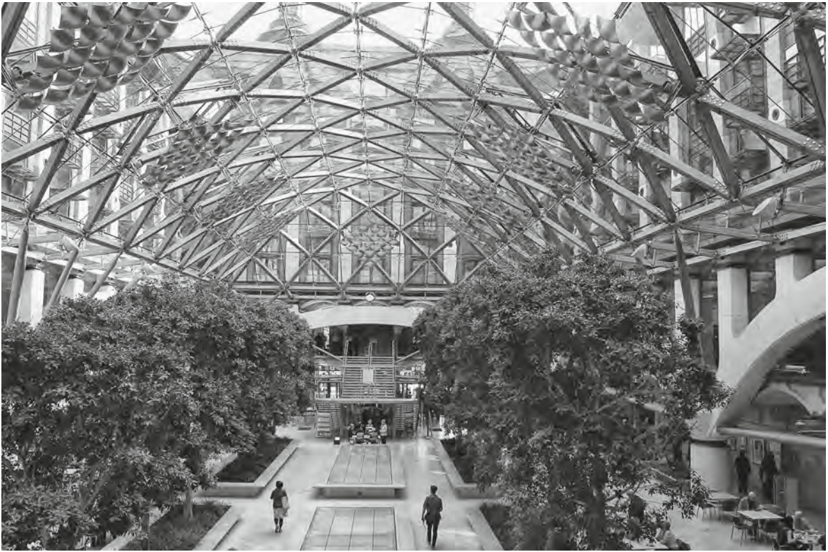
Figure 33.17 The courtyard roof at Portcullis House (London) uses American white oak, selected for its strength and appearance (Hopkins Architects, Engineer: Arup). © Arup
