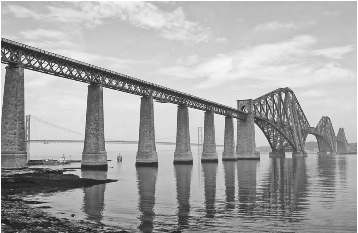
Figure 4.4 The Forth Railway Bridge
