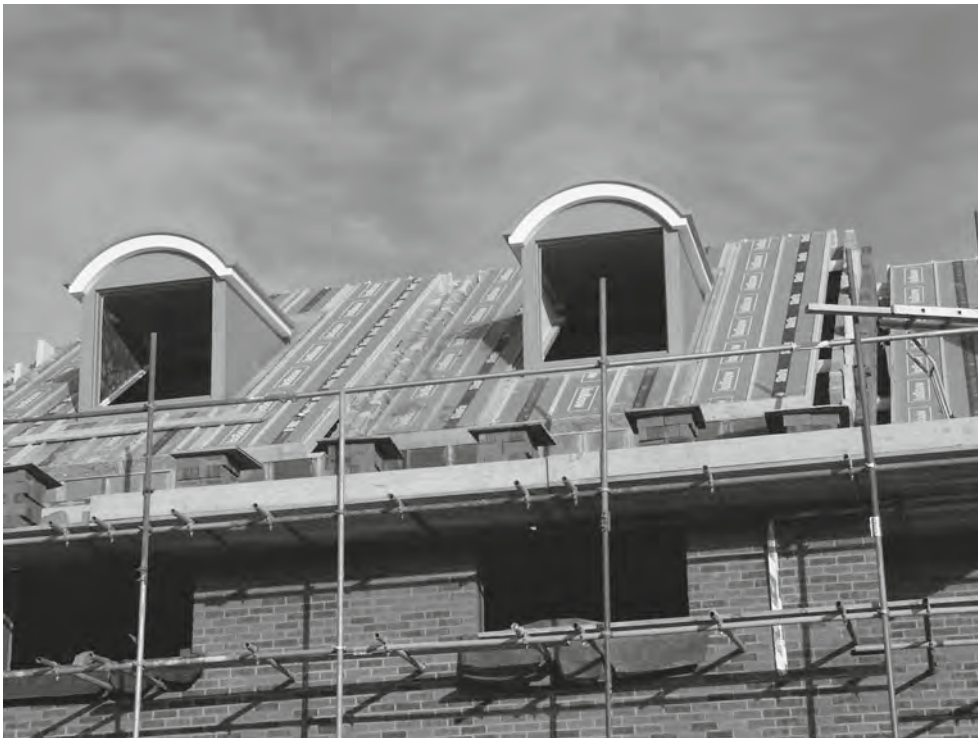
Figure 24.11 Roof elements were used to construct this roof
