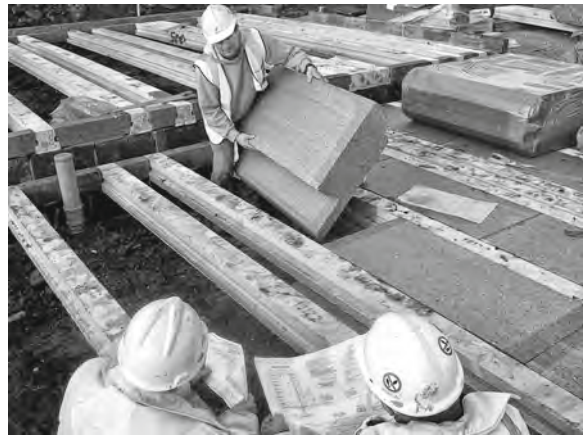
Figure 24.16 Beam and EPS infill
