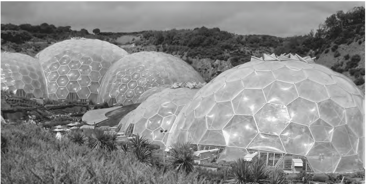
Figure 25.6 Polygonal ETFE cushions – Eden Project, Cornwall. Architects: Grimshaw Architects. Photograph: Arthur Lyons (This image was published in Materials for Architects and Builders , Arthur Lyons, 4th edition, p. 314. Copyright: Butterworth Heinemann, 2010)
