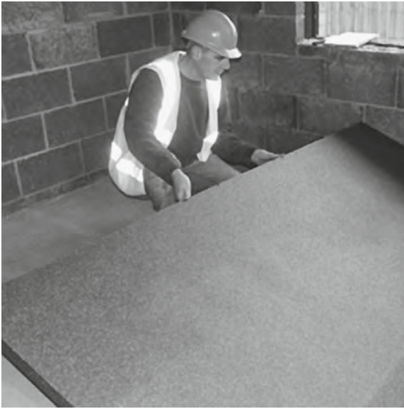
Figure 24.14 EPS used over a concrete slab
