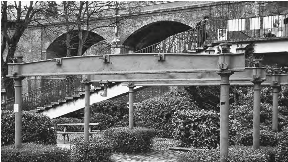
Figure 5.1 A bay of cast iron columns and beams from a textile mill, re-erected on campus at Manchester University
