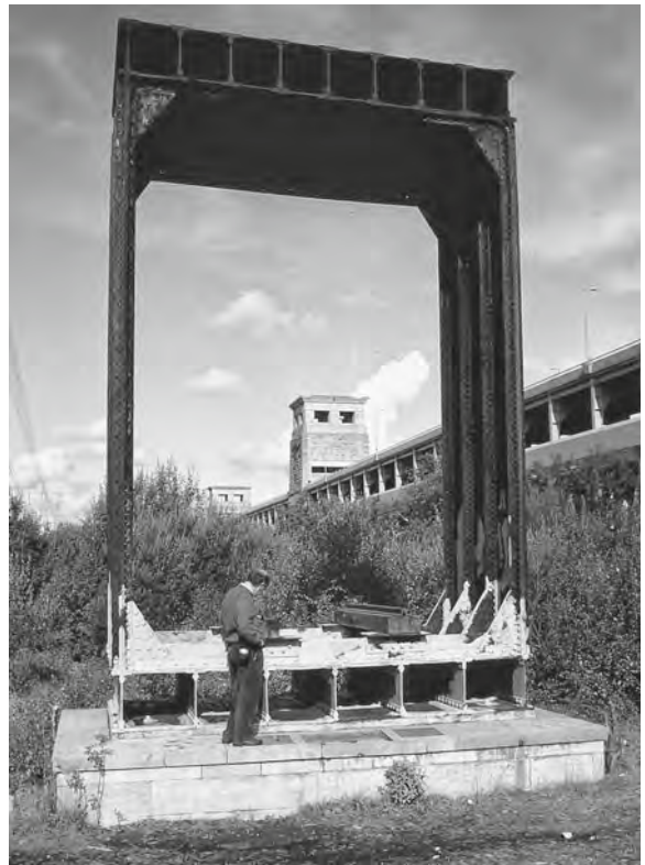
Figure 6.6 The surviving section of the huge tubular girders of the 1850 Britannia Railway Bridge over the Menai Strait, re-erected close to the replacement steel arch bridge after the tubes were irreparably damaged by fire in 1970
