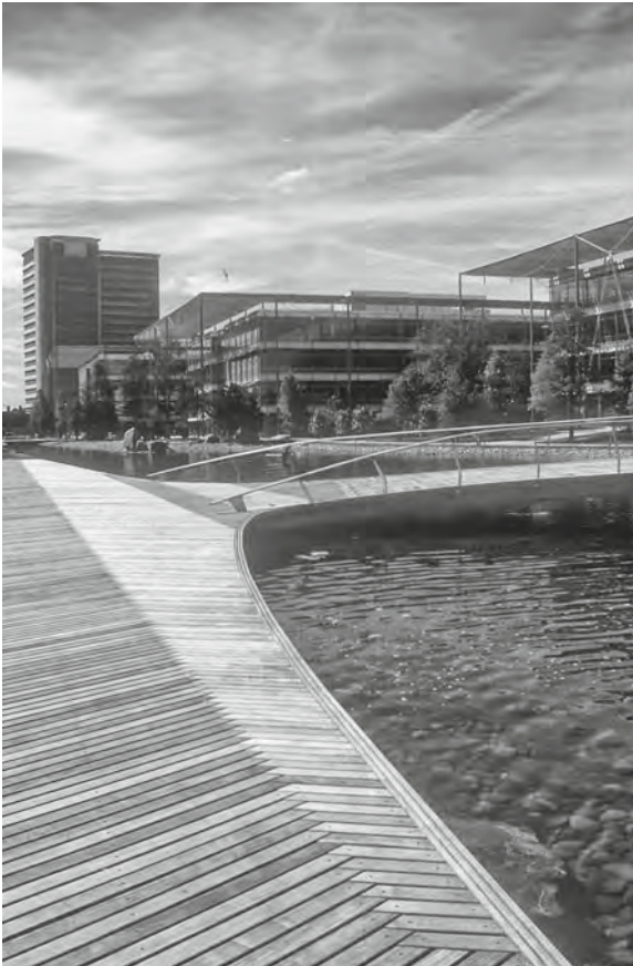
Figure 33.10 The tropical hardwoods are generally strong and durable, making them ideal for decking. The deck at Chiswick Park uses a timber called Vitex that was available with FSC certification (Architect: Richard Rogers Partnership, Engineer: Arup). © Arup
