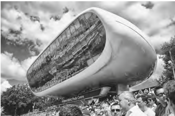
Figure 2.7 The Investec Media Centre at Lord's Cricket Ground, London. Designed in aluminium by Future Systems and fabricated in the Pendennis shipyard
