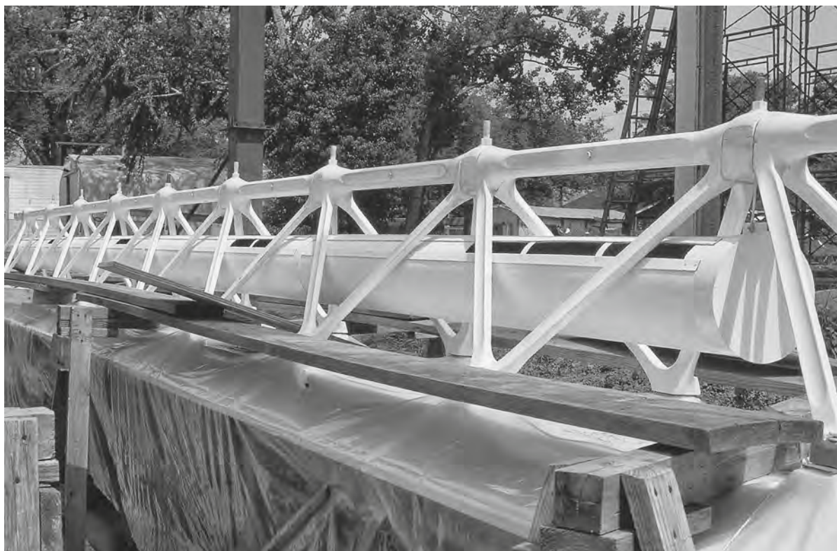
Figure 5.13 Ductile cast iron roof trusses for the Menil Gallery, Houston (courtesy of Arup)
