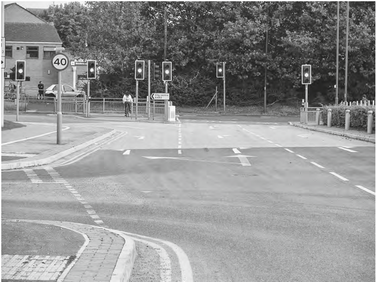
Figure 34.18 Traffic signal approach showing Clause 924 High Friction Surfing
