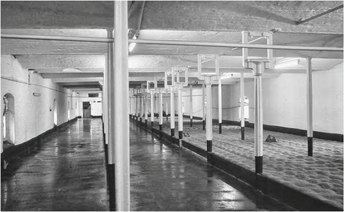
Figure 5.9 Ditherington Mill, Shrewsbury of 1797, the first multi-storey iron-framed building
