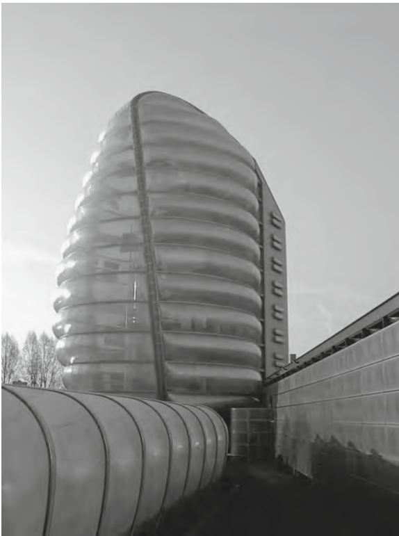
Figure 25.5 Banded ETFE cushions – National Space Centre, Leicester. Architects: Grimshaw Architects. Photograph: Arthur Lyons. (This image was published in Materials for Architects and Builders , Arthur Lyons, 4th edition, p. 315. Copyright: Butterworth Heinemann, 2010)
