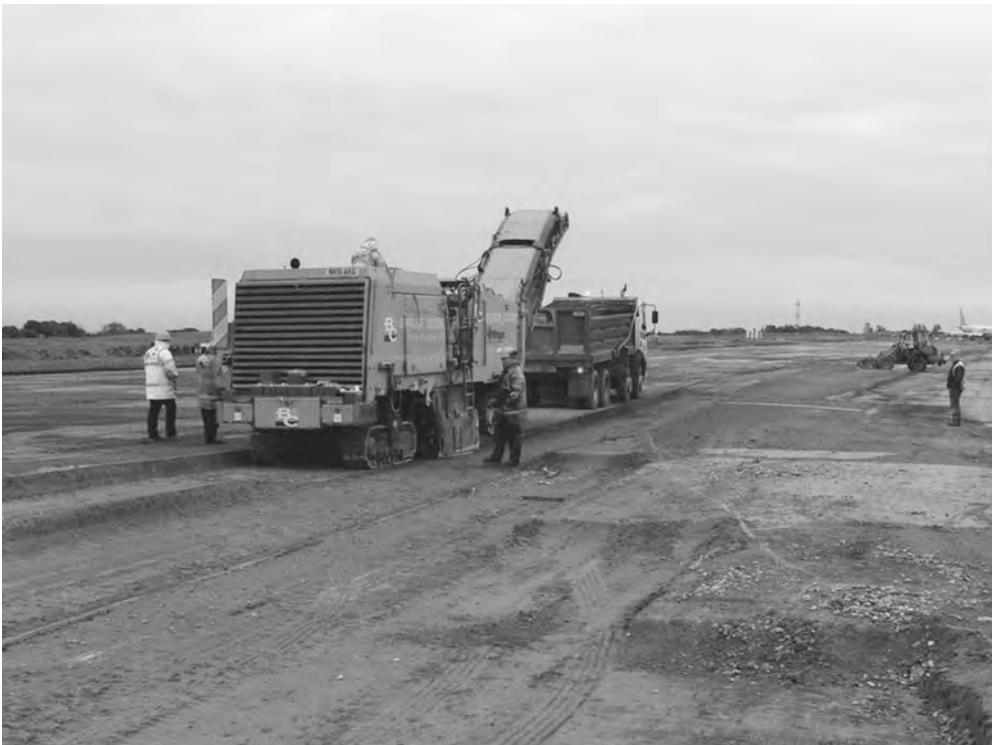
Figure 34.31 Road plane removing a fretted pavement surfacing material
