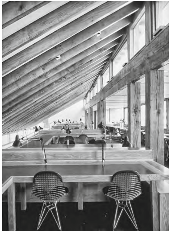
Figure 33.7 At Darwin College, Cambridge, the oak columns were installed green and allowed to season in situ. The fissures are the result of the greater tangential shrinkage (for oak 8%, compared to only 4% radially) (Architect: Dixon Jones, Engineer: Arup). © Arup
