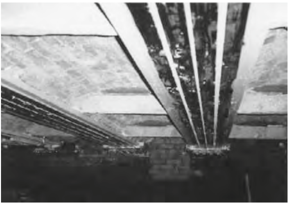
Figure 31.2 Hythe Bridge strengthening, Oxford, using prestressed CFRP plates (courtesy Mouchel Parkman) (Continued)
