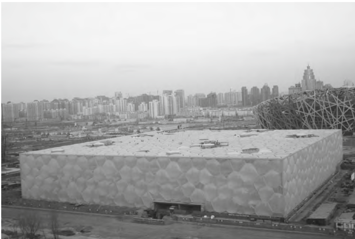
Figure 36.4 The Water Cube, Beijing
