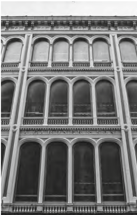
Figure 5.10 The façade of the 1855–6 Gardner's warehouse in Glasgow, with cast iron panels forming both the structure and the envelope
