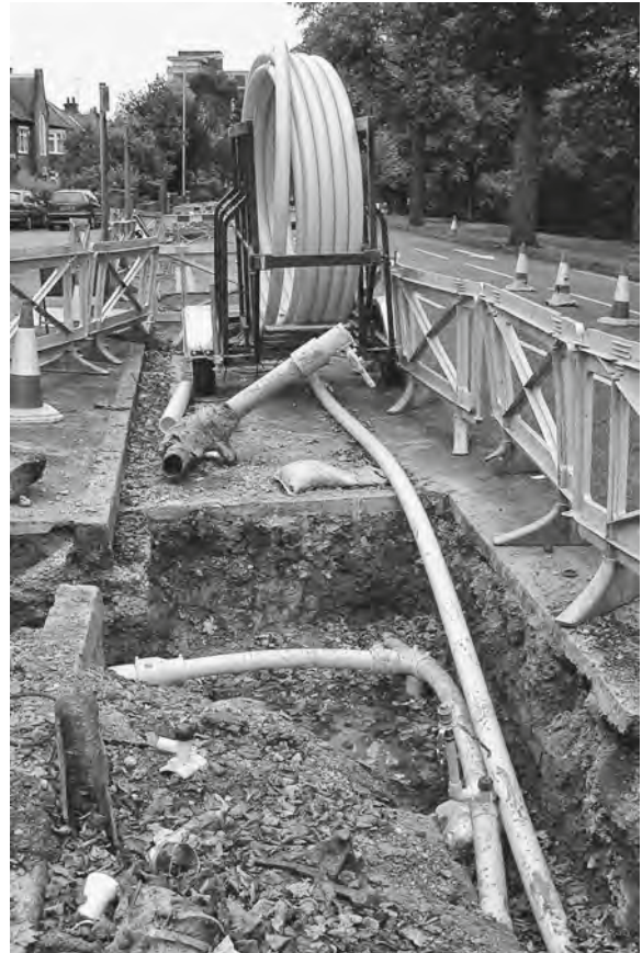
Figure 22.5 Slip-lining of polyethylene gas pipe into old main
