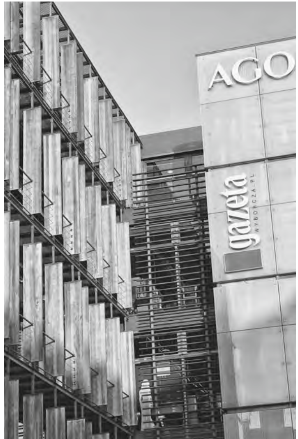
Figure 33.11 Western red cedar is a durable timber often used for cladding, and seen here at the new headquarters for a prominent Polish newspaper (Architect: JEMS, Engineer: Arup). © Arup
