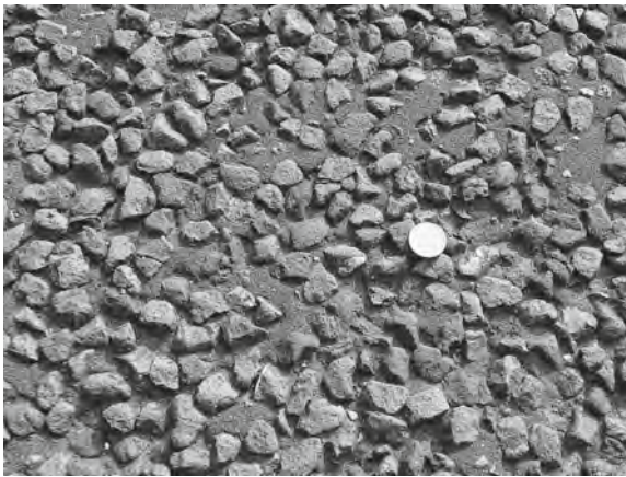
Figure 34.11 20mm Chipped HRA to a high speed county road
