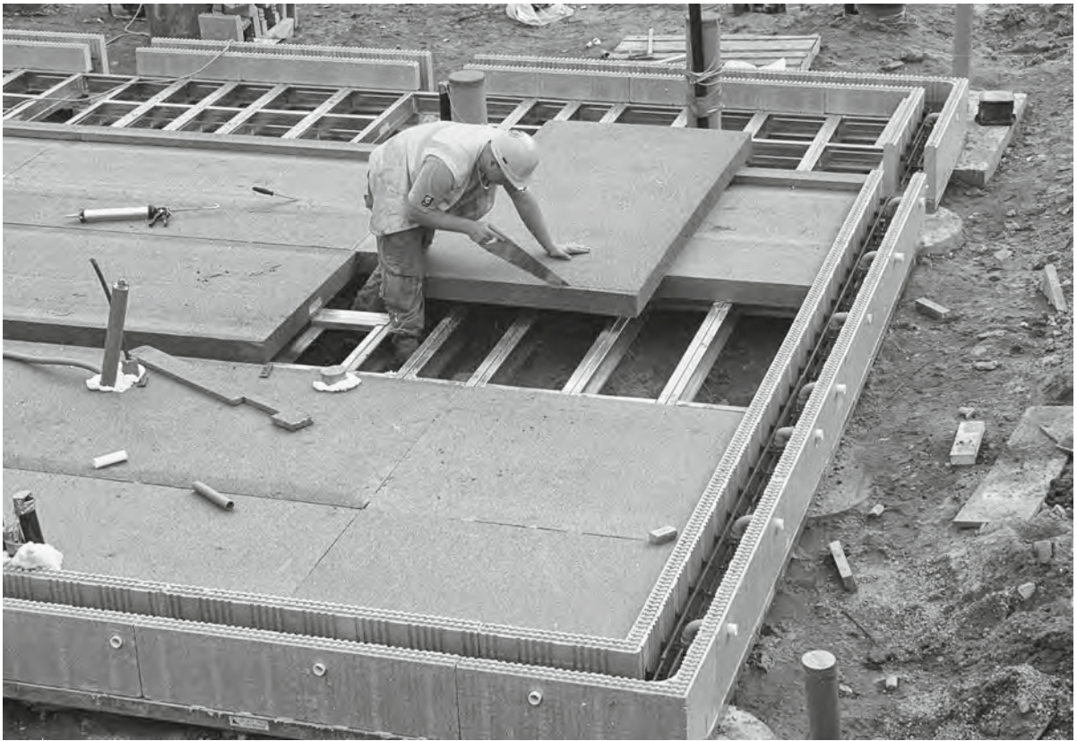
Figure 24.17 EPS spanning suspended beams
