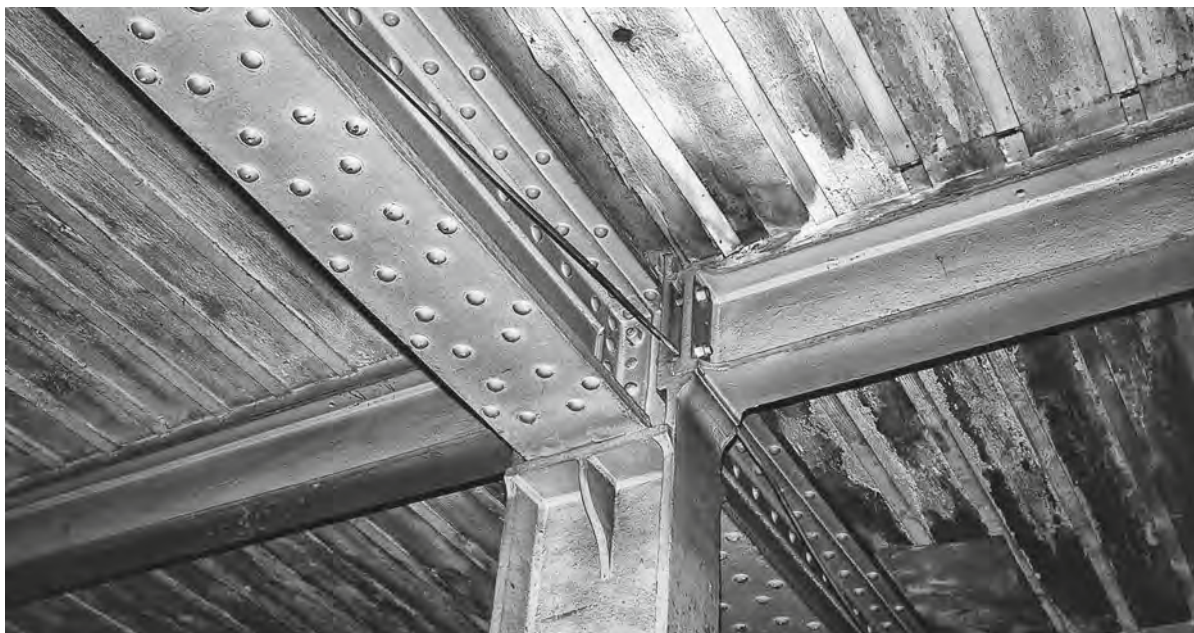
Figure 5.12 Column-beam junction in the Boat Store at Sheerness Dockyard
