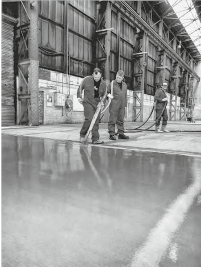
Figure 17.2 A pump-applied, self-levelling mortar, specifically developed for the rapid resurfacing and levelling of existing concrete floors, providing a hard, smooth, flat surface, resilient enough to accept the heavy wheeled traffic typical of industrial workshops and warehouses. This formulation chemically binds the mix water without evaporation, allowing further work, including the application of water-based systems such as epoxy paint coatings, in as little as 6 hours. Reproduced with kind permission of Ardex (UK) Ltd
