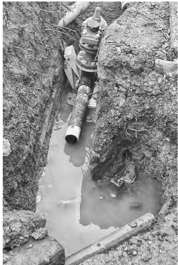
Figure 22.8 Peelable water pipe jointing
