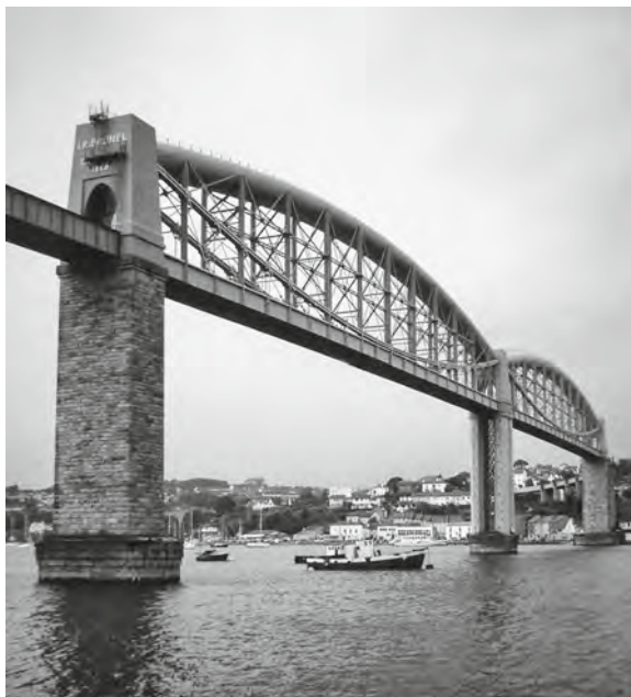
Figure 6.9 The 1859 Royal Albert Bridge across the River Tamar west of Plymouth; two self-anchored ‘suspension arches’, each spanning 139 m, still carrying mainline rail traffic to and from Cornwall
