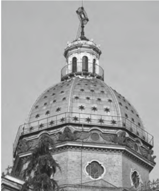
Figure 2.1 The aluminium-clad dome of the San Gioacchino Church in Rome, in service since 1897
