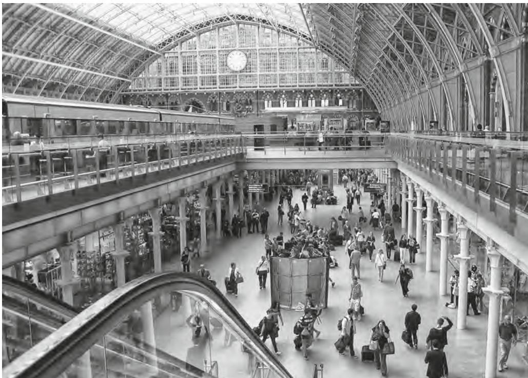
Figure 6.8 The 73 m span roof of St Pancras Station, completed in 1868 and recently restored to accommodate London's international passenger rail terminal
