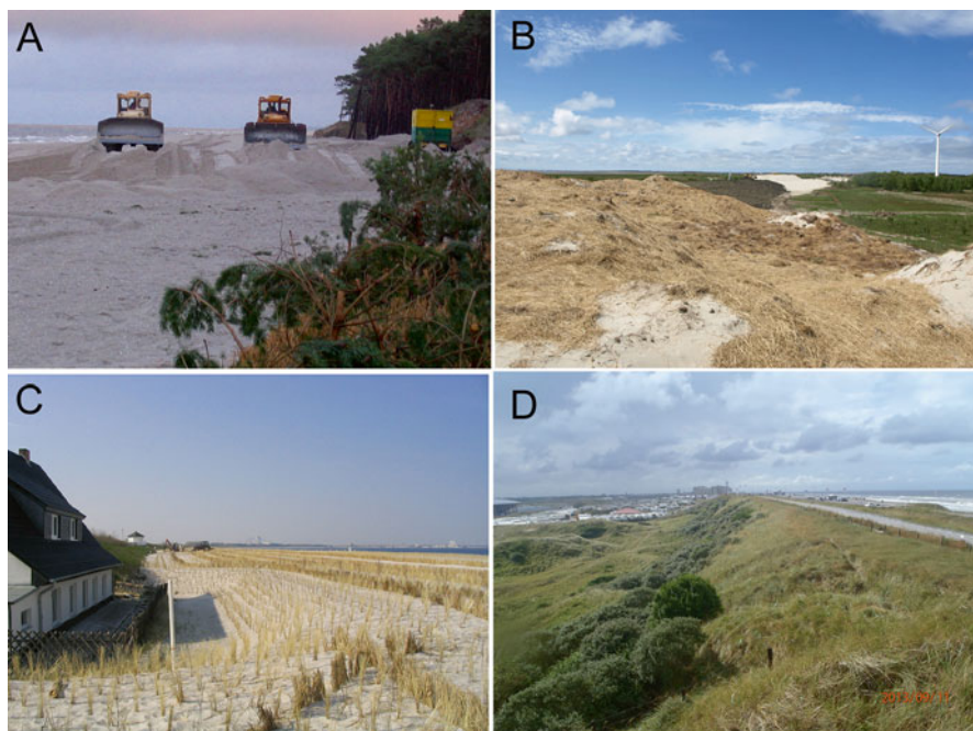
Fig. 14.21 Dunes and beach nourishment phases. (a) Beach nourishment and dune rebuild, Mrzezyno, Poland. (b) Artificial dune ridge built for flood protection, scattered reeds to support the soil development, Spiekeroog Island, Germany. (c) Completely rebuilt foredune, Hohe Düne near Warnemünde, Germany. (d) Built already mature dyke, pretending to be foredune, Zandvoort, Netherlands
