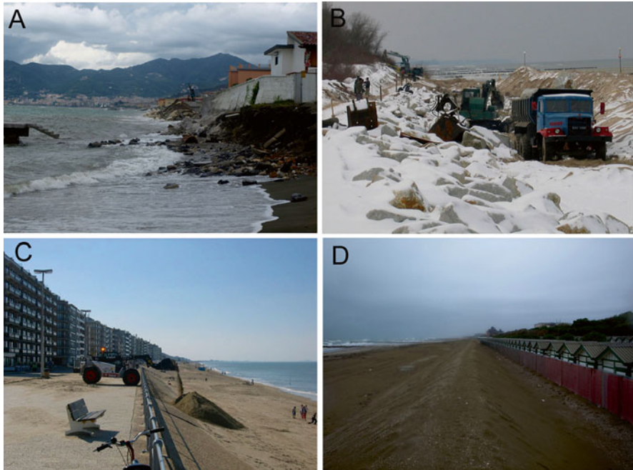
Fig. 14.16 Coastal dune erosion issues. (a) Coastal erosion, dune destroyed by the sea, Salerno Italy. (b) Covering eroded dunes by rock blocks, near Kolobrzeg, Poland. (c) Instead dunes concrete dyke with promenade, the removal of naturally accumulated sand disturbing walkers, Koksijde, Belgium. (d) Artificial sand dyke resembling dune, Lido on the Venice Spit, Italy
