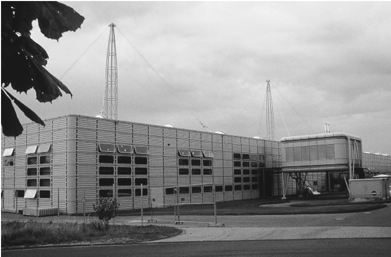
The panels at Iguaz can be quickly switched from solid to glass, from walls to doors, making it easy to adapt the building to various uses with minimal time, cost, or disruption.
