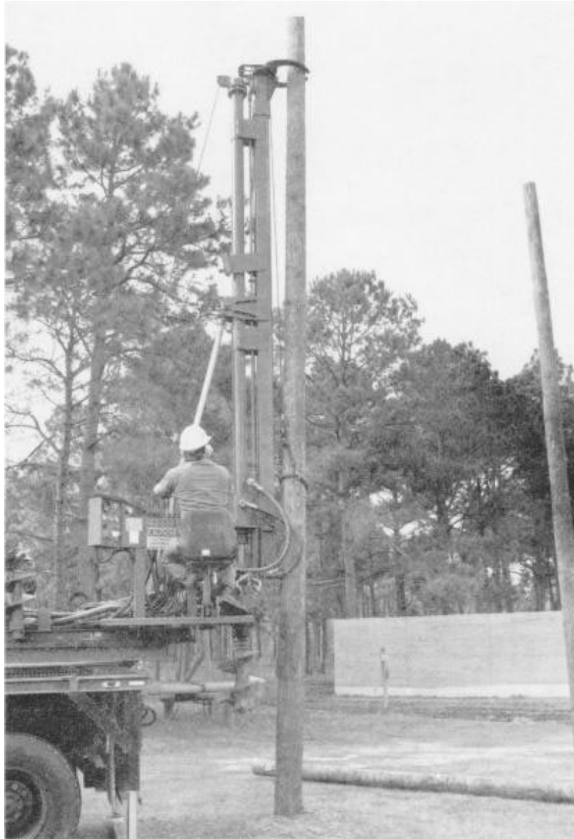
Figure 4-52.—Auger truck setting a pole.
