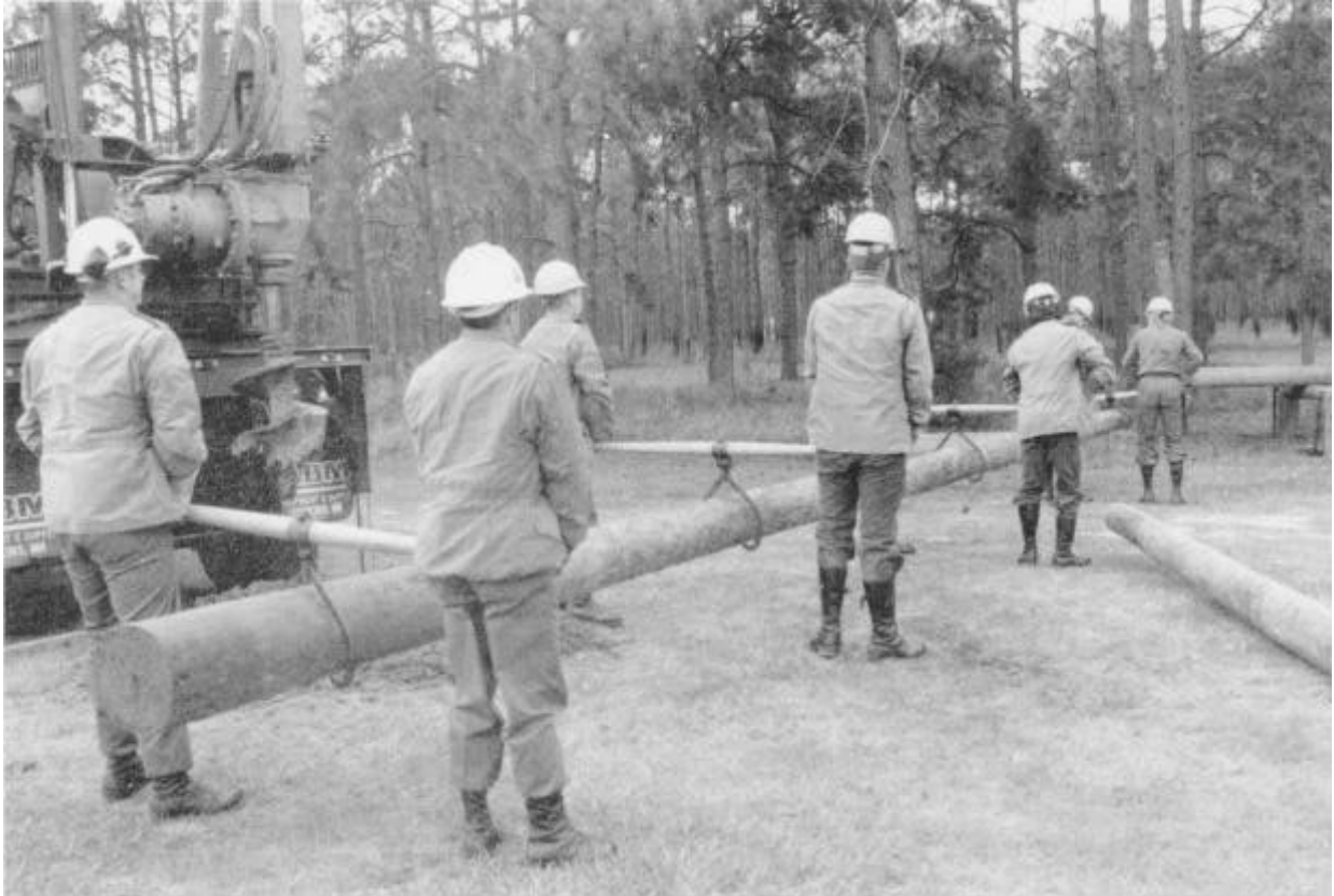
Figure 4-54.—Manually positioning a pole.
