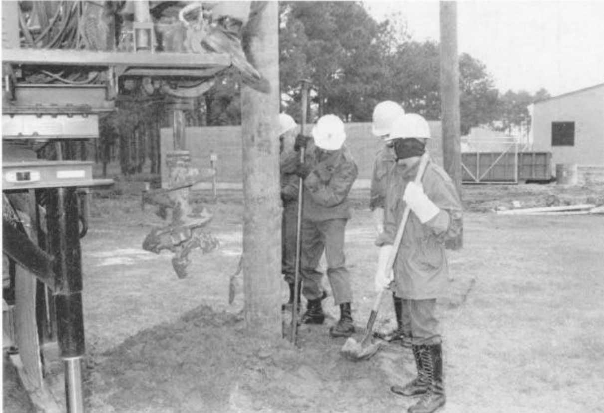
Figure 4-58.—Tamping and backfilling erected pole.
