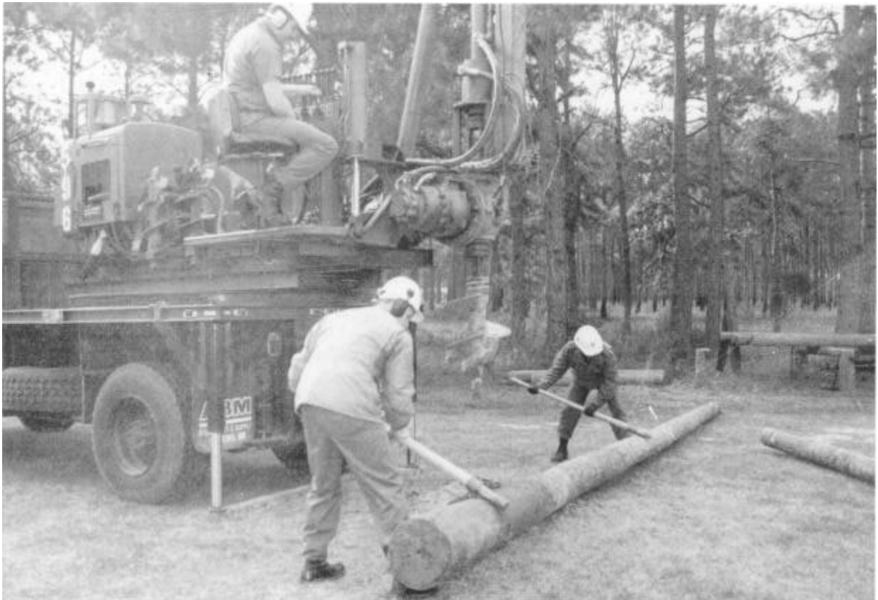
Figure 4-51.—Pole positioning before being set.
