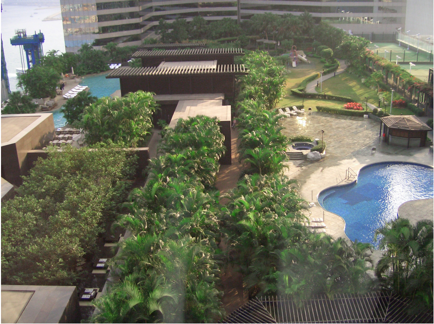
Fig. 8 Rooftop gardens increase biodiversity in cities while at the same time reduce heat transfer to the interior of buildings
