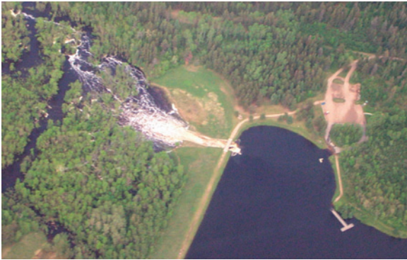
FIGURE 4-4 Flood spillway in use on Hayes Lake, Roseau River, United States. (Source: US National Oceanographic and Atmospheric Administration, 2002.)
