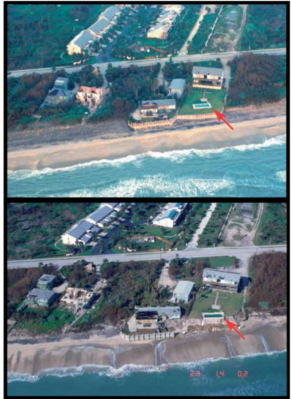
FIGURE 4-3 Example of a seawall failure following Hurricane Jeanne in 2004, Melbourne Shores, Florida. (Source: United States Geological Survey, 2004.)
