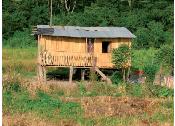
FIGURE 4-1 House built on stilts above annual flood levels in Guayas Province, Ecuador. (Source: Author.)
