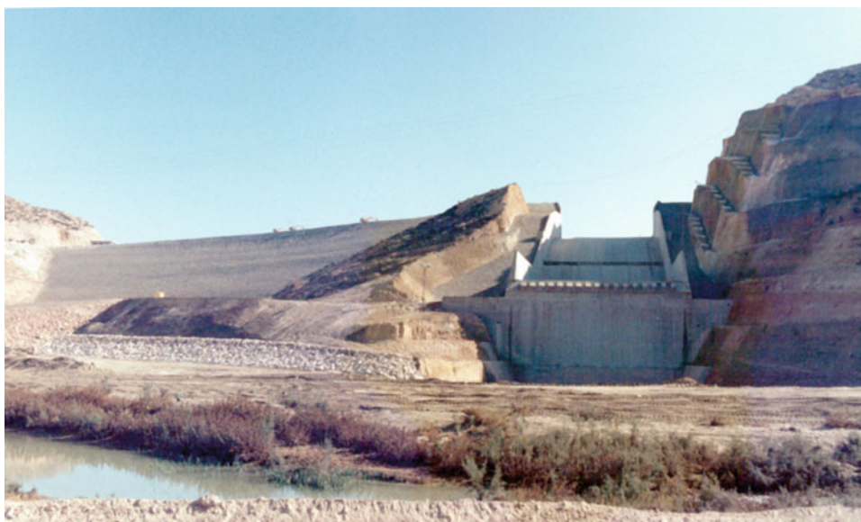
Fig. 1.1 Gargar dam (Algeria). Spillway
