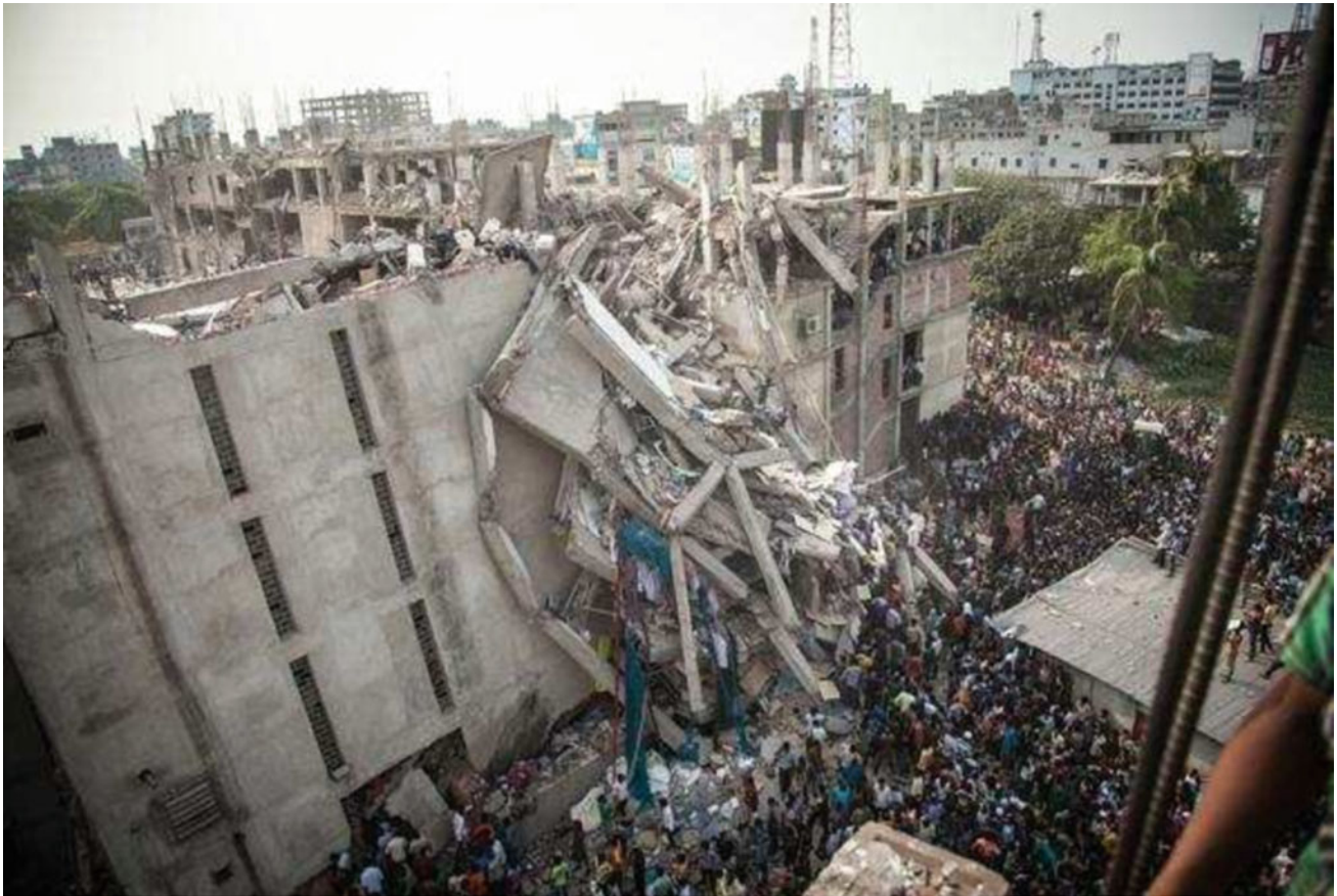
Fig. 6.3 Example of building collapse (Source The Economist)
