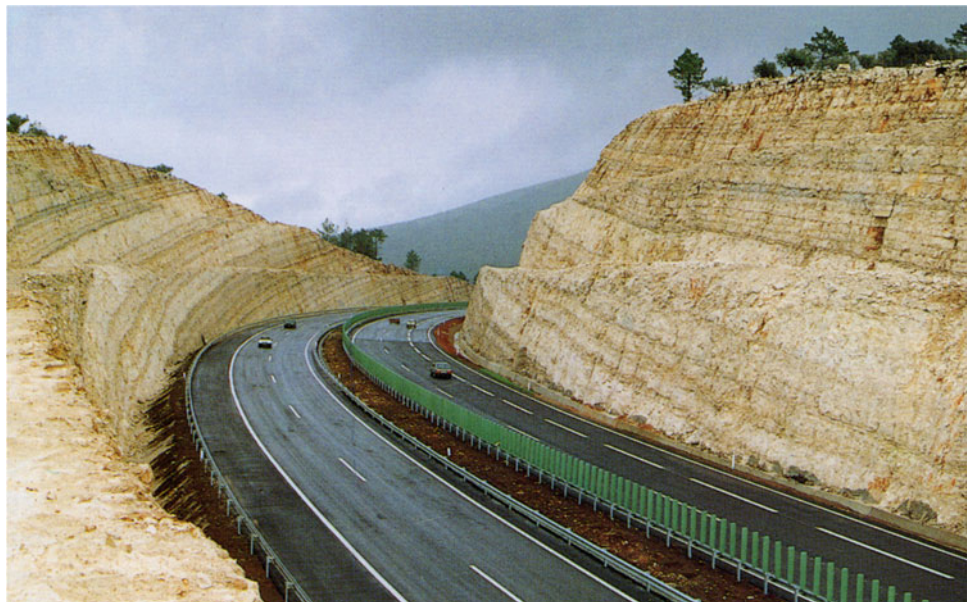
Fig. 1.3 Motorway A1. Solution open excavation
