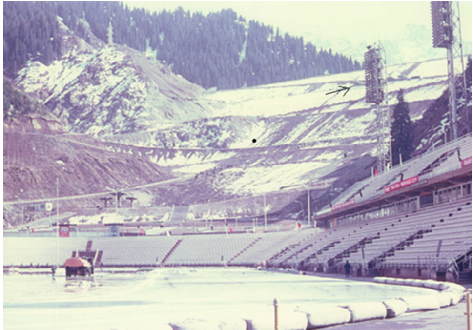
Fig. 50.1 Medeo dam and skating ring Medeo. 1973 dam level shown by arrow/Photo by V.S. Shibakova, April 1977
