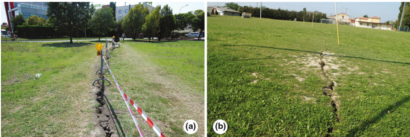
Fig. 19.3 a Ground crack noticed in mid-August 2013 at the outskirts of Ferrara, b ground crack formed by the 20th May 2012 M_L 5.9 quake
