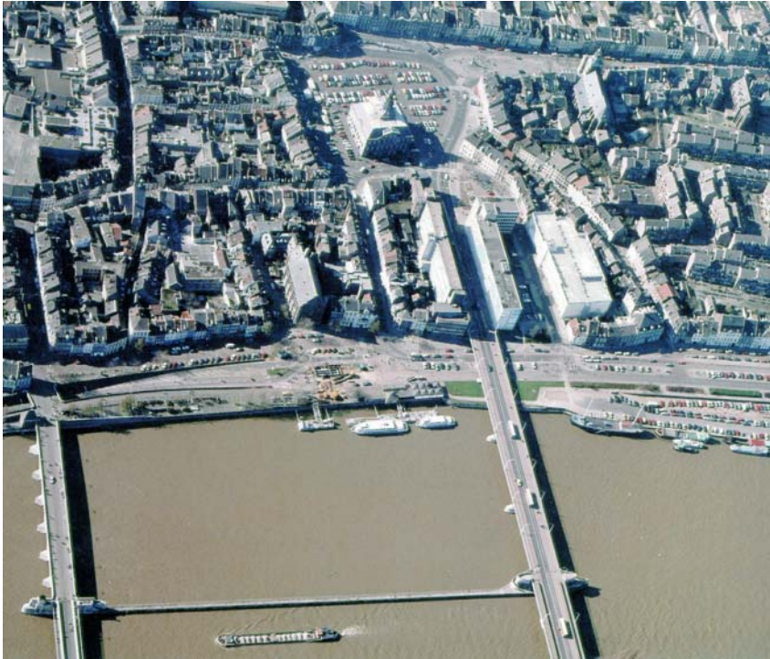
Fig. 1. River Meuse, Maastricht. Bird view on the western Meuse boulevard (situation before construction of the cut-and-cover tunnel). The Wilhelmina Bridge is located north (right on the picture), the St.-Servaas Bridge is located south (left).
