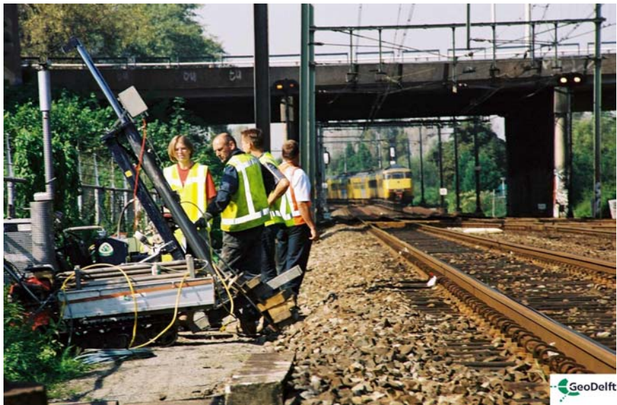
Fig. 2. Electrical density test below railway.
