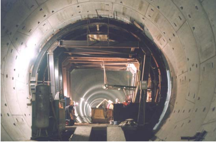
Fig. 3. Photo of prestressed steel rings at cross connection 2.
