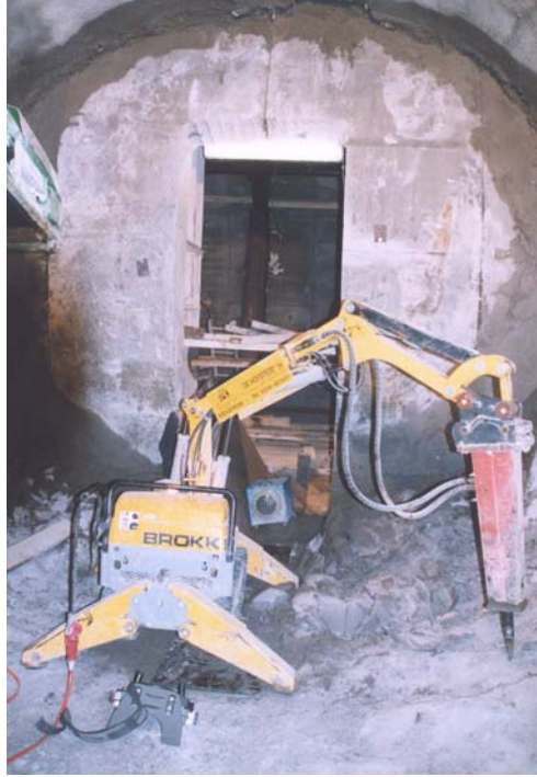
Fig. 7. Photo of the excavated cross connection 2.
