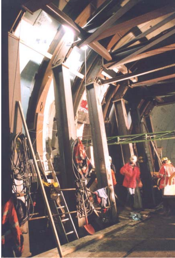
Fig. 8. Detail photo of the prestressed steel rings at cross connection 2.
