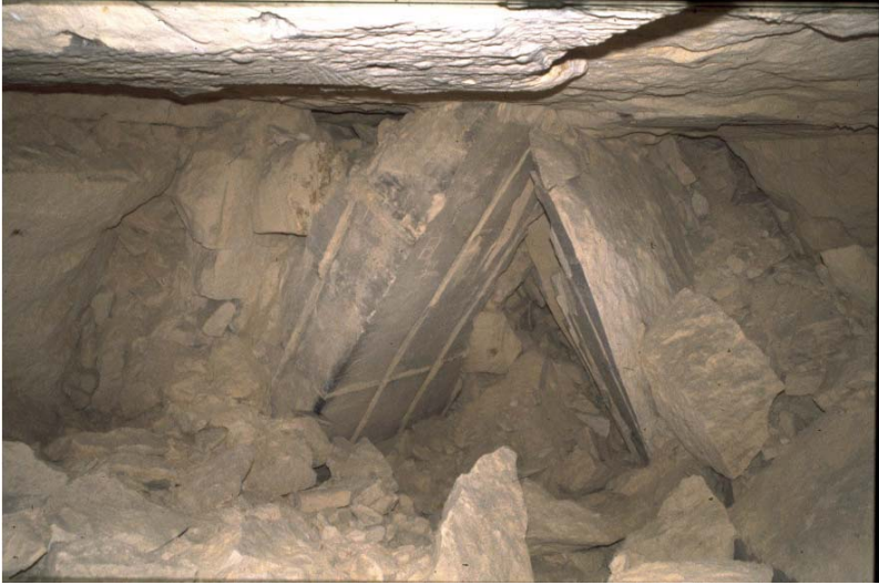
Fig. 2.4. Inside the collapse area of the Muizenberg near Kanne. Segments of opposite pillar walls moved into the gallery partly by rotation, and were crushed by the rapidly descending overburden.
