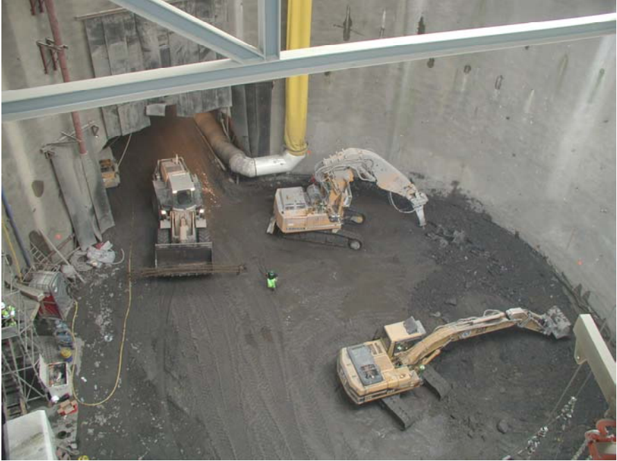
Fig. 7. Intermediate temporary construction shaft.
