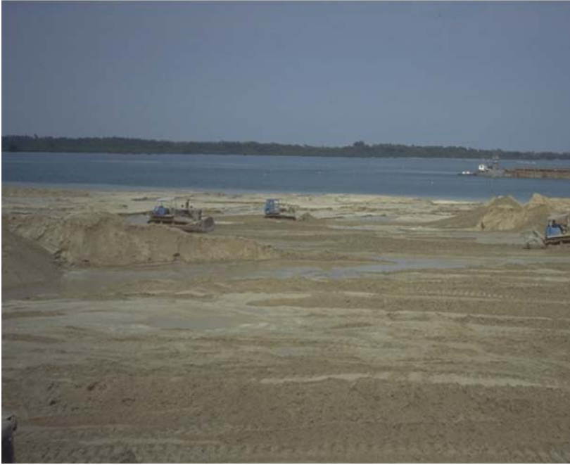
Fig. 2. Reclamation work at Singapore.
