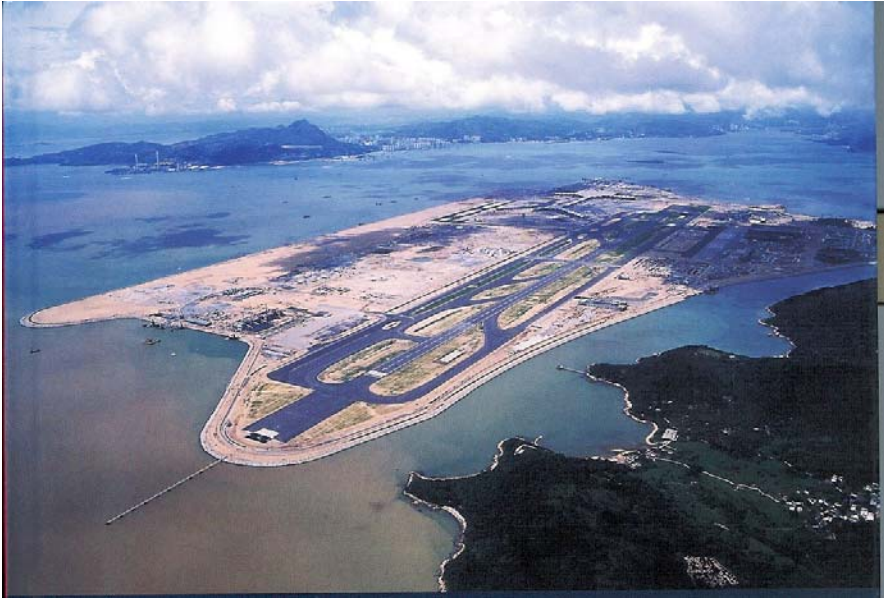
Fig. 1. The New Hong Kong International Airport under construction.
