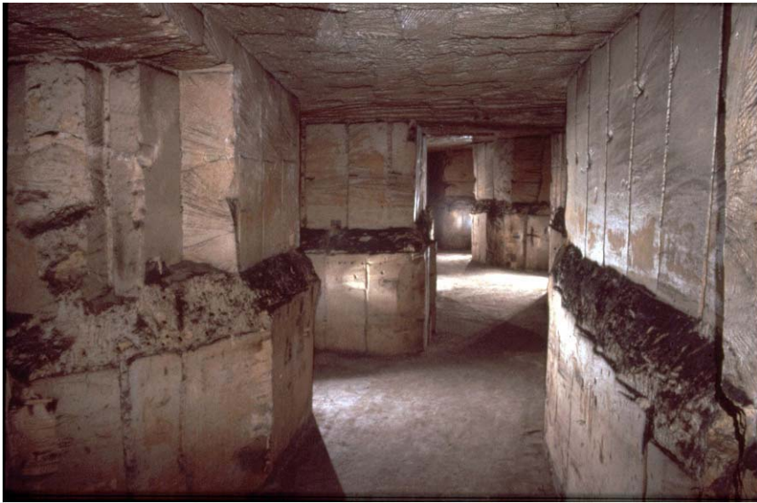
Fig. 1.2. The Heidegroeve near Valkenburg before the collapse of 1988. Two mining levels can be distinguished separated by a hardground. The total pillar height is 4.6 m (Courtesy of J Silvertant).
