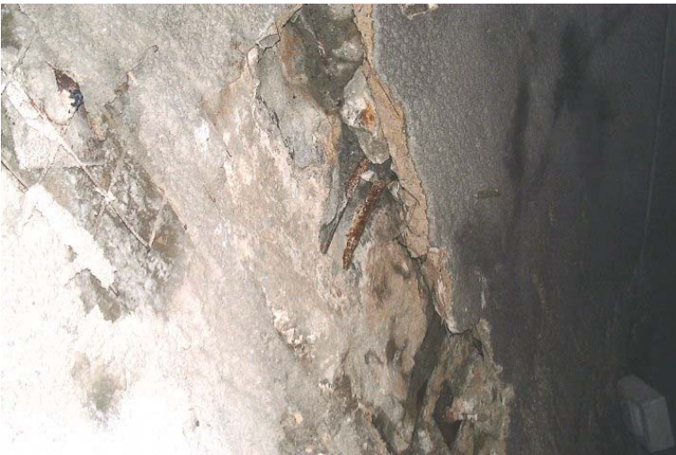
Fig. 2. Detail of the support fractured in the north crown side in the top heading advance section.
