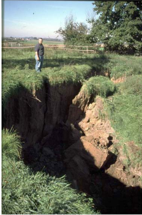
Fig. 2.7. Severe subsidence as a result of the large-scale roof collapse near Zussen, with faults of some m width and up to 8 m vertical offset.
