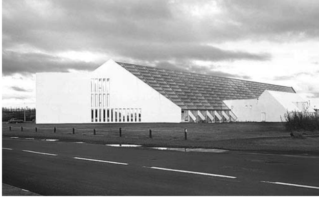
Figure 2. Modern school building at Selfoss in South Iceland
