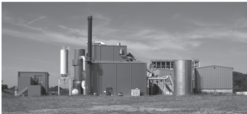
Figure 3.16 An example of a bubbling fluidised bed cogeneration installation with an electrical output of 7.6 and 14 MW heat output (courtesy of Valmet, Finland)
