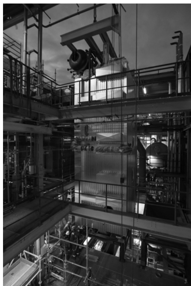
Figure 5.1 The insertion of the heat recovery steam generator in a sewage sludge plant (photograph by www.voog.nl and courtesy of NEM)
