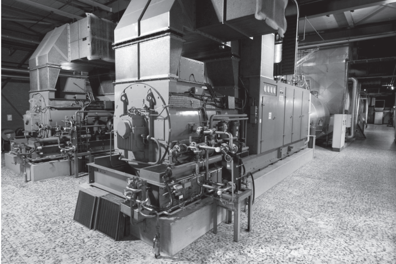
Figure 3.2 A cogeneration installation based on four 3.6 MW aero-derivative gas turbines in a paper factory (courtesy of CENTRAX)
