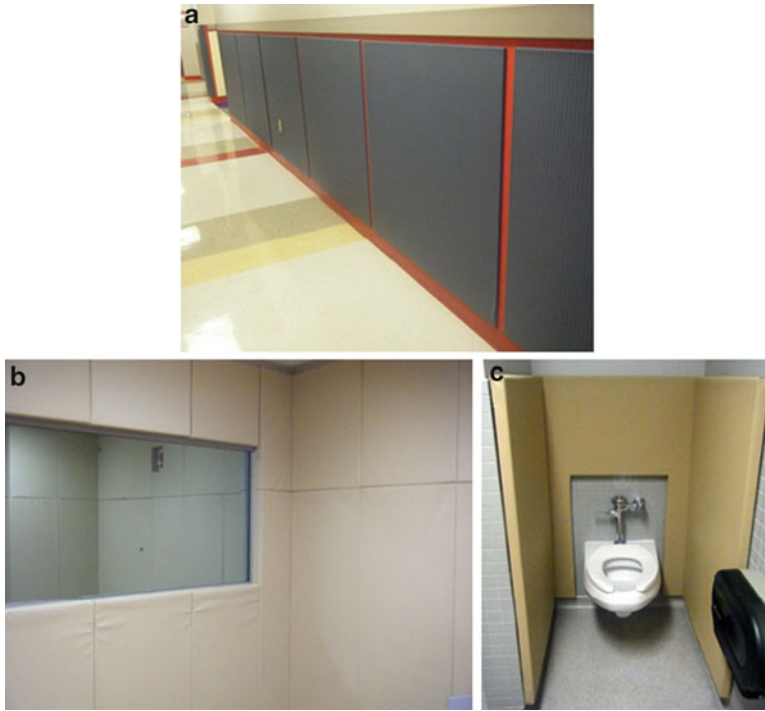
Fig. 6.1 Acrovyn® wall panels covering the wall in a hallway are shown in picture (a). A room with a padded floor and walls with a one-way mirror for observation is shown in picture (b). A padded commode is shown in picture (c)
