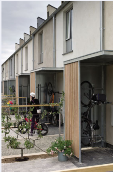
Figure 2.56 Swindon: bike shed. Reproduced by permission of Glenn Howells Architects.
