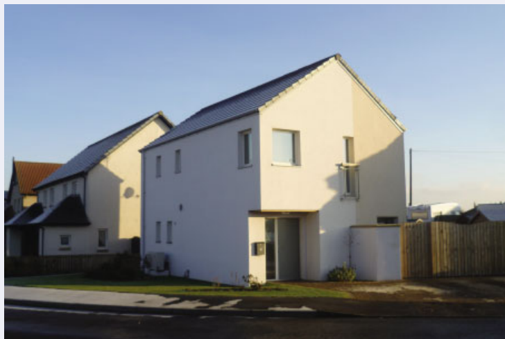
Figure 2.59 Pittenweem: north facing
