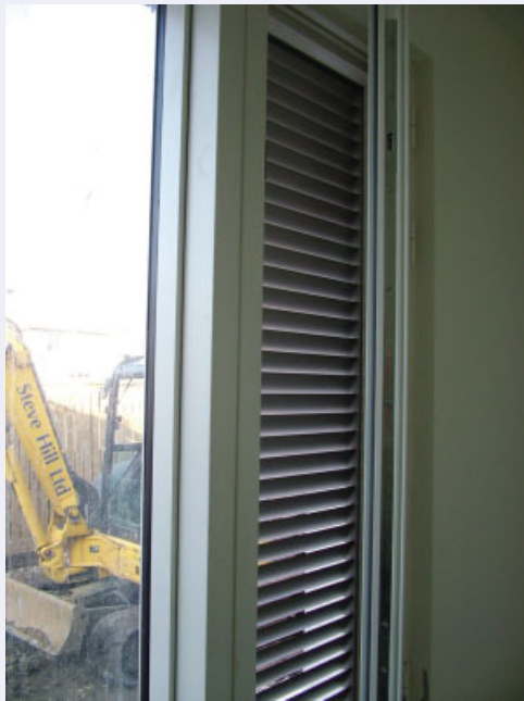
Figure 2.55 Swindon: window detail showing open louvres
