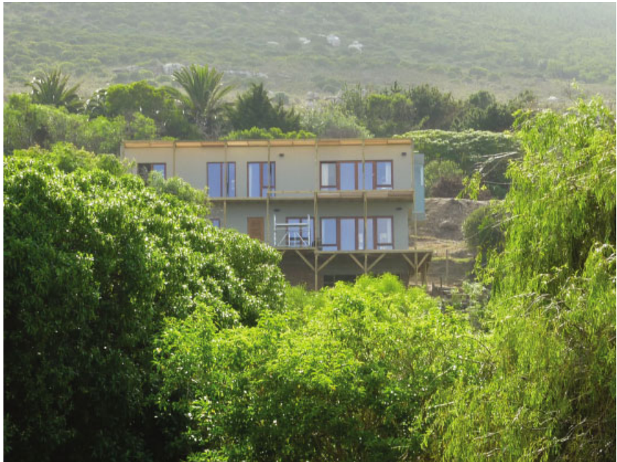
Figure 7.1 Hemp house in Nordhoek, South Africa (front). Reproduced by permission of Hemporium, South Africa.
