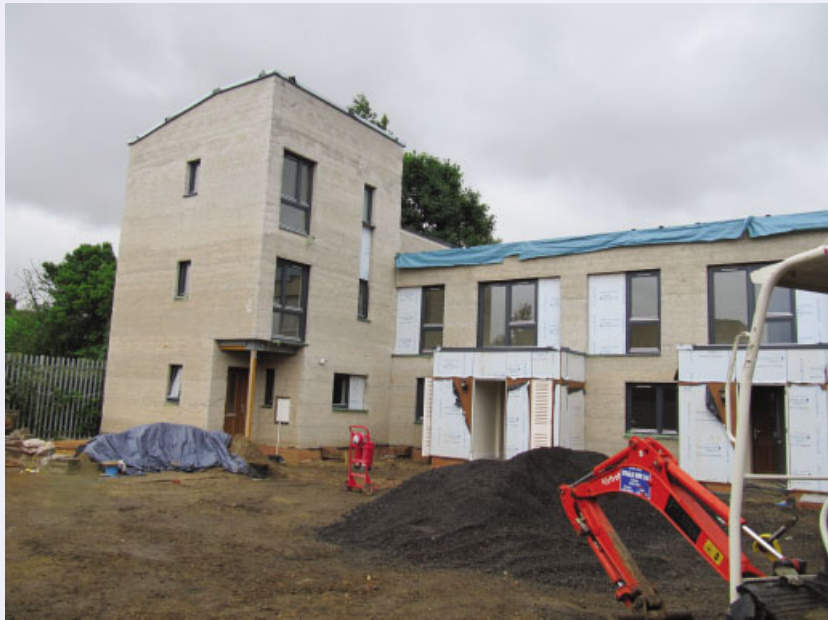
Figure 2.21 Callowlands: different coloured bands on the hempcrete show variation in drying out. Reproduced by permission of Luke Brooker MSc, The Airey Miller Partnership.
