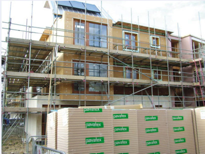
Figure 2.39 Letchworth: Pavatex Wood fibre construction of three-storey units
