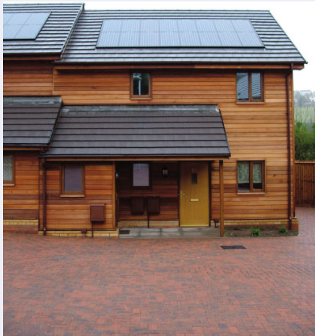
Figure 2.3 Abertridwr: elevation showing PV cells on roof
