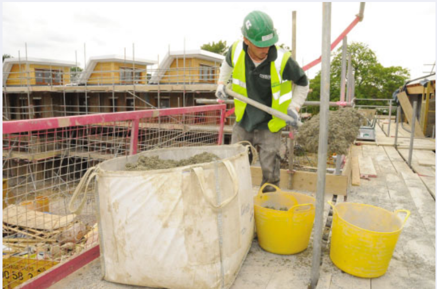
Figure 2.41 Letchworth: manual placing of hempcrete on site
