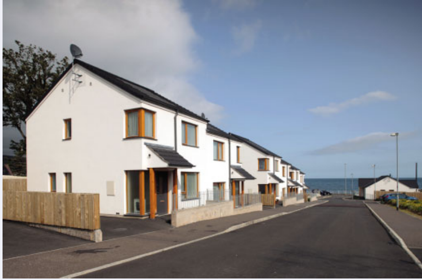
Figure 2.11 Carnlough: finished houses
