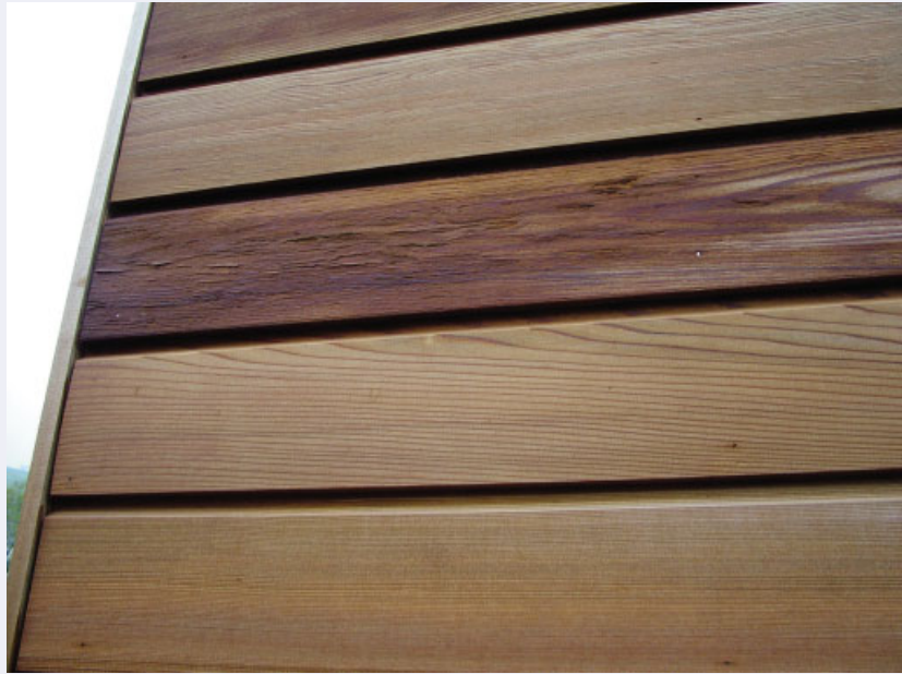
Figure 2.4 Abertridwr: cedar cladding detail
