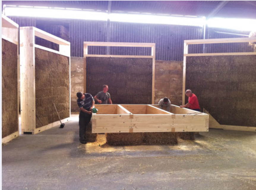
Figure 2.35 Modcell strawbale 'flying factory' as will be used on the LILAC project. Reproduced by permission of ModCell.
