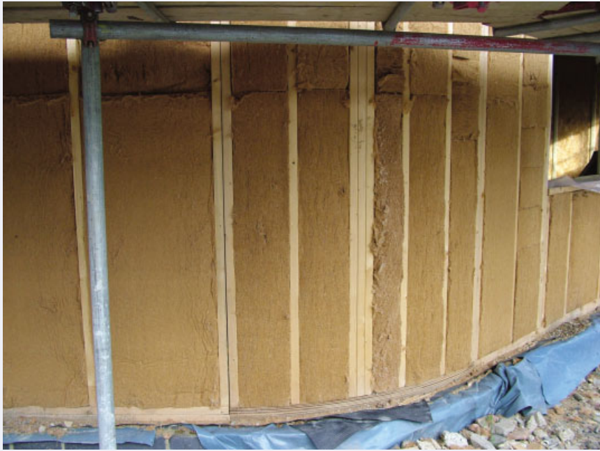
Figure 2.38 Letchworth: detail of wood fibre construction
