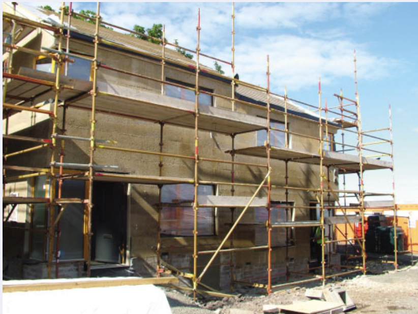
Figure 2.8 Carnlough: hempcrete before render applied
