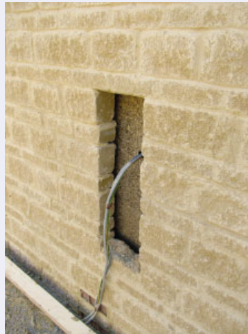
Figure 2.14 Blackditch: wall detail showing cavity and stone facing
