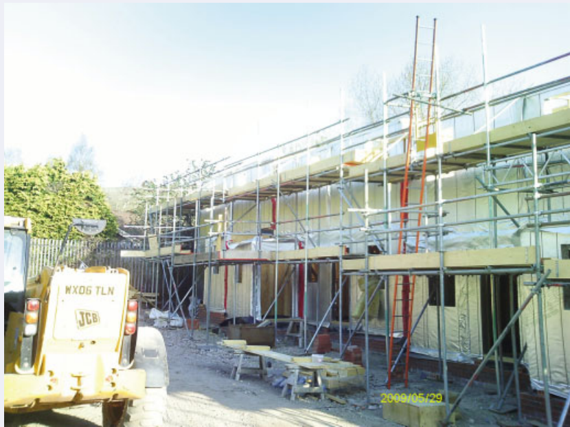
Figure 2.5 Abertridwr: under construction. Reproduced by permission of Green Hill Construction Ltd.
