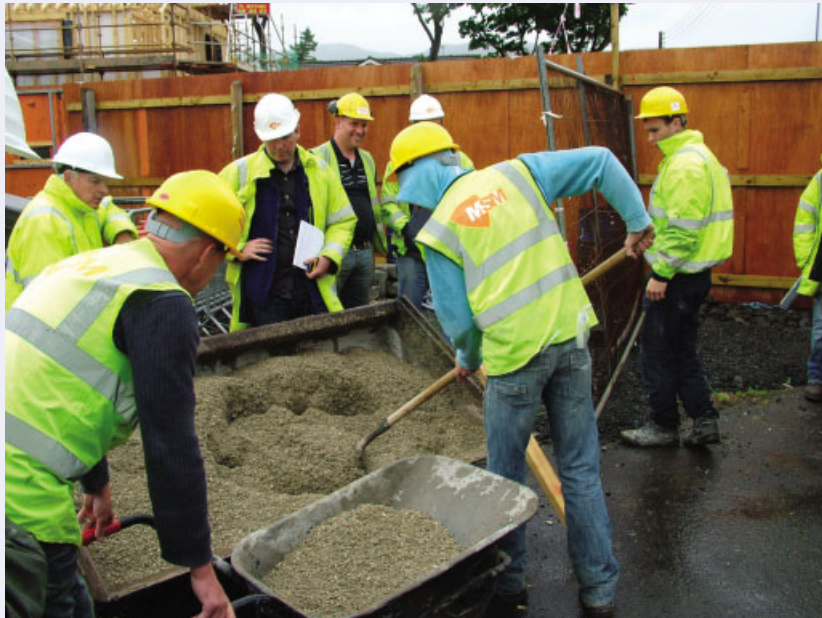
Figure 2.7 Carnlough: contractors staff training on using hempcrete
