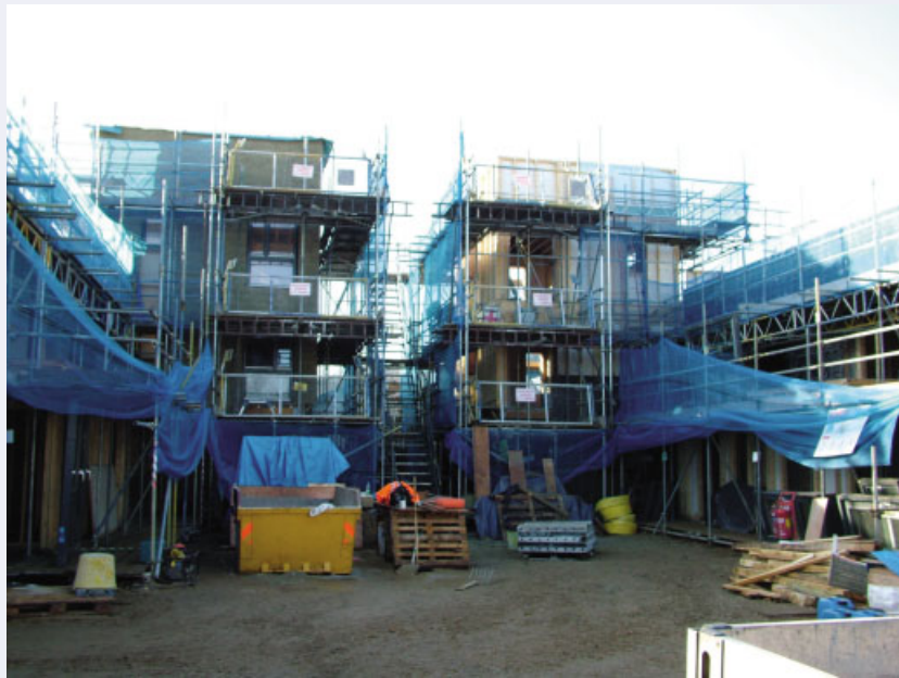
Figure 2.18 Callowlands: three-storey block under construction
