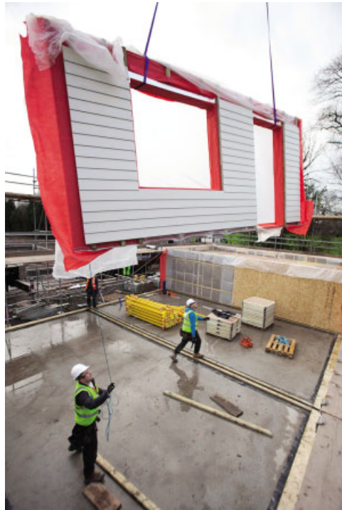
Figure 7.11 LoCaL house being erected on site. Reproduced by permission of The Accord Group.
