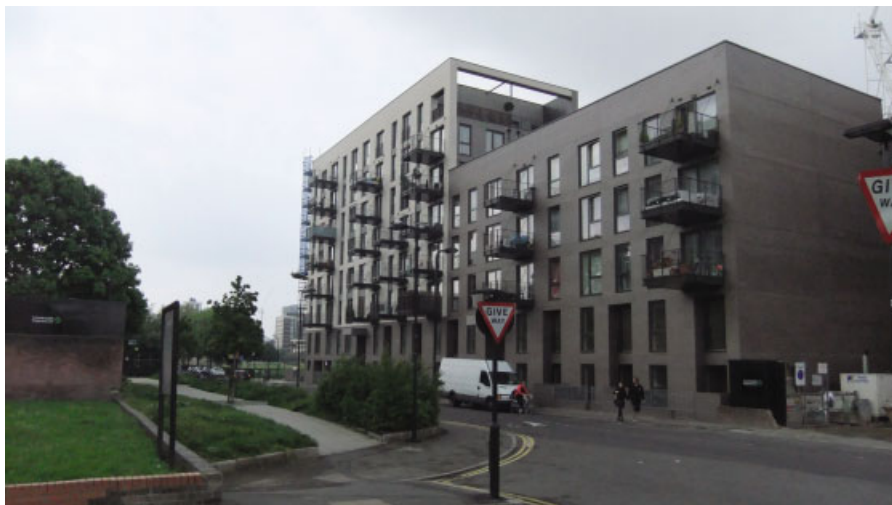
Figure 1.4 Bridport House, Hackney, solid timber panel multi-storey construction
