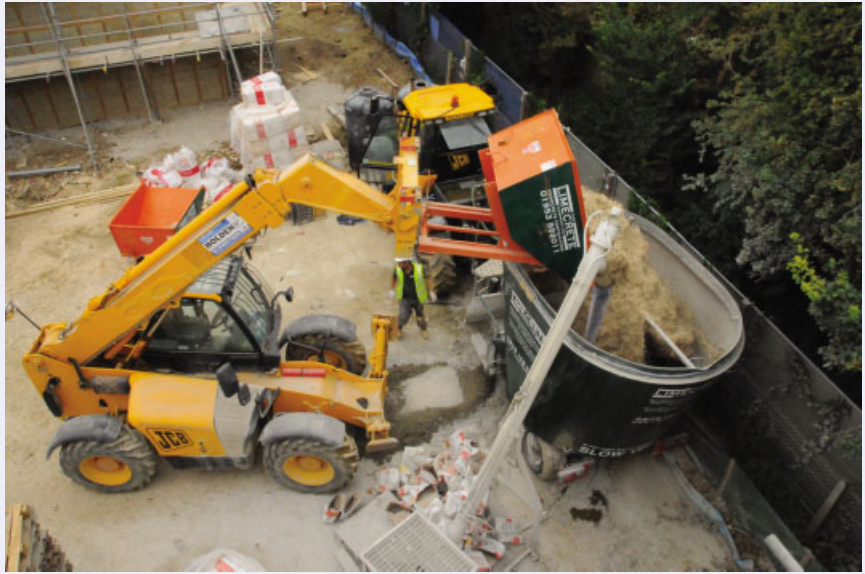
Figure 2.40 Letchworth: the Limecrete Company mixing hempcrete on site. Reproduced by permission of The Limecrete Company Ltd.
