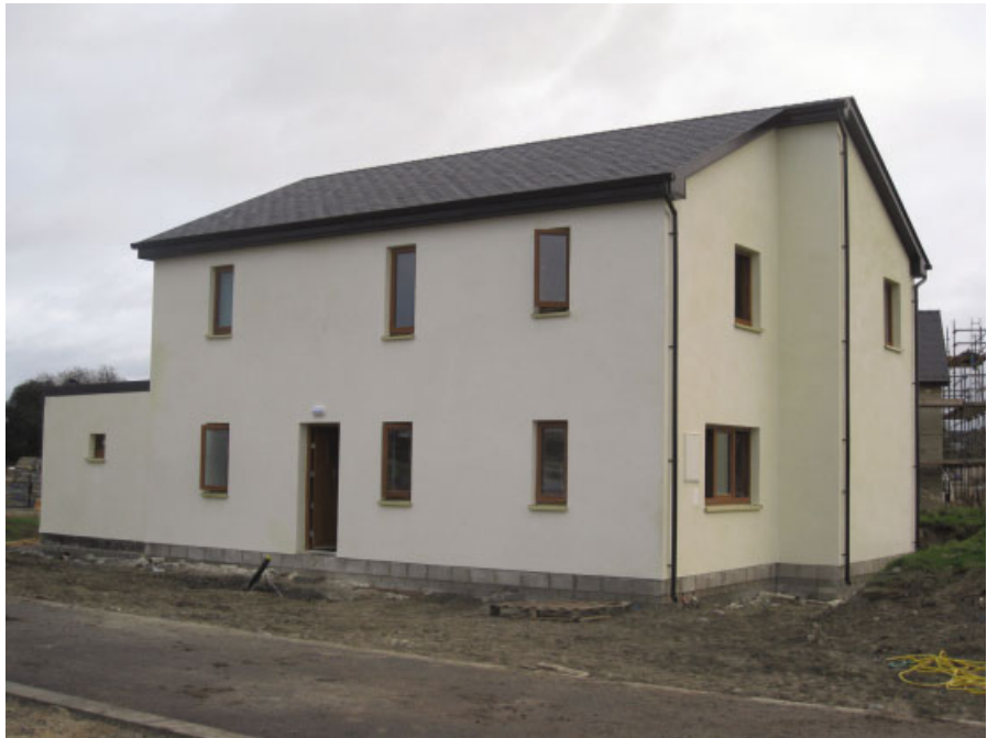
Figure 7.3 Cloughjordan hempcrete house designed by Niall Leahy. Reproduced by permission of Brendan Power, Acorn Energy.
