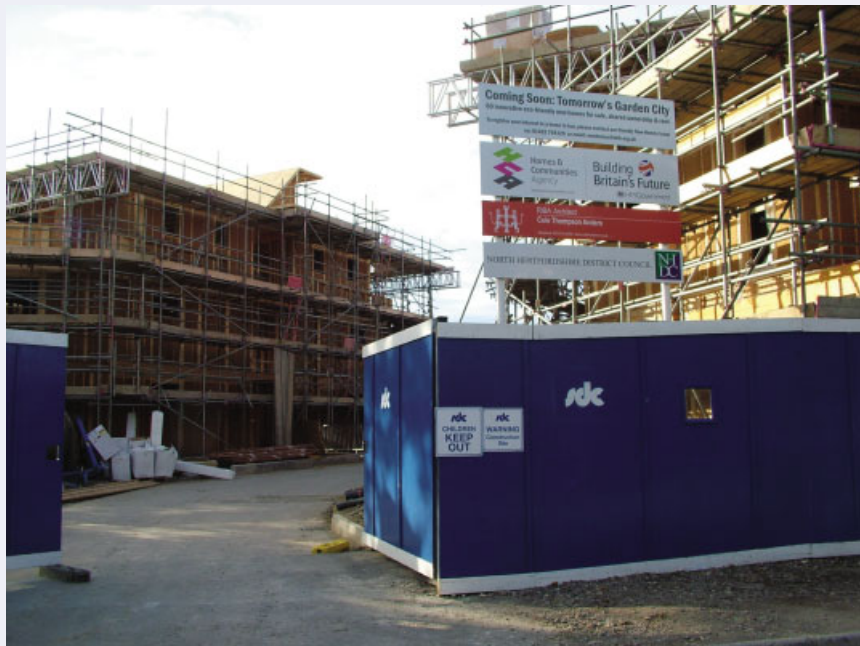
Figure 2.37 Letchworth: work in Progress on site
