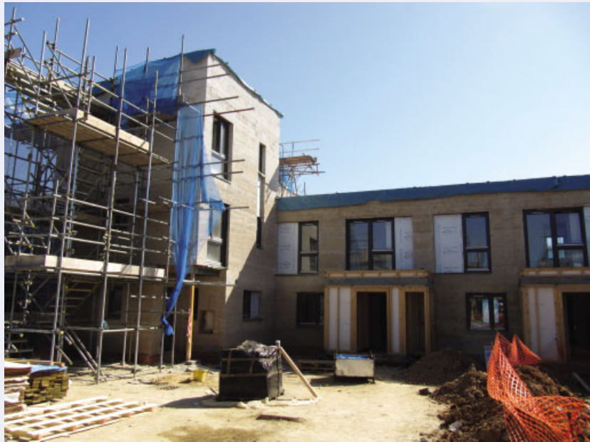
Figure 2.19 Callowlands: hempcrete when scaffolding starts to come down. Reproduced by permission of Luke Brooker MSc, The Airey Miller Partnership.
