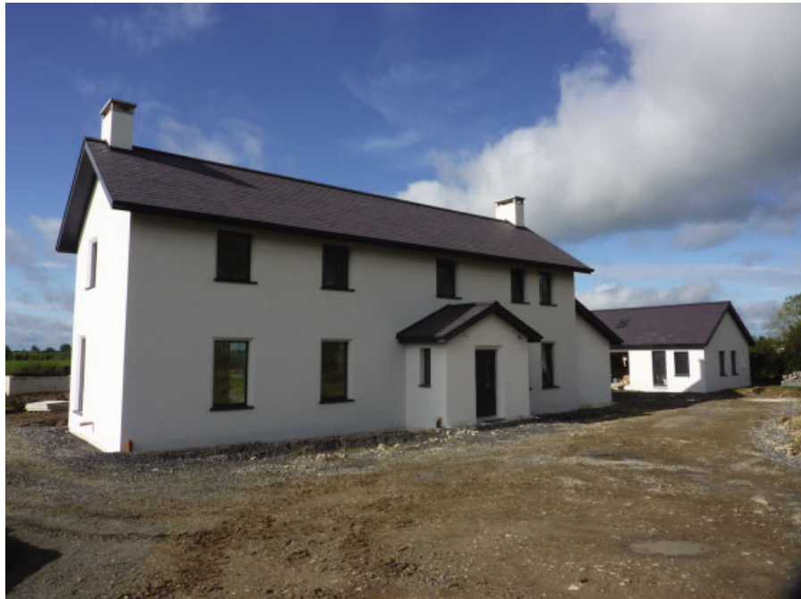
Figure 7.4 Longford hemp house designed by Winkens. Reproduced by permission of Winkens Architecture.
