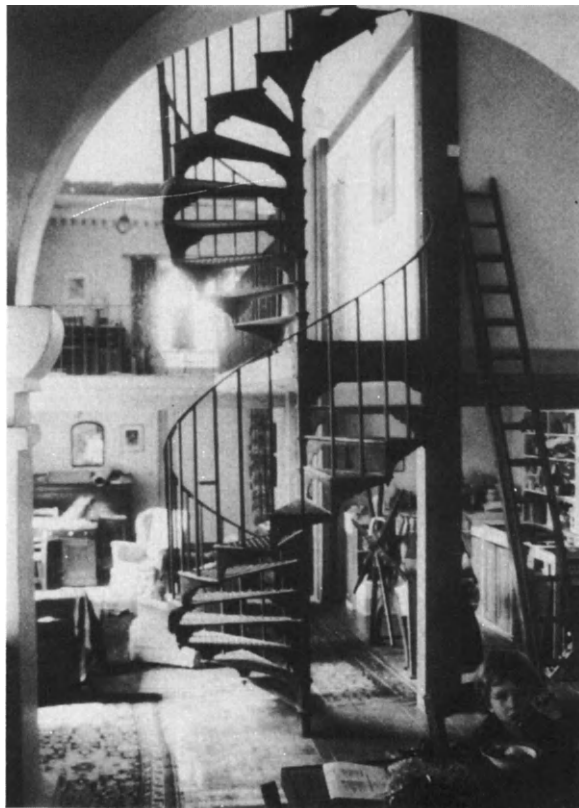
Interior ground level
