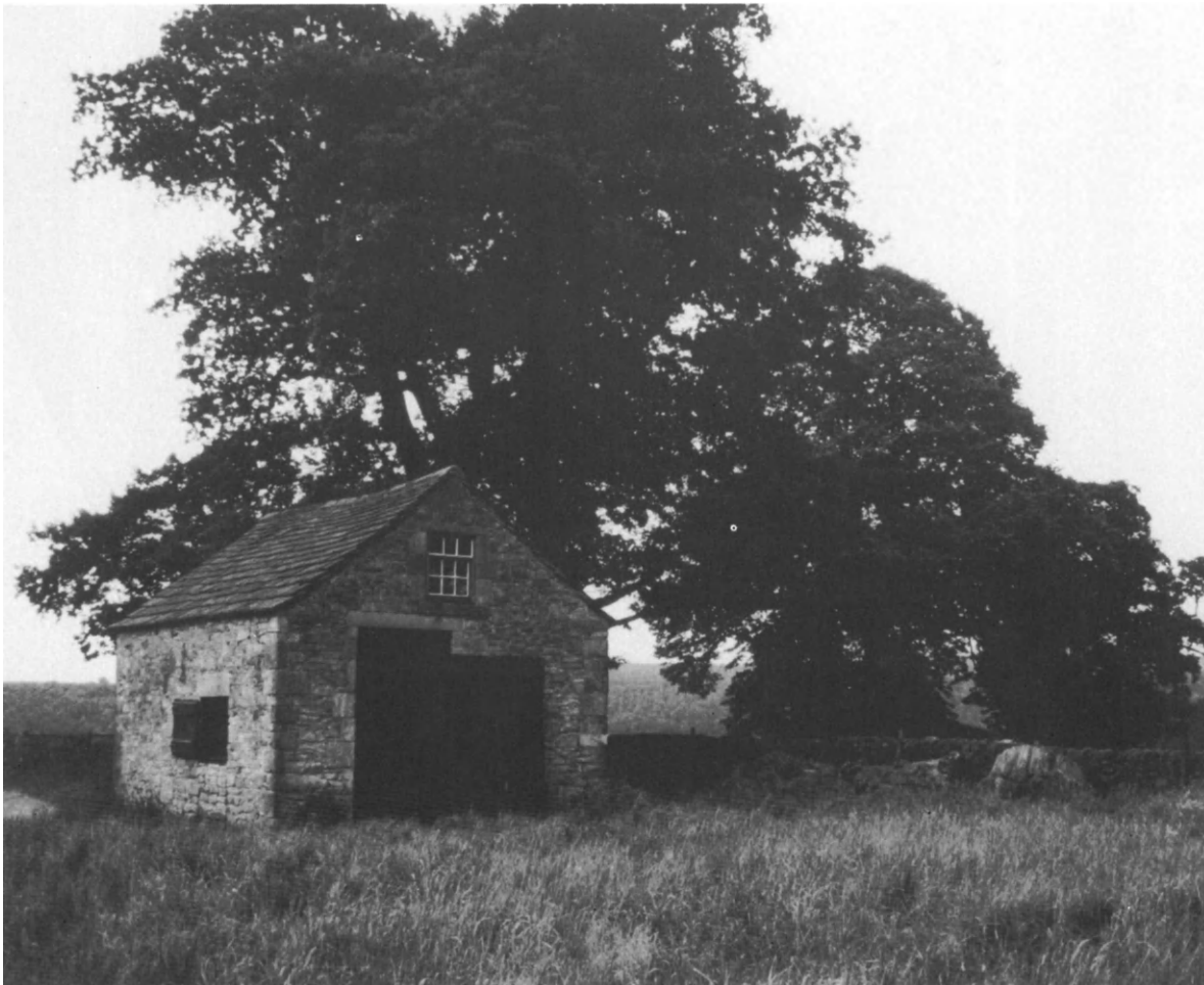
A typical field barn
