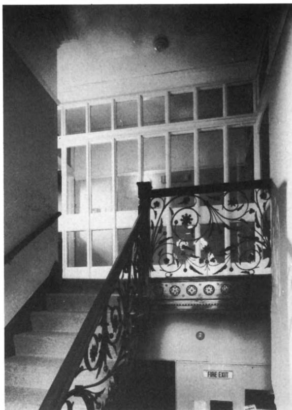
The staircase, showing the fire screen
