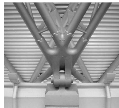
11.11 Casting for pinned connections at Ponds Forge, Sheffield (architect: FaulknerBrowns)
