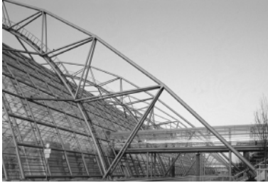
4.21 Leipzig Messe — external structure supporting glazing (architect: Von Gerkan Marg & Partners and Ian Ritchie)
