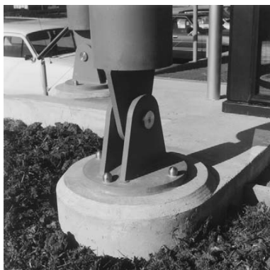
6.13 Typical pinned connection to a foundation
