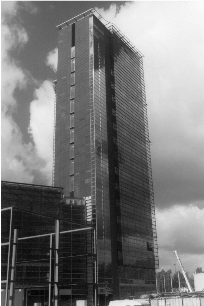
11.4 Use of weathering steel in the Baltic Square Tower in Finland (architect: Helin & Co.)
