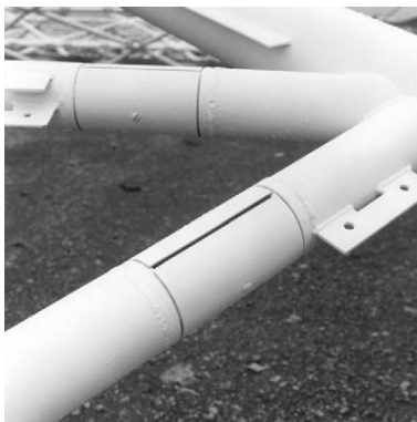
6.10 Connection with cover plate
