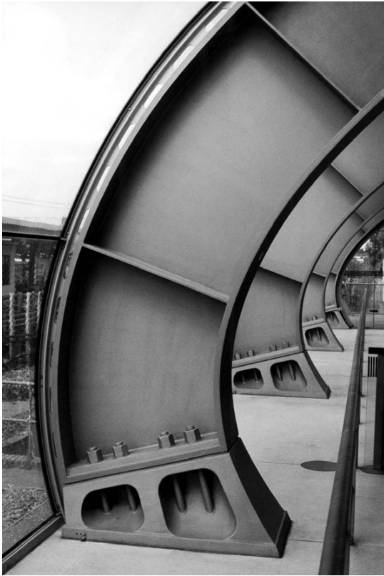
2.14 Curved fabricated beam at Stratford Station, London (architect: Wilkinson Eyre)
