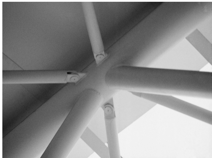
6.16 Welded connection of CHS bracing members to CHS chord
