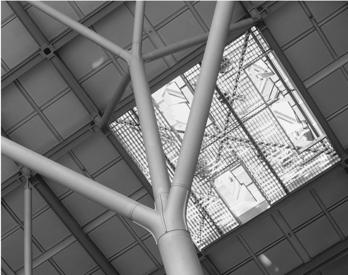
11.10 Tubular connections of 'trunk' to 'branch' at Stuttgart Airport (architect: Von Gerkan Marg & Partners)
