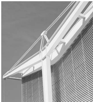
2.11 Tied column used for architectural effect at Stockley Park, London (architect: Foster and Partners)
