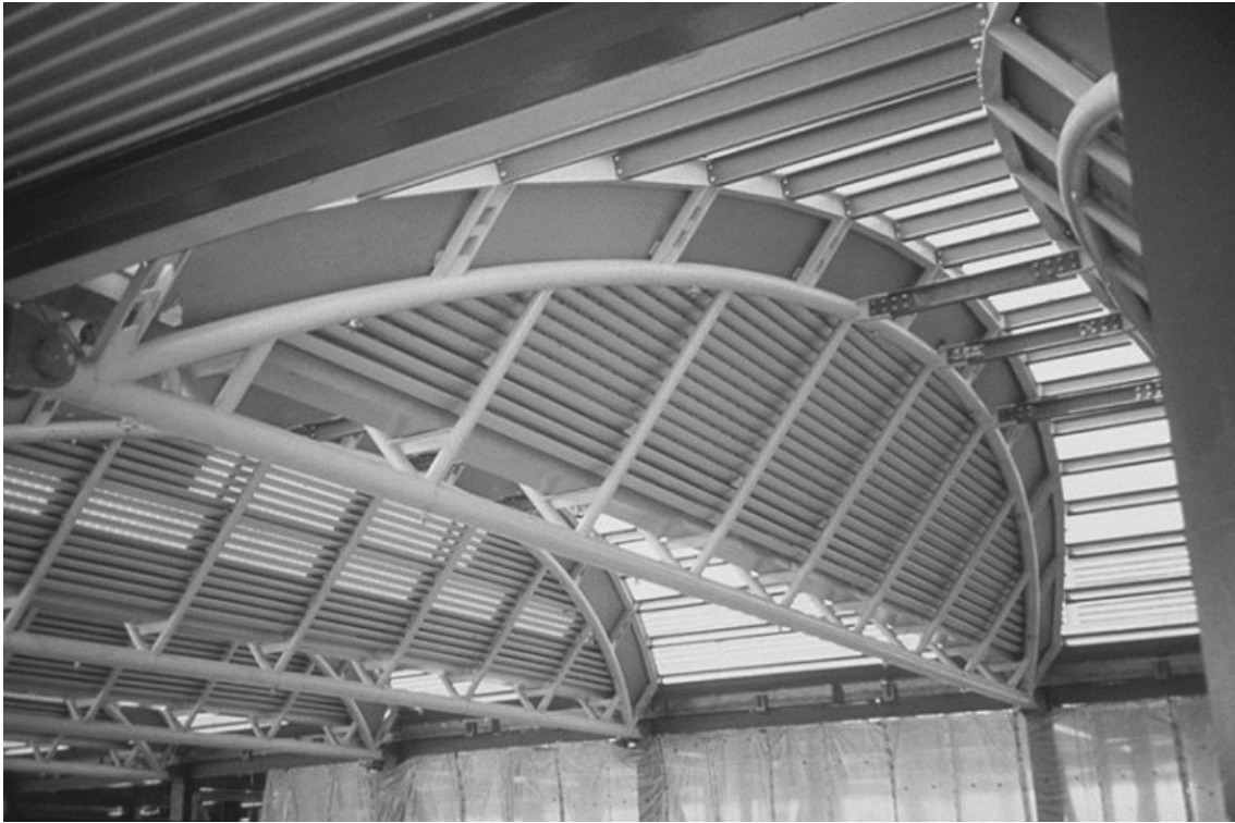
13.7 Curved water-filled roof trusses at the HACTL Superterminal One Cargo Handling Facility, Hong Kong International Airport (architect: Foster and Partners)
