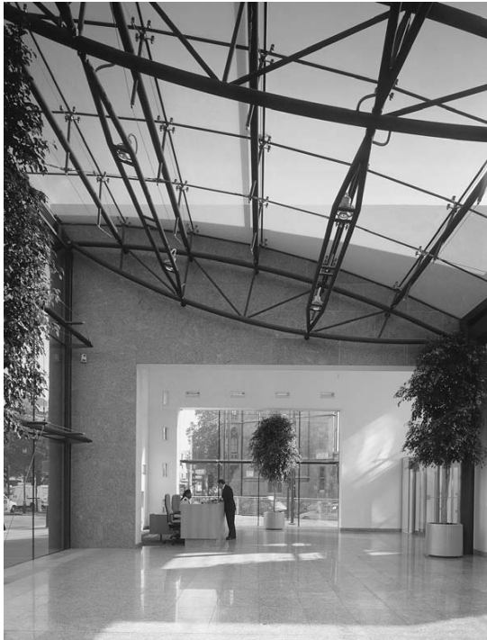
9.16 Curved truss used to support the roof of the Department for Trade and Industry building (architect: DEGW)
