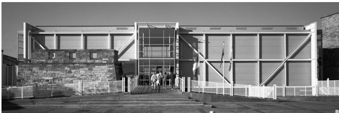
2.4 Visitor centre, Limerick, Ireland. The structure of the building is expressed on the outside, including the vertical bracing (architect: Murray O'Laoire Associates)
