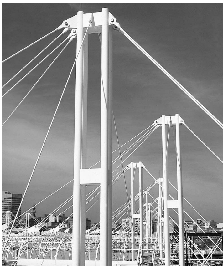
6.11 Column cluster arrangement at Darling Harbour, Sydney (architect: Philip Cox & Partners)
