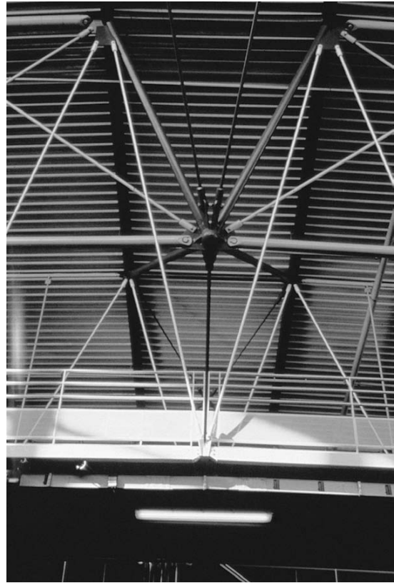
11.7 Cast node between tension members at L'Oreal, Paris
