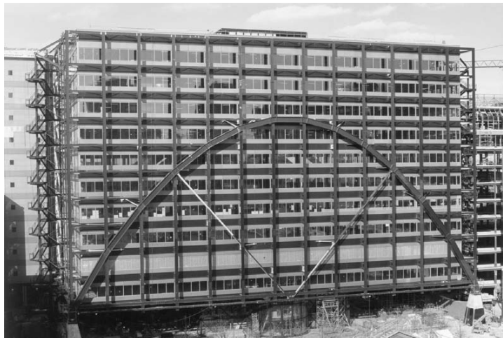
2.5 Internal arch structure over railway lines at Broadgate, London (architect: Skidmore Owings & Merrill)
