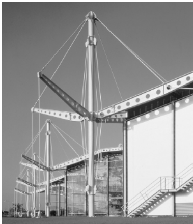
1.2 The Renault Parts Distribution Centre, Swindon, showing mast and tension structure (architect: Foster and Partners)
