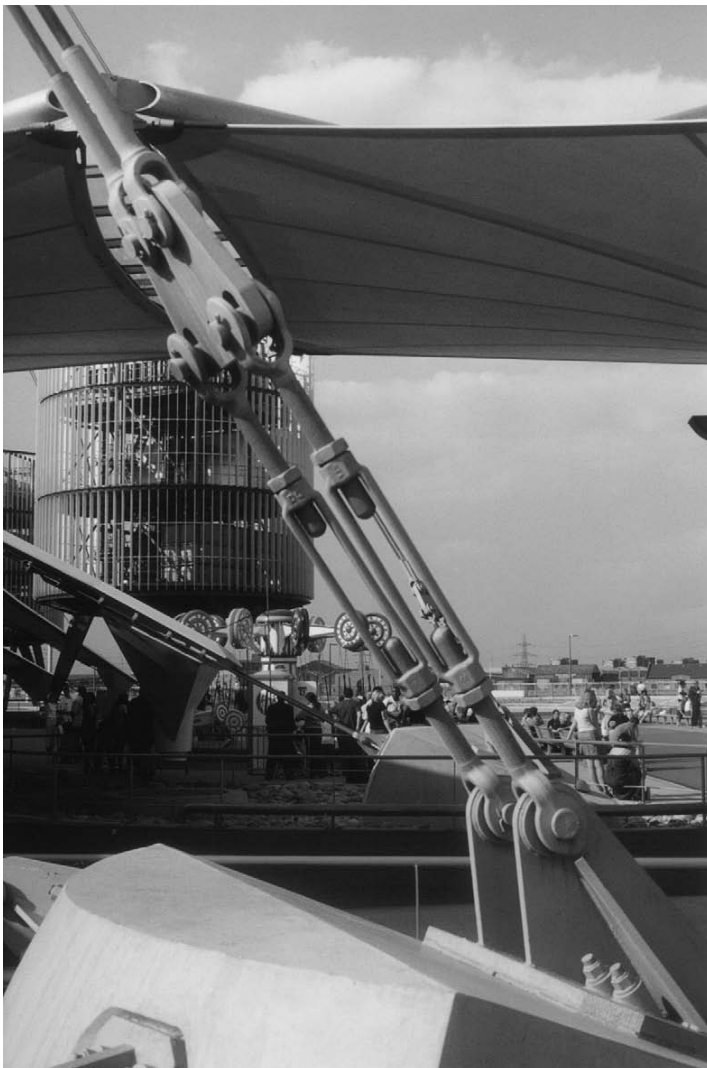
7.32 Coupler device used for an X-braced connection
