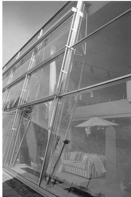
9.17 Inclined trusses to support a glazed wall
