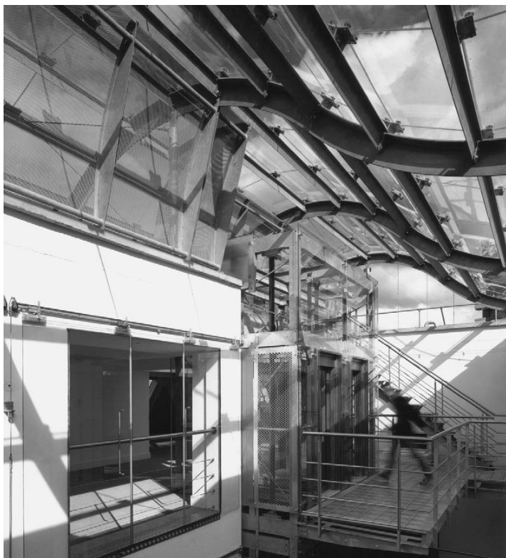
9.1 Glazing attachments to curved roof beam (architect: Jestico and Whiles)
