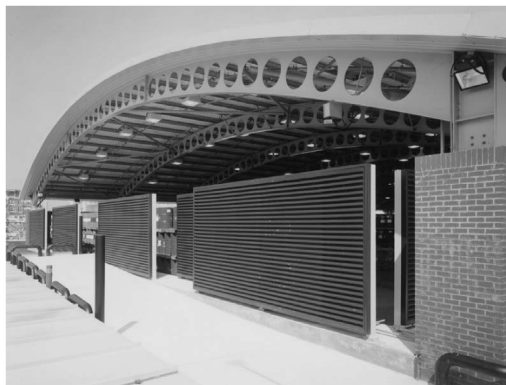
3.2 Portal-frame structure created using cellular beams
