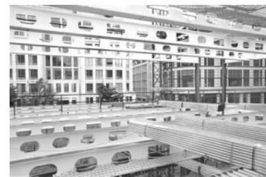
4.11 Fabricated beams with multiple openings
