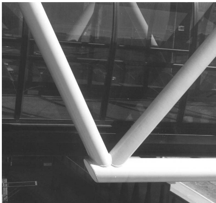
6.21 Example of welded CHS connection in a truss
