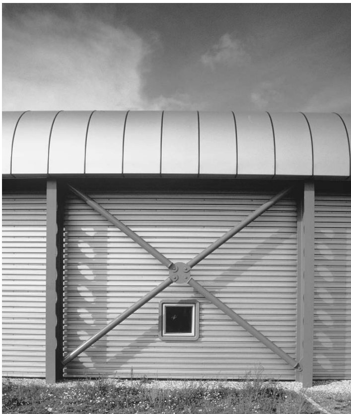
3.19 X-bracing using CHS sections used at a sports centre in Hampshire (architect: Hampshire County Council)
