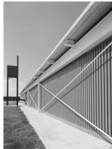
2.3 Reliance Controls, Swindon, with multiple braced panels (the stubs of the steel roof beams were left exposed to facilitate easy extensions to the factory) (architect: Foster and Partners)
