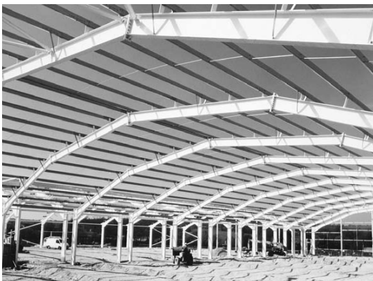
3.11 Long-span portal frame used to create an arch structure
