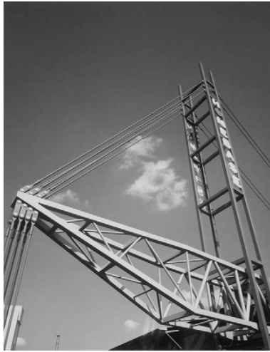
2.9 Homebase, London, showing a central spine supported by tension rods from mast (architect: Nicholas Grimshaw & Partners)
