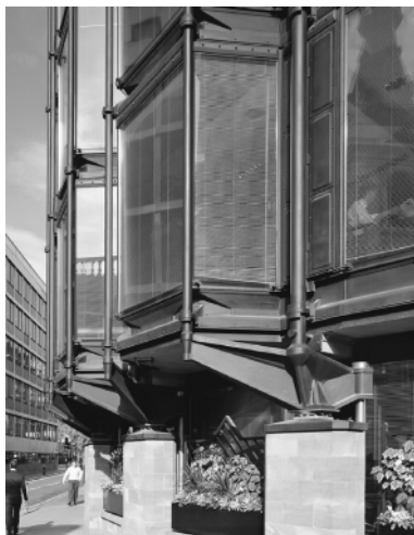
11.5 Cast bronze supports to cladding system, Bracken House, London (architect: Michael Hopkins and Partners)
