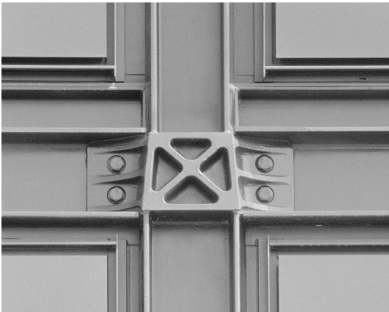
11.8 Cast node between beams and columns at New Square, Bedford Lakes, London — see also Colour Plate 12 (architect: Michael Hopkins and Partners)
