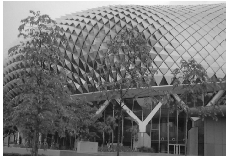
8.7 Mero space frame incorporating solar shading ,used in the Esplanade Theatre Complex, Singapore (architect: Michael Wilford & Partners and DP Architects Pte Ltd)
