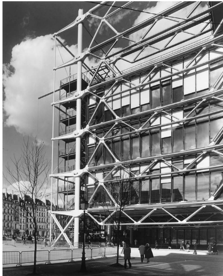
3.14 Example of continuity achieved through a series of pinned connections, Centre Pompidou, Paris (architect: Renzo Piano and Richard Rogers)
