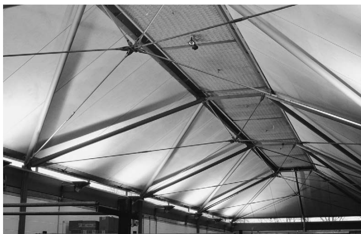
4.37 Inclined tubular trusses to create a folded plate roof (architect: Haworth Tompkins Architects)
