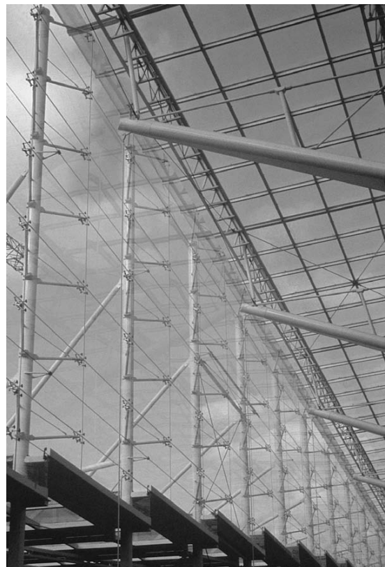
9.15 Tubular mullion used to support a tall glazed wall (architect: RFR)
