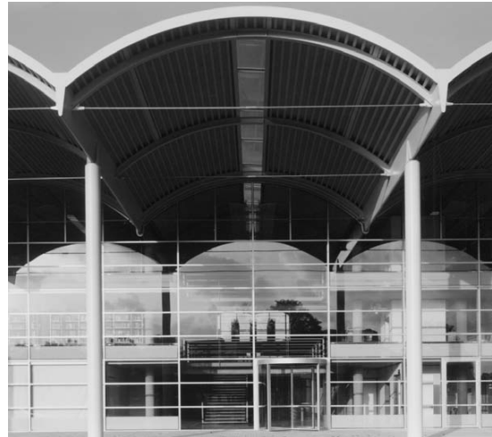
2.15 Fabricated V beam of Cranfield Library (architect: Foster and Partners)
