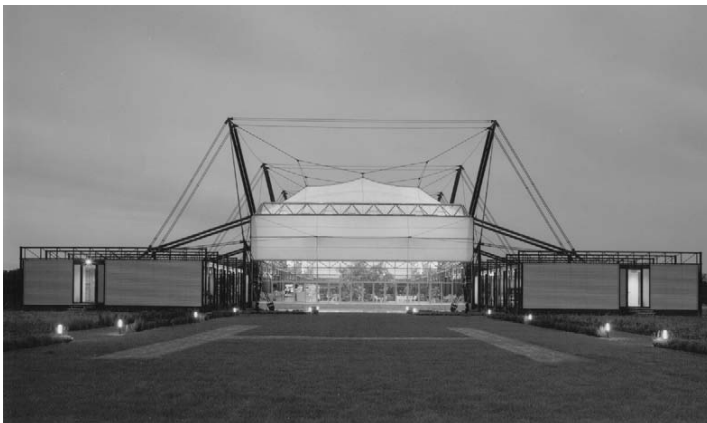
7.1 Tension-tye structure used to support a membrane roof at the Schlumberger Research Centre, Cambridge (architect: Michael Hopkins & Partners)
