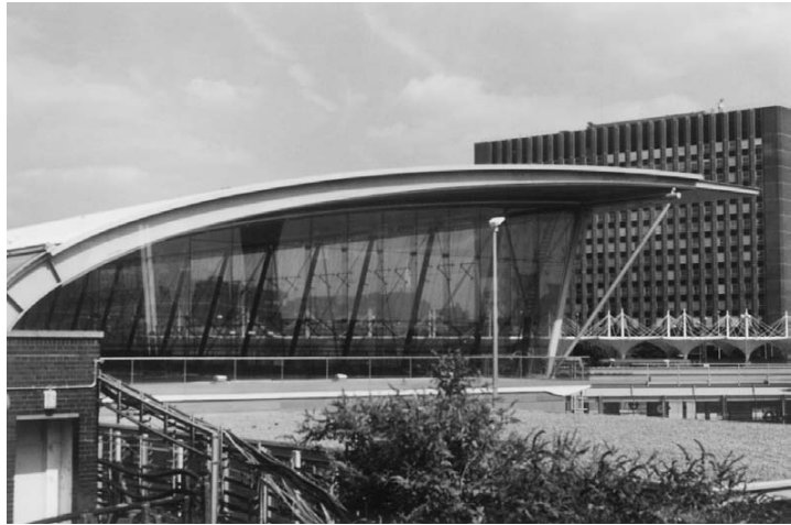
2.18 Stratford Station showing use of repetitive curved frames (architect: Wilkinson Eyre)
