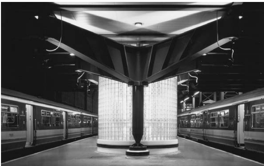
1.8 Operations Centre at Waterloo, London, showing a fabricated cantilever beam supporting a walkway (architect: Nicholas Grimshaw & Partners)
