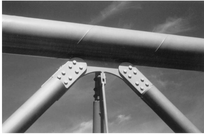
6.23 Architectural use of a bolted gusset-plate connection in a lattice truss for a railway bridge
