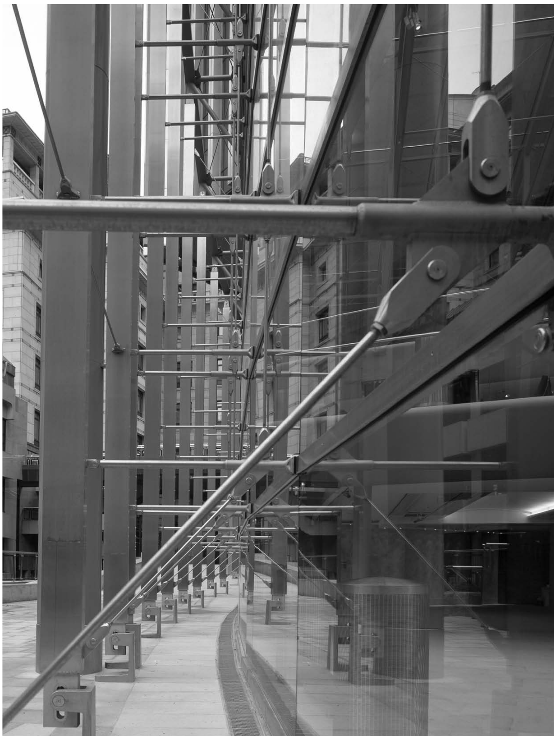
11.3 Entrance lobby to Tower 42, London, showing stainless steel mullions and tie rods (architect: DEGW)
