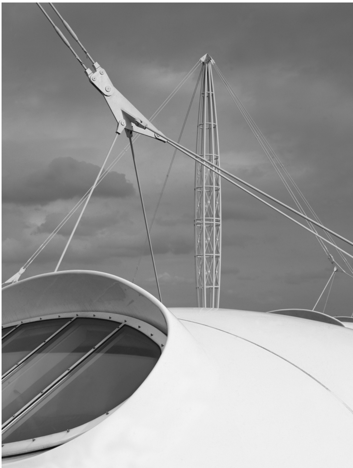
7.8 Fabricated fork detail at Igus Factory, Cologne (architect: Nicholas Grimshaw & Partners)
