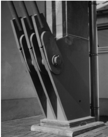
7.9 Column base attachment for tension rods at sports stadium, Cologne (architect: Verena Dietrich)
