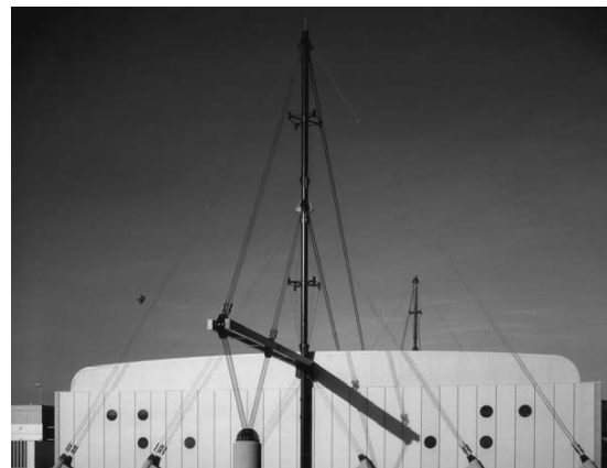
7.3 Oxford Ice Rink with discrete foundation supports (architect: Nicholas Grimshaw & Partners)
