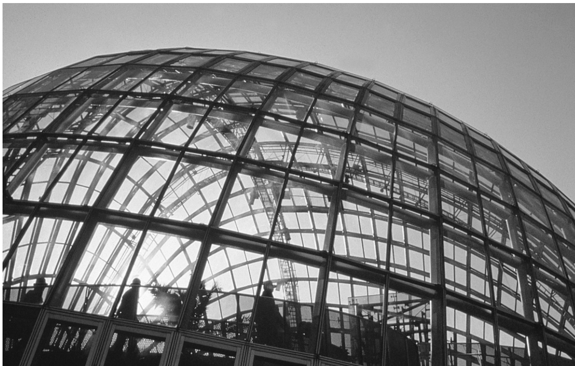
9.2 Shell structure clad in glazing at the Museum of Fruit, Yamanashi, Japan (architect: Itsuko Hasegawa)
