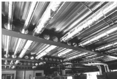
4.4 Cellular beam shows integration of circular service ducts
