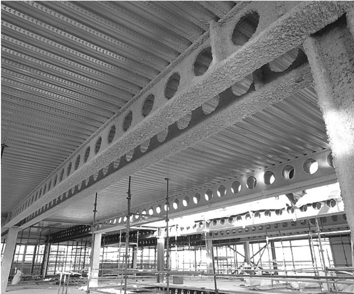
13.1 Sprayed protection to cellular beams
