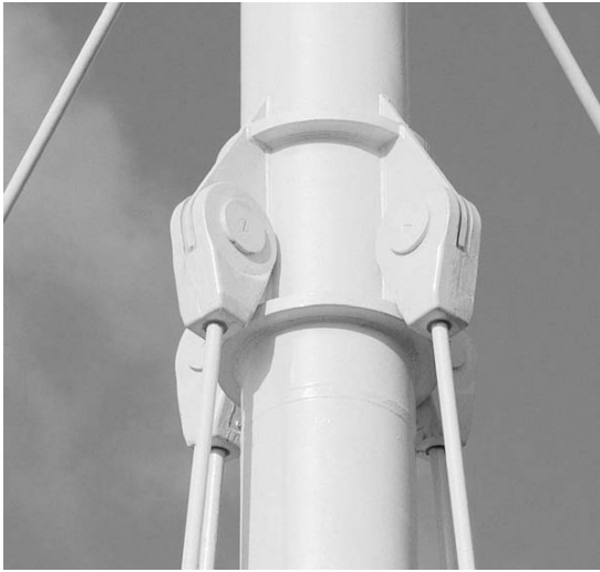
7.5 Intermediate attachment to column in the Renault Parts Distribution Centre (architect: Foster and Partners)
