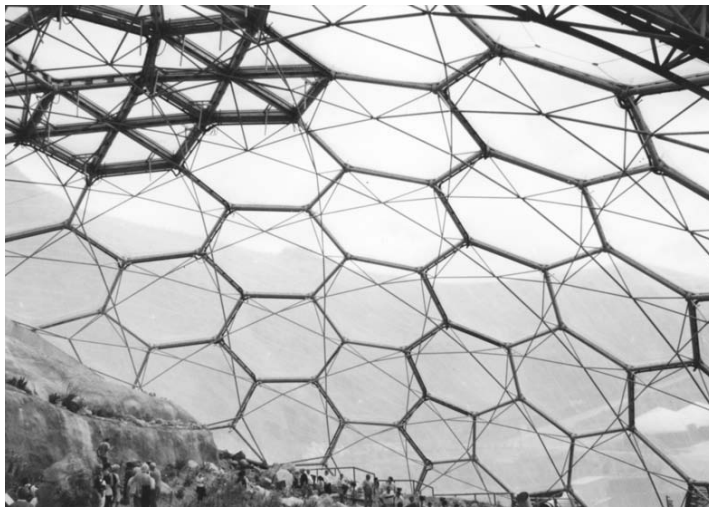
8.6 MERO space-frame node used in the Eden Project, Cornwall (architect: Nicholas Grimshaw & Partners)
