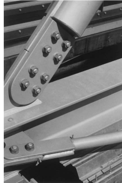
6.5 Spliced connection between CHS and an I-beam
