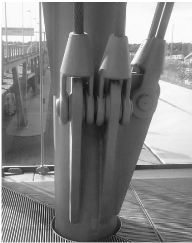
6.7 Connection of ties to tube at Cologne Airport (architect: Murphy Jahn Architects)
