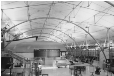
4.18 TGV station at Lille, showing the use of a tubular tied arch structure
