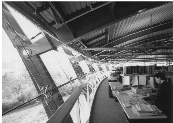
10.5 Steelwork penetrating the façade of the Western Morning News building, Plymouth (architect: Nicholas Grimshaw & Partners)
