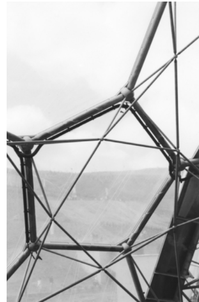
8.6 MERO space-frame node used in the Eden Project, Cornwall (architect: Nicholas Grimshaw & Partners)
