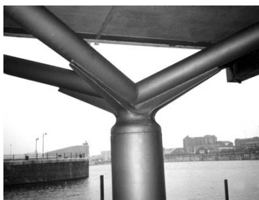
14.3 Complex welded node of tubular column
