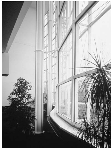
6.30 Royal Life UK headquarters — steel tubular column with four pairs of fins (architect: Arup Associates)
