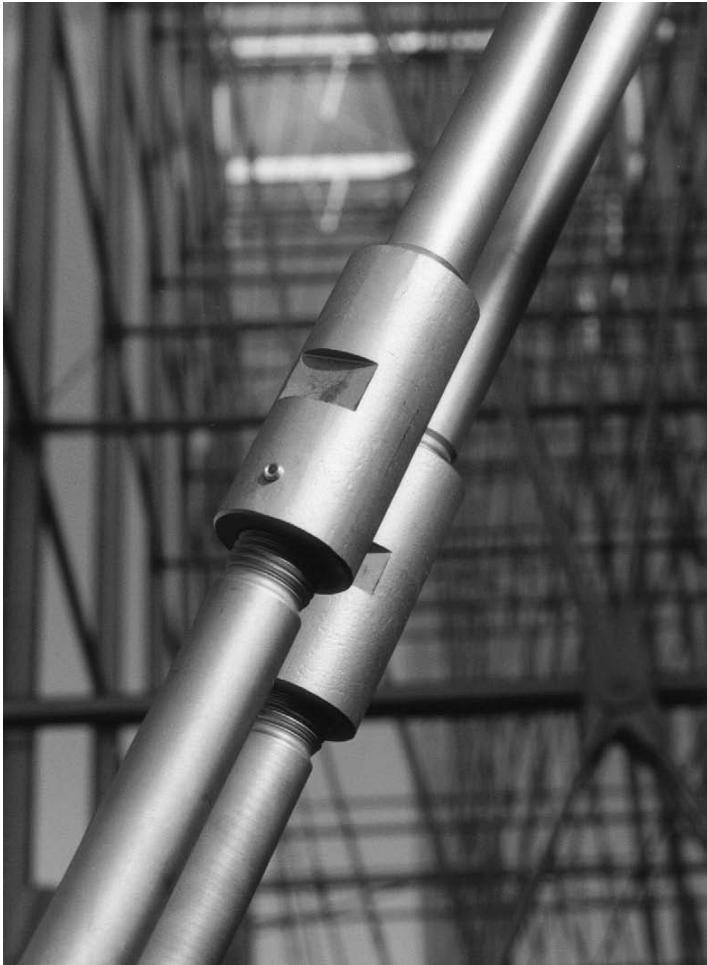
7.13 Typical coupling between stainless steel bars
