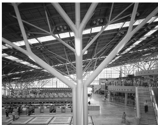
1.12 Stuttgart Airport Roof using tubular column ‘trees’ — see also Colour Plate 9 (architect: Von Gerkan Marg & Partners)
