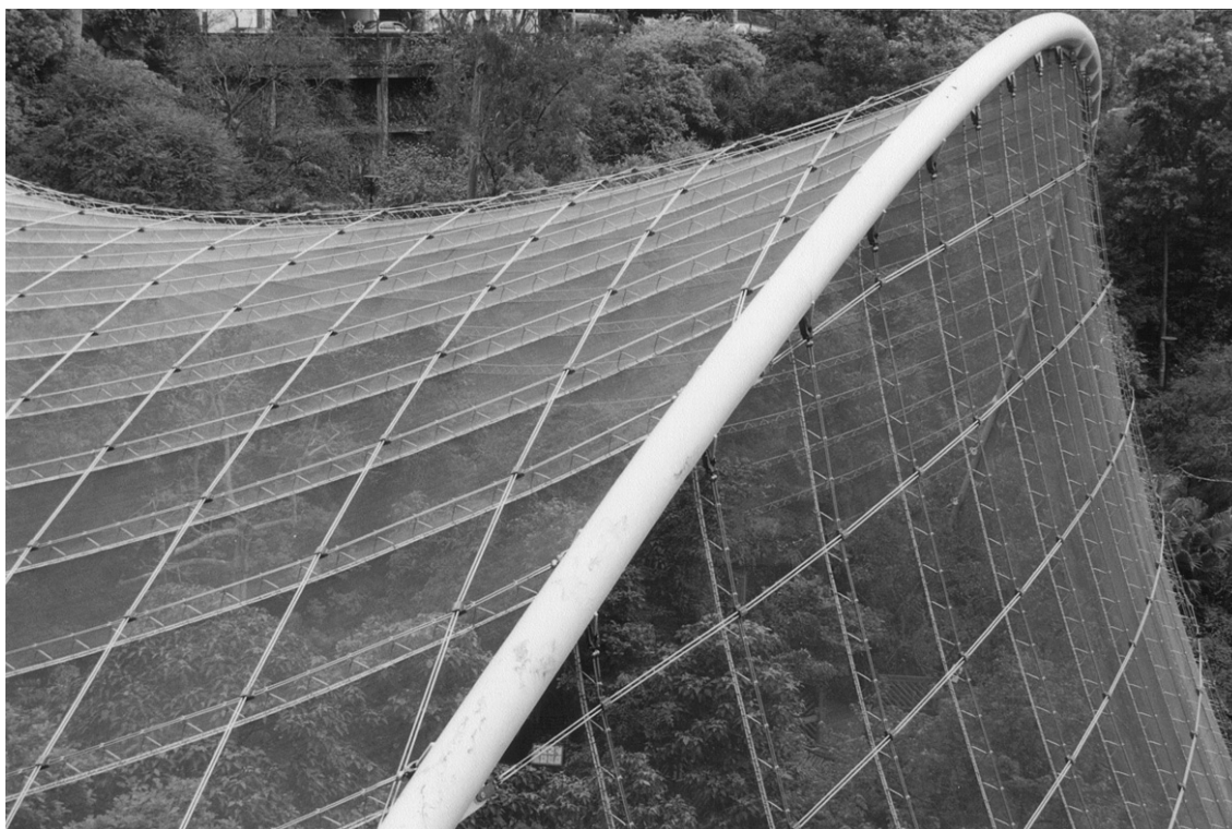
7.39 Tubular arch used to support a cable structure in the Hong Kong Aviary (architect: Hong Kong Architectural Office)
