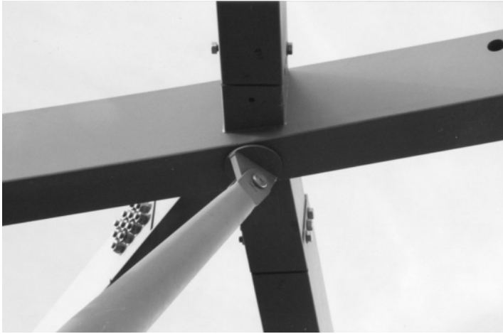
6.32 'Hybrid' welded and bolted connection
