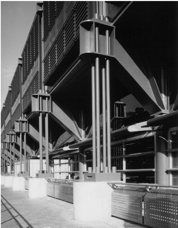
7.7 Tension anchors to cantilever beams at Sainsbury's supermarket, Camden, London (architect: Nicholas Grimshaw & Partners)
