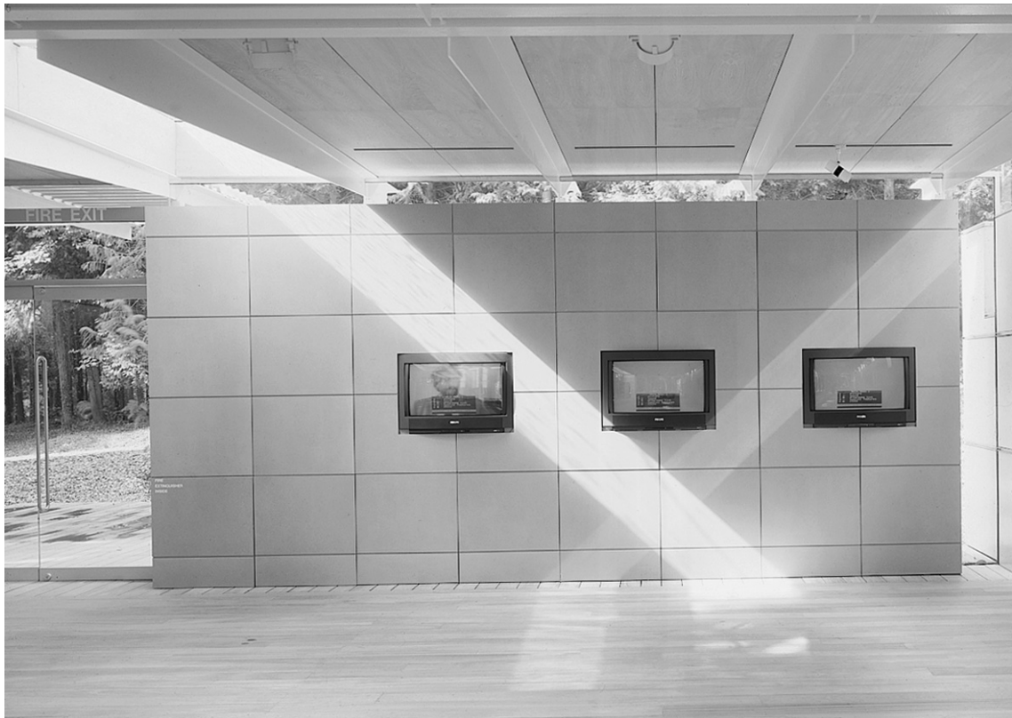
10.4 Tapered beams (T-sections) penetrating glazed envelope — Hat Hill visitor's centre, Goodwood, Sussex (architect: Studio Downie)
