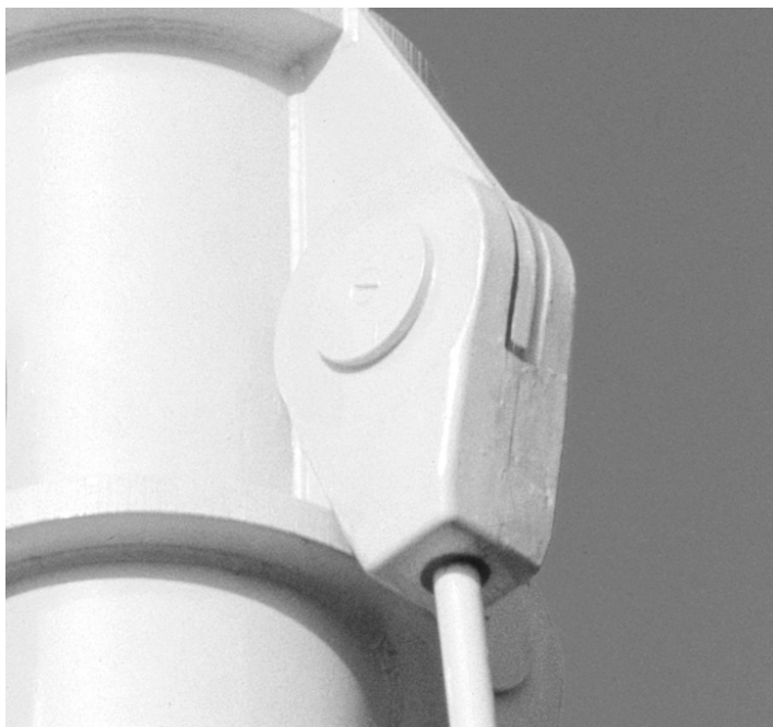
7.15 Sealant applied between fork and plate at the Renault Parts Distribution Centre, Swindon (architect: Foster and Partners)
