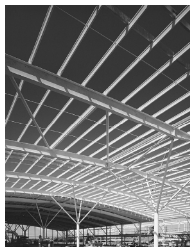
3.16 Portal-frame effect created using inclined pinned members
