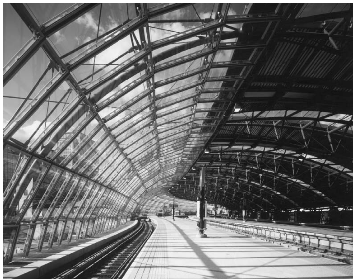
1.11 Waterloo International Terminal, striking long-span roof comprised of tapering tubular trusses (architect: Nicholas Grimshaw & Partners)
