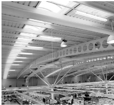
4.15 Cellular beams used in an Asda store, Tamworth
