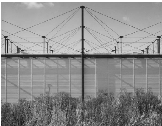
7.2 Fleetguard, Quimper, in which heavy loads were supported by the primary structure (architect: Richard Rogers Partnership)
