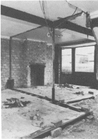
Figure 7 View of internal steelwork showing main floor support at midspan
