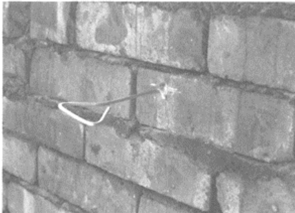
Figure 10 New stainless steel wall tie fixed with resin
