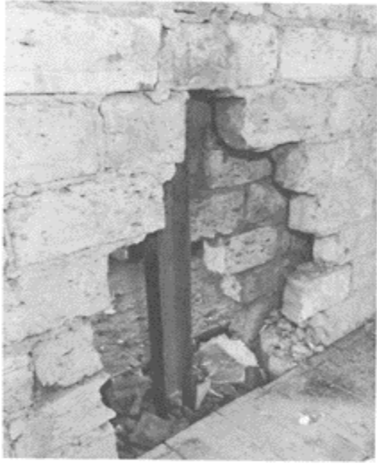
Figure 6 Steel frame embedded within party wall
