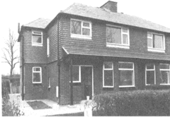
Figure 13 External view of the completed houses
