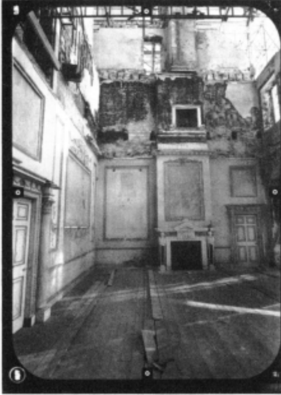
Figure 3.4 Uppark House, salon. One of the UMK photographs used in the preparation of the elevation shown in Figure 3.5. The ground floor salon was mostly undamaged, unlike the first- and second-floor levels. (Reproduced with the permission of the National Trust; Architects, The Conservation Practice.)
