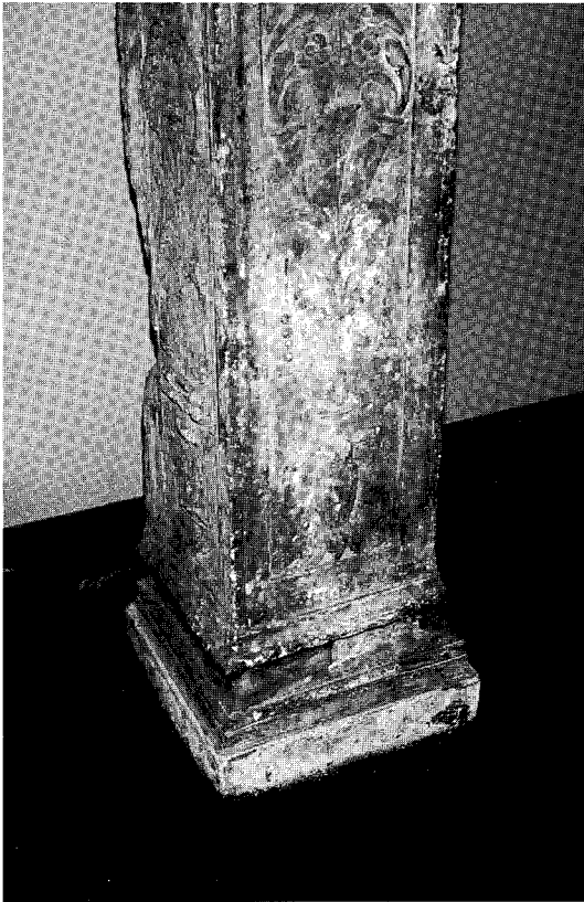
Figure 11.1 Detail of carved plinth, showing spalling caused by the migration of soluble salts in cement
