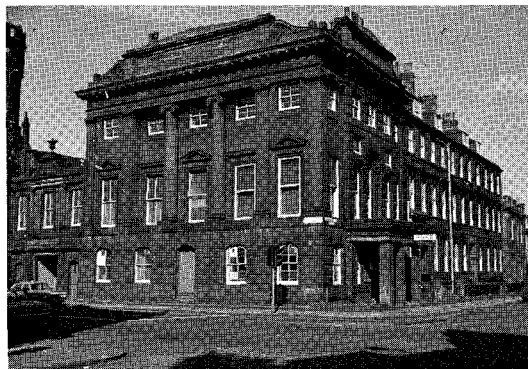
Figure 8.4 The soiling pattern in this illustration of a sandstone building in Leith (Scotland) is clearly different to that of Figure 8.1. In this case the most exposed features are the most heavily blackened
