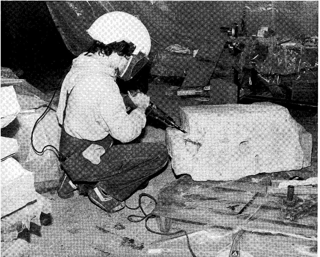
Figure 12.3 Lead being extracted from hole for hinge bracket (bracket visible at lower right). In the Burrell Collection, Glasgow
