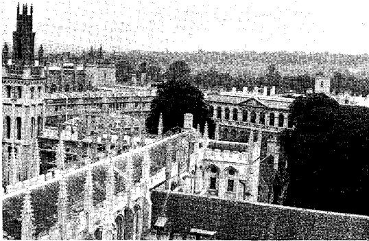
Figure 1.27 Wall head maintenance is just as critical in an occupied building but the situation is less of a philosophical problem. This building complex in the university city of Oxford has had a long history of repair and maintenance which includes essential replacement of copings and weatherings when they fail but also preserves the architectural integrity by replacement of decayed pinnacles
