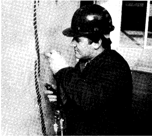
Figure 2.26 Injecting resin to repair masonry cracks
