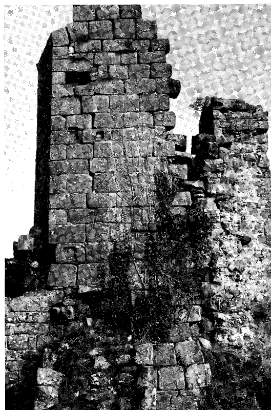
Figure 1.5 Developing fractures may take decades to become serious, but may also fail with surprising rapidity, especially when temperature extremes, such as a long dry summer or severe freeze-thaw cycling at the end of the winter, interfere with the normal equilibrium. Recording and monitoring of fractures, and temporary support, are desirable if not essential
