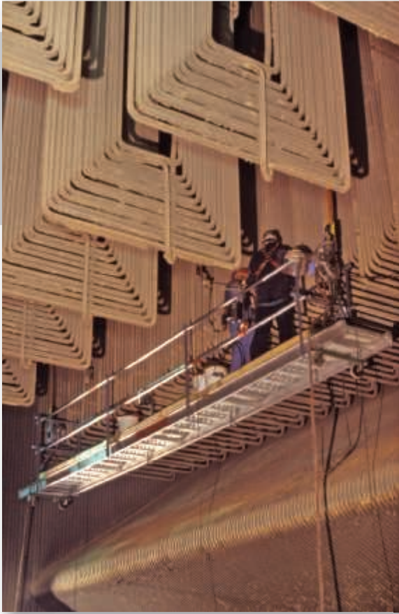
Two employees are on scaffolding near the top of Stanton Energy Center's 23-story high boiler, checking and repairing super heaters.
