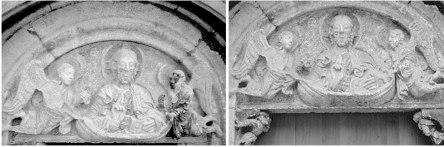
Fig. 7.37 View of Romanesque portal of St. Ulrich church in Regensburg/Germany. State 1985 during cleaning intervention ( left ) and 10 years later ( right )
