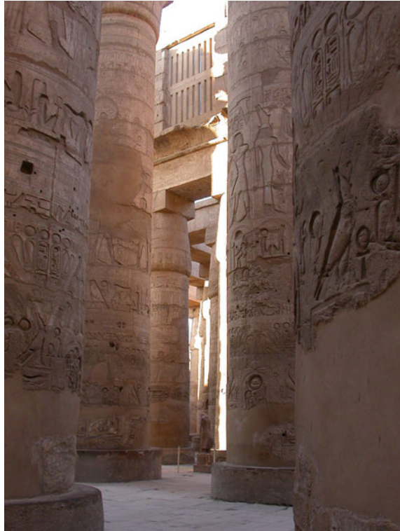
Fig. 1.4 Columns in the Karnak Temple in Luxor, Egypt. The thickness of the cross-beams on top of the columns takes into account the low bending strength of the sandstone
