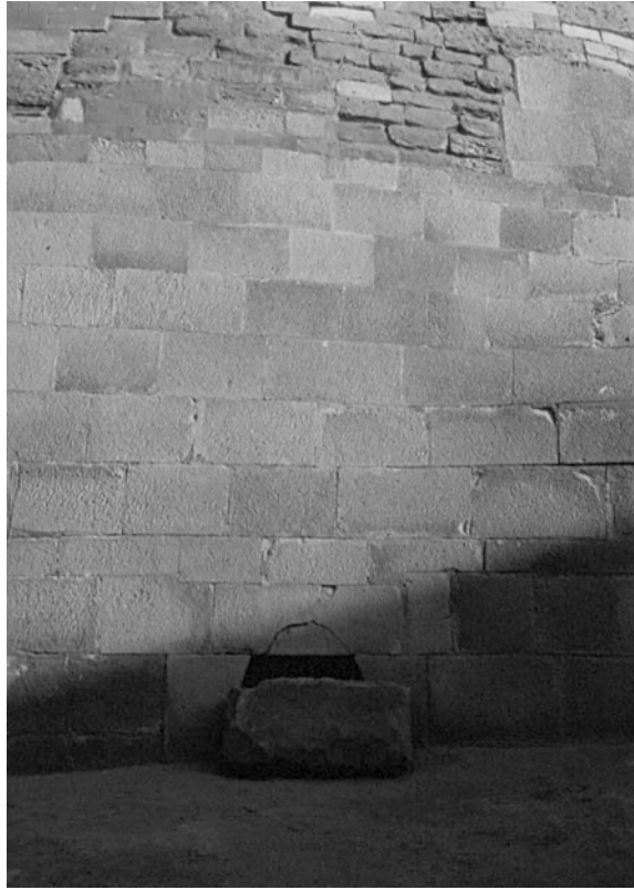
Fig. 7.1 Great Sphinx in Gizah. Replacement stone from the first restoration under Pharaoh Thutmose IV
