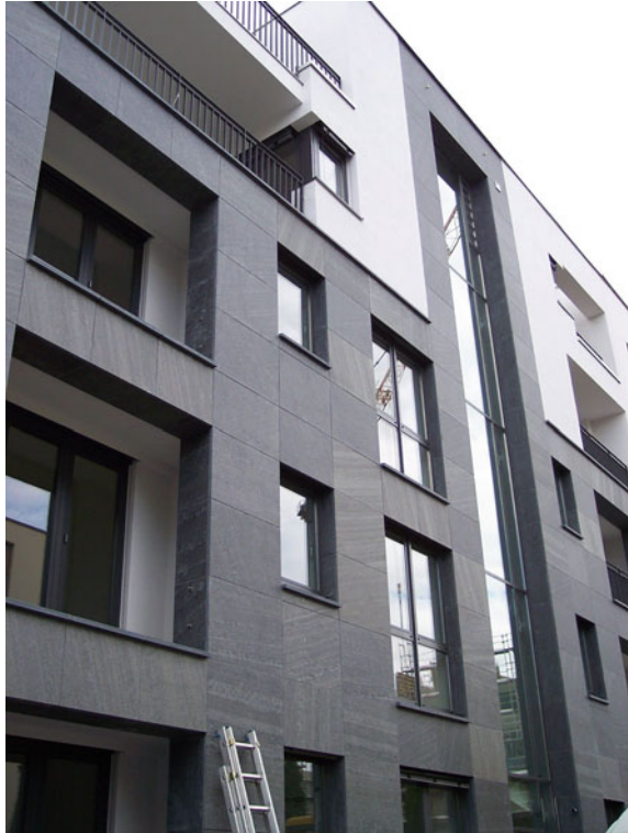
Fig. 2.48 Building clad with the Knotenschiefer (knotted slate) of Theuma. The very specific decor is due to the contact metamorphic overprint, which had produced the mineral growth (Natursteinwerk Theuma AG, Theuma in Germany)
