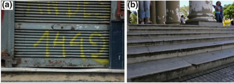
Fig. 3.67 Carrara Marble stairs in (a) in Montevideo (Uruguay) and (b) in Buenos Aires (Argentina) clearly show differential abrasion
