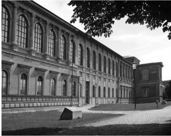
Fig. 7.80 View of the south façade of Alte Pinakothek Munich, Germany
