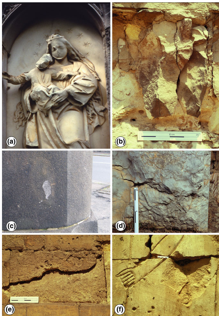
Fig. 6.9 Detachment 2: a disintegration—sugaring of marble (Old Southern Cemetery, Munich, Germany), b disintegration—crumbling (limestone, mosque in Cairo, Egypt) (Figure by B. Fitzner), c blistering (granite, Church of Christ, Dresden, Germany), d fragmentation—splintering (limestone, Sanctuary of Demeter, Eleusis, Greece) (Figure by B. Fitzner), e contour scaling (limestone, masonry, Cairo, Egypt) (Figure by B. Fitzner), and f bursting (sandstone, Luxor Temple, Luxor, Egypt) (Figure by B. Fitzner)
