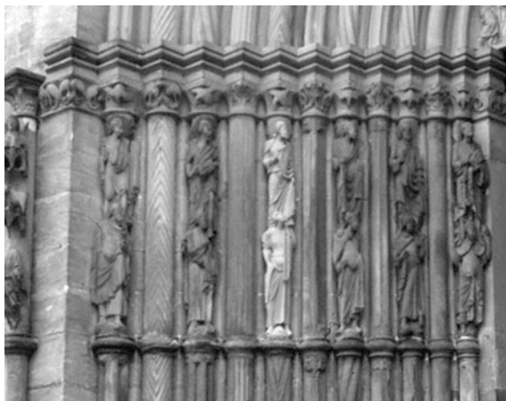
Fig. 7.13 The first epoxy bound replica ( light color ) of a pair of sculptures of the Fürstenportal at Bamberg Cathedral
