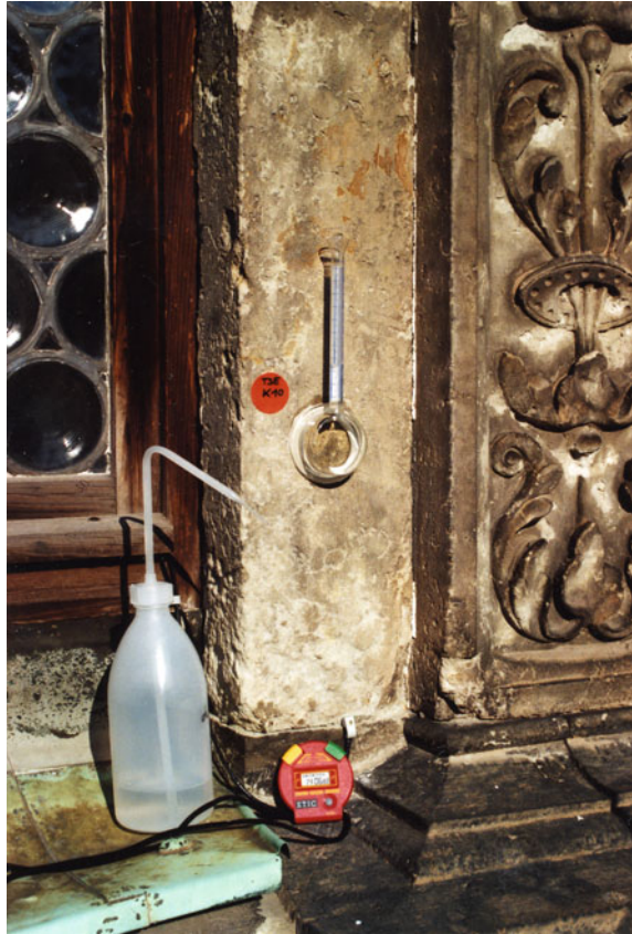
Fig. 6.34 Setup of the Karsten tube measurement on a facade
