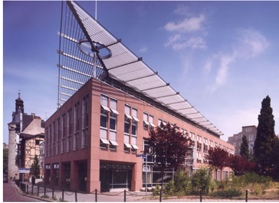
Fig. 2.34 Dresdner Bank in Halle (Germany) clad with the Löbejün Rhyolite (SH Naturstein, Löbejün in Germany)
