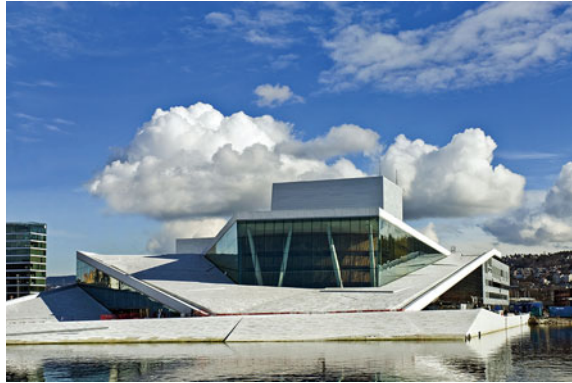
Fig. 2.45 The Oslo Opera House where the external facade is covered with Carrara Marble (Vando D'Angiolo, Campolonghi Italia Spa)
