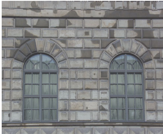
Fig. 7.60 Discolored stone repair mortars on Greensandstone ashlars at Residenz Munich, Germany
