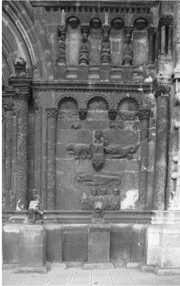
Fig. 7.25 White limestone surface lay open after detachment of black crusts. Romanesque portal of St. Jacob church Regensburg, Bavaria
