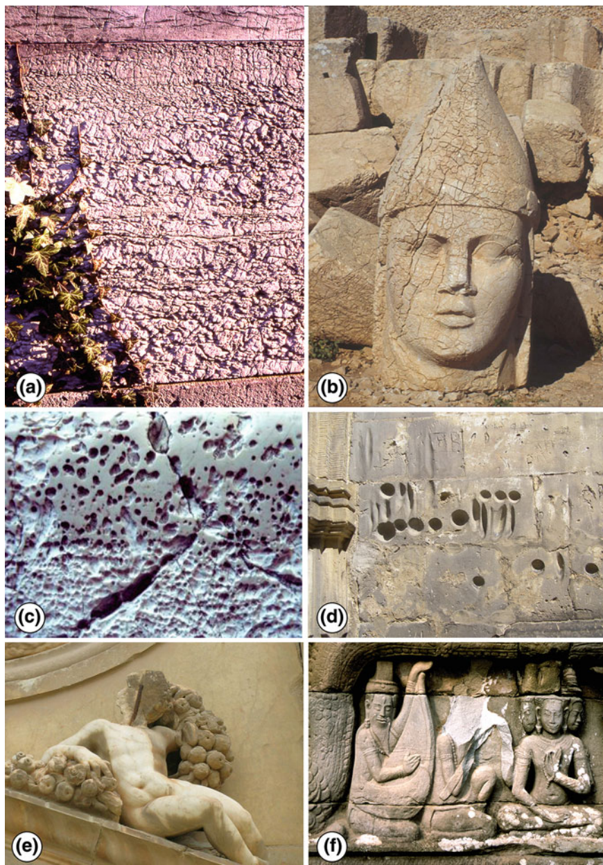
Fig. 6.11 Material loss 2: a microkarst (Munich in Germany) (Figure by W.-D. Grimm), b microkarst (limestone, Nemrud Dag, Turkey) (Figure by B. Fitzner), c pitting (marble, Rialto Bridge, Venice, Italy) (Figure by B. Fitzner), d cut (Quedlinburg in Germany), e missing part (Budapest), and f mechanical damage (sandstone, Banteay Chmar Temple, Cambodia)
