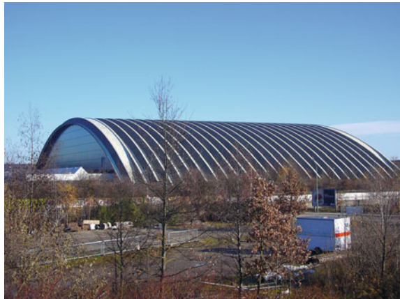
Fig. 1.9 Big hall of German Federal Mail in Munich, built 1965–1969. Length 124 m, height 31 m, width of the arch 146 m
