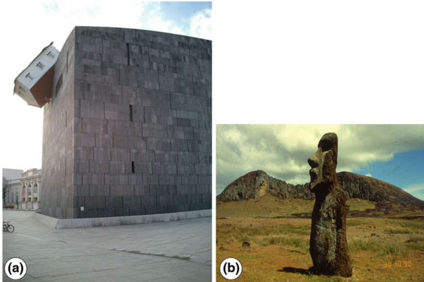
Fig. 2.38 a MUMOK Museum of Modern Art in Vienna (Austria) is clad with basaltic lava (Krings, Schmitz Naturstein GmbH & Co. KG), and b Moai from Easter Island in Chile is made from tuff (Figure by B. Fitzner)
