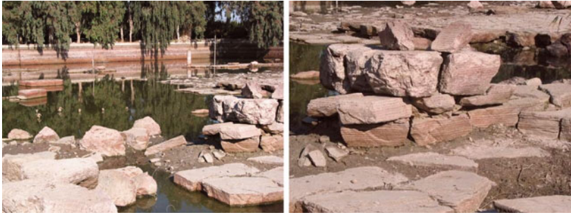
Fig. 4.30 Ephesus, Turkey: the rosy stain on white calcareous limestone is caused by bacteria-forming blooms in the brackish water of the pond overlaying the subterranean parts of the Artemision
