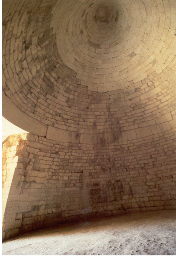
Fig. 1.5 View of the false vault in the Tomb of Atræus in Mykène, Greece
