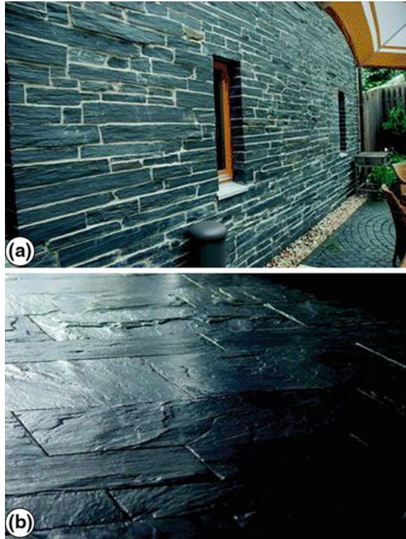
Fig. 2.40 Use of slate as cladding material: a The slate wall of Lotharheil and b Slate flooring tiles (Schieferwerk Lotharheil & Teichmann SchieferZentrum, Geroldsgrün in Germany)
