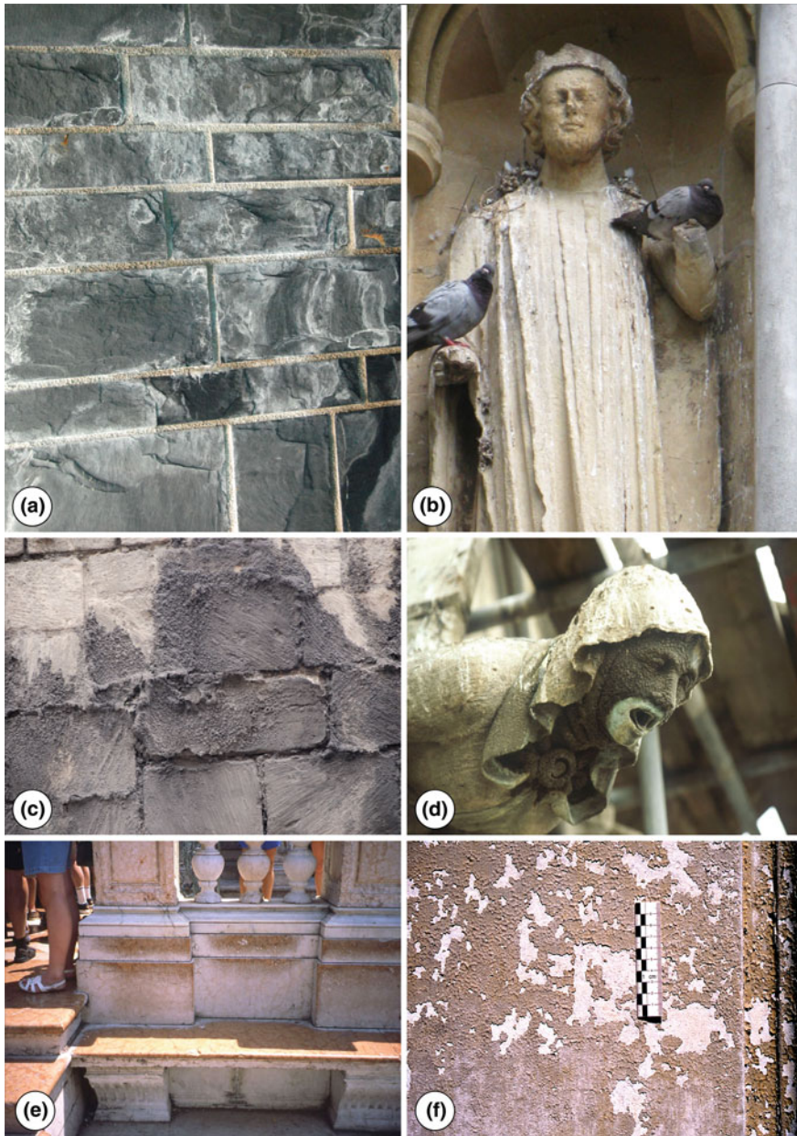
Fig. 6.12 Discoloration and deposit 1: a encrustation (slate, Bad Steeben in Germany), b deposit of pigeon droppings (limestone, Wells Cathedral, U.K.), c gypsum crust (limestone, Halle, Germany), d gypsum crust (limestone, Naumburg Cathedral, Germany) (Figure by B. Fitzner), e bleaching and glossy aspect (limestone, Piazza San Marco, Venice, Italy), and f film: old oil paint on sandstone (Dresden, Germany)
