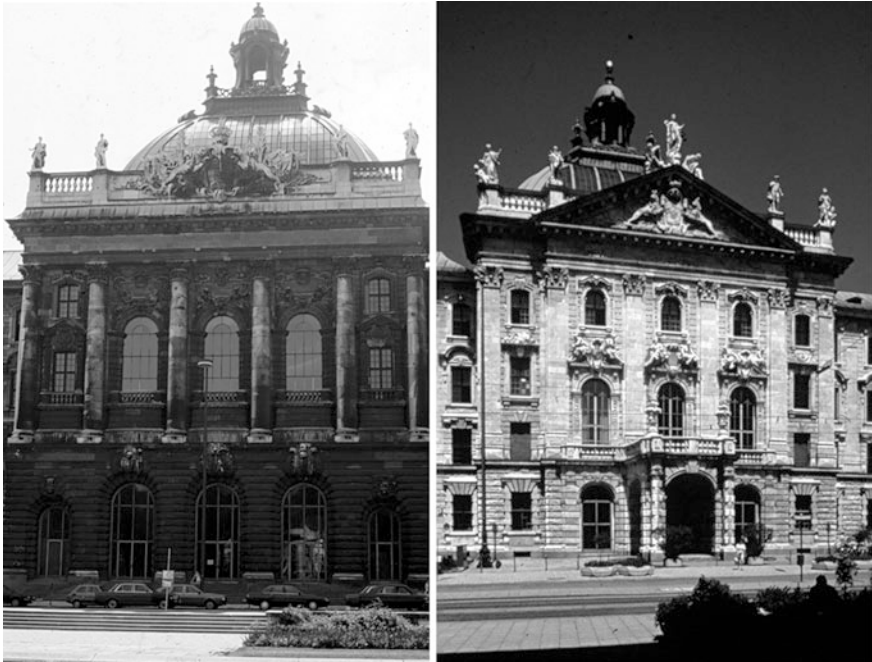
Fig. 7.31 Justice building in Munich before and after cleaning with JOS technique
