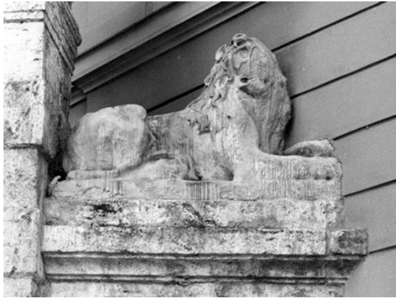
Fig. 7.78 Dark vestiges of rinsing rain drops on the hydrophobic surface. Lion on the Gate to Pranner Street Munich, Germany
