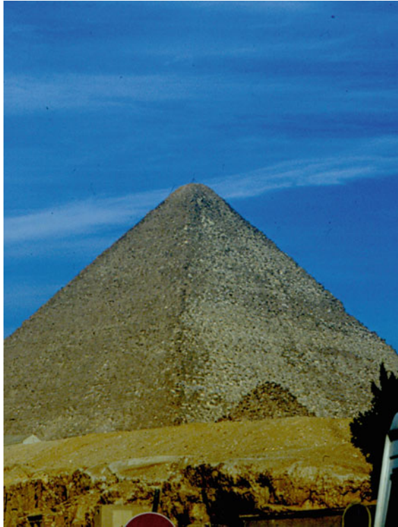
Fig. 1.3 View of the Cheops Pyramid. In spite of the height of 146 m, the pressure at the base is much less than the compressive strength of the limestone
