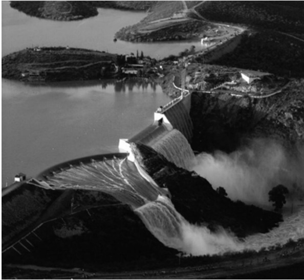
Figure 4. Francisco I. Madero Dam, one of the most important reservoirs in HAR6.
