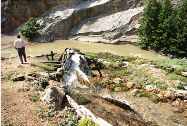
Fig. 3 Water elevated through a trench dug about 400 m upstreams, feeding the penstock of a water mill
