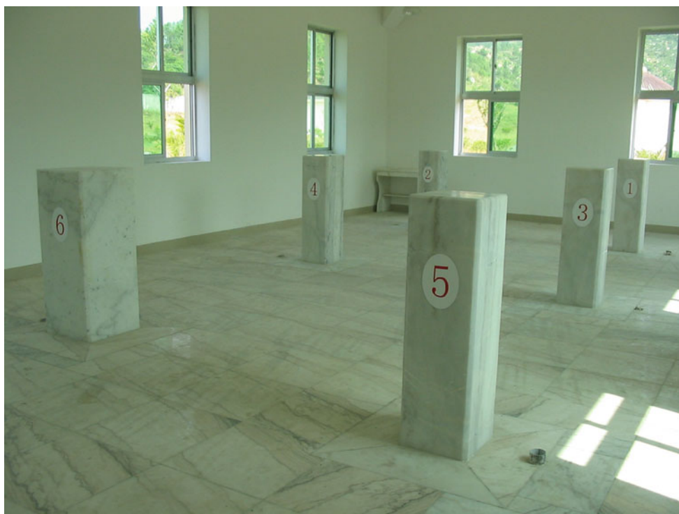
Fig. 1.8 The Quanzhou magnetic observatory absolute house featuring the pillars for the absolute measurement of the geomagnetic vector
