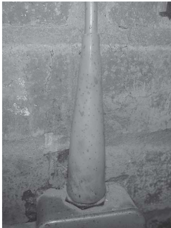
Figure 3.20 A PVC shroud after 30 years service without direct exposure to sunlight
