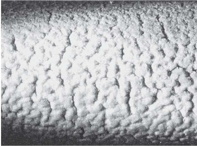
(c) Severe surface degradation
