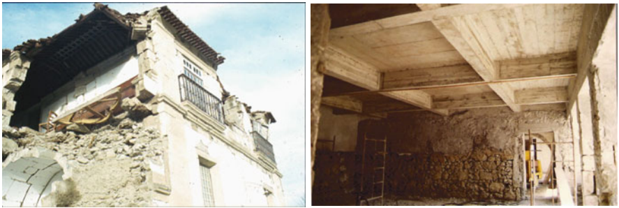
Fig. 9.4 Açores 1980 earthquake: damage to the monumental structures and reconstruction with reinforced concrete
