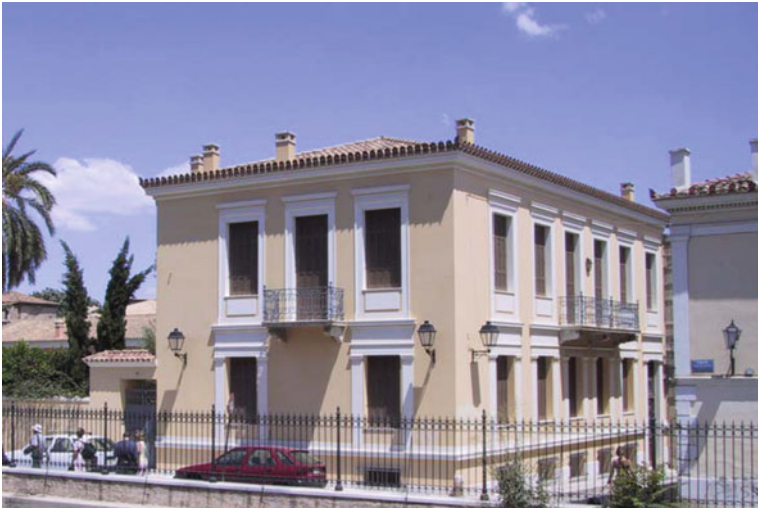
Fig. 1.7 A “neoclassical” building in Athens (19th cent), a monument of local importance
