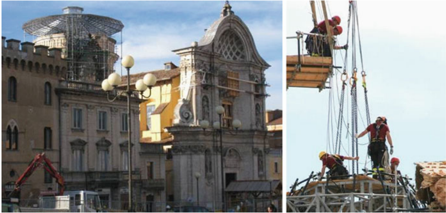
Fig. 20.5 Drum of the Anime Sante's church in the historical centre of L'Aquila ( left ); special groups of National Fire Brigade men at work on the Anime Sante's dome ( right )
