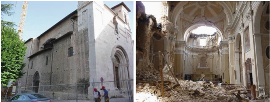
Fig. 20.10 St. Mark church in L'Aquila: external ( left ) and internal ( right ) views
