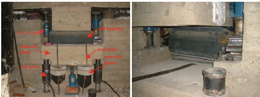
Fig. 17.24 Placement of the hydraulic presses and removal of the central bearing
