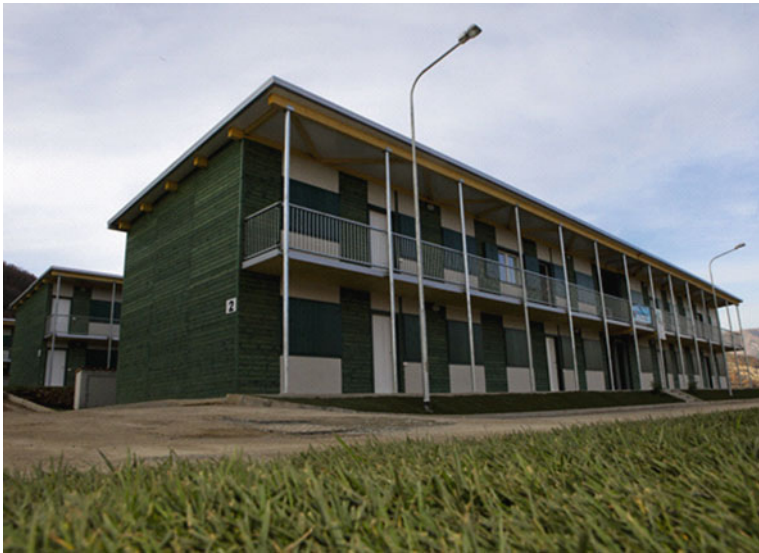
Fig. 19.17 Two-story multimodule M.A.P. inside L' Aquila municipality
