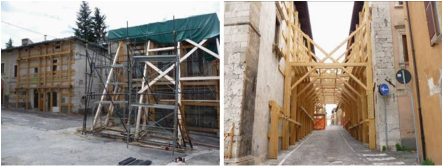
Fig. 20.9 Three types of safety measures on façades in the historic centre of L'Aquila: wooden grids and ties, traditional props, shoring systems acting on facing buildings
