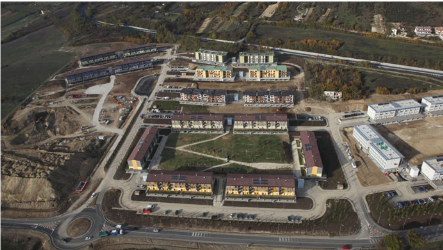
Fig. 19.13 Aerial view of one settlement of the Project C.A.S.E. (Bazzano) on October 29, 2009. Twenty-one buildings are all completed and inhabited by about 1,600 people
