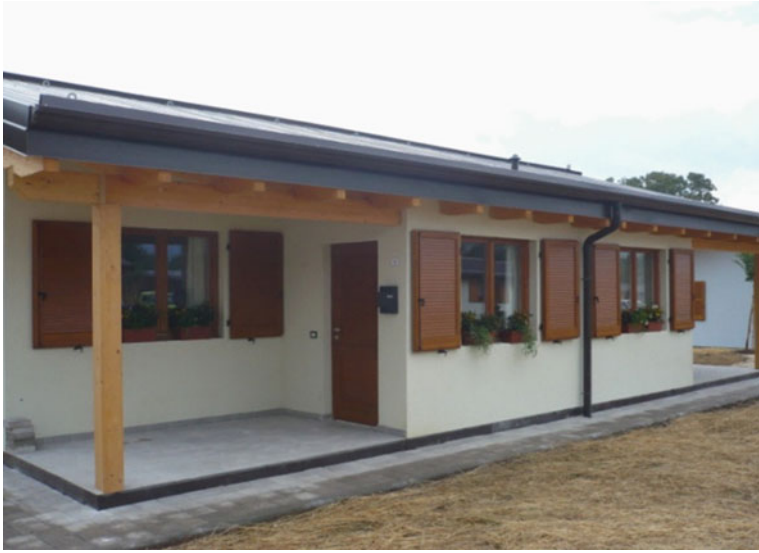
Fig. 19.16 One-story single-module M.A.P. out of L' Aquila
