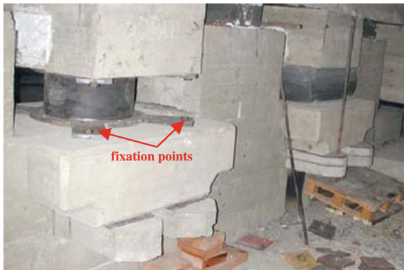
Fig. 17.25 Installed new and old bearing
