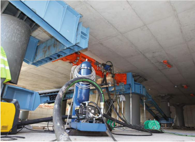
Fig. 19.15 Test set-up for the on-site experimental check
