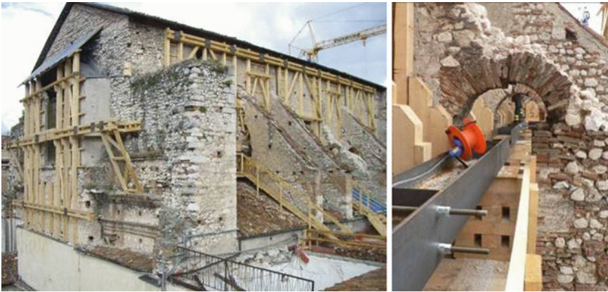
Fig. 20.7 Intervention on Santa Margherita's church in the historical centre of L'Aquila
