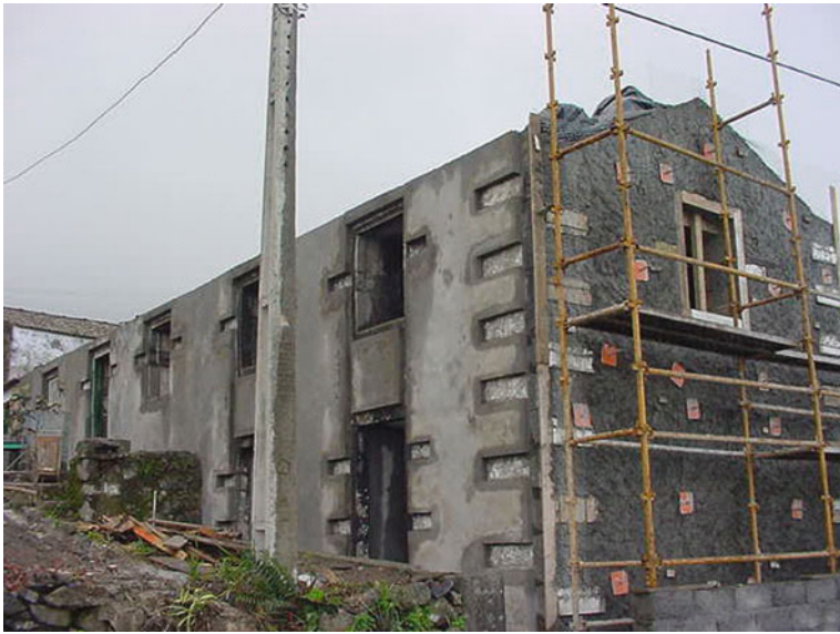
Fig. 9.2 Wire mesh in plaster covering
