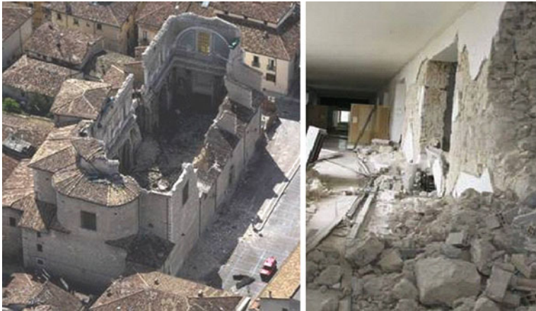
Fig. 19.12 The partial collapses of S. Maria di Paganica and of the Abruzzi Museum in L'Aquila
