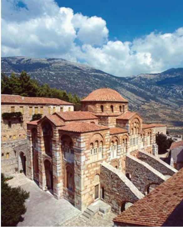
Fig. 1.4 The Hosios Loukas monastery 11th cent. Church (Greece), strengthened by means of external buttresses (11th cent)
