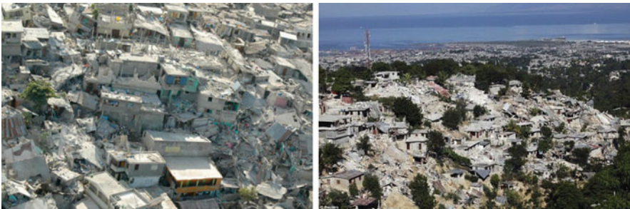
Fig. 9.8 Haiti earthquake. Overview of damage caused to buildings (photos: http://www.refinery29.com/pipeline/img/earthquake-haiti.jpg and http://3.bp.blogspot.com/_U54NM9QE5VY/S07Fcu30qDI/AAAAAAAAAJY4/p06ii_gUrbl/s640/haiti+earthquake.jpg )
