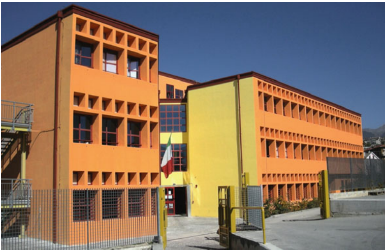
Fig. 19.20 A strengthened school at the start of the scholar year
