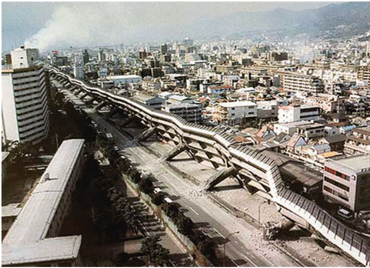
Fig. 10.9 Collapse of the Hnshin Expressway, Kobe earthquake, 1995
