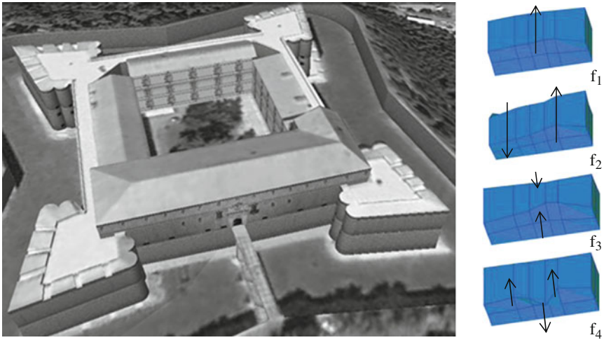
Fig. 20.19 Mode shapes emerged from the dynamic data acquisition
