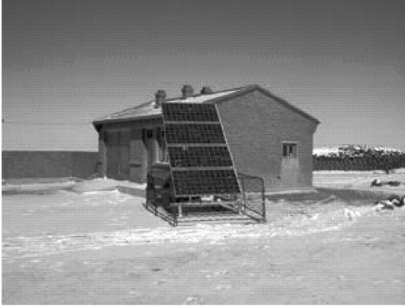
Figure 4. Solar powered house in winter.
