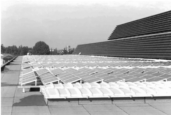
Figure 3. Bologna Airport 80KWp.
