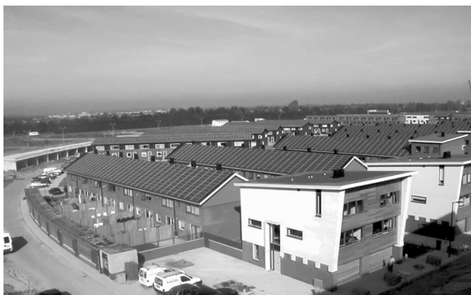
Figure 4. Example of Roof mounted PV suburb at Vroonermee-Zuid.
