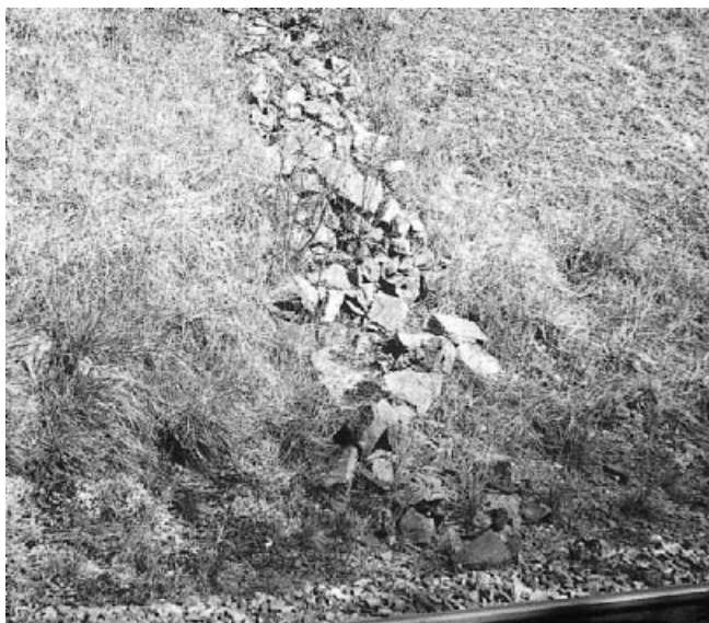
Fig. 6.2. Counterforts and Herring-bone drainage.
