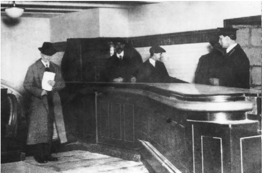
Fig. 12.1. An early underground escalator.
