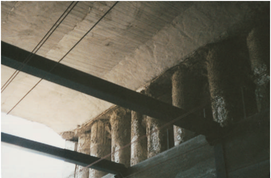
Fig. 8.3. Bored piles used as cut-and-cover tunnel support.
