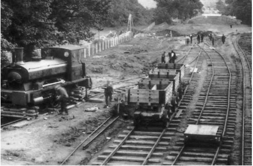
Fig. 1.1. Early railway construction.
