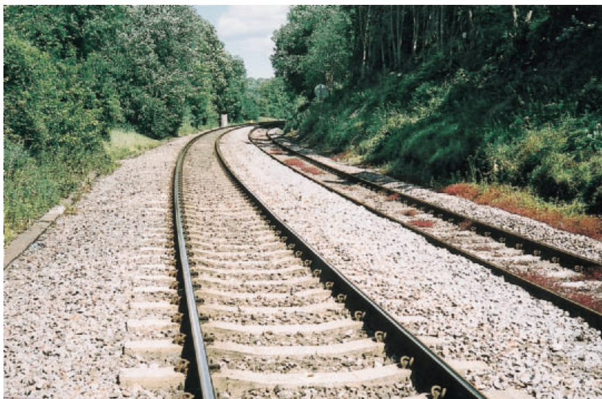
Fig. 5.7. Continuous welded track.
