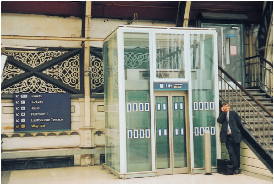
Fig. 12.4. Hydraulic lift for passengers at footbridge.
