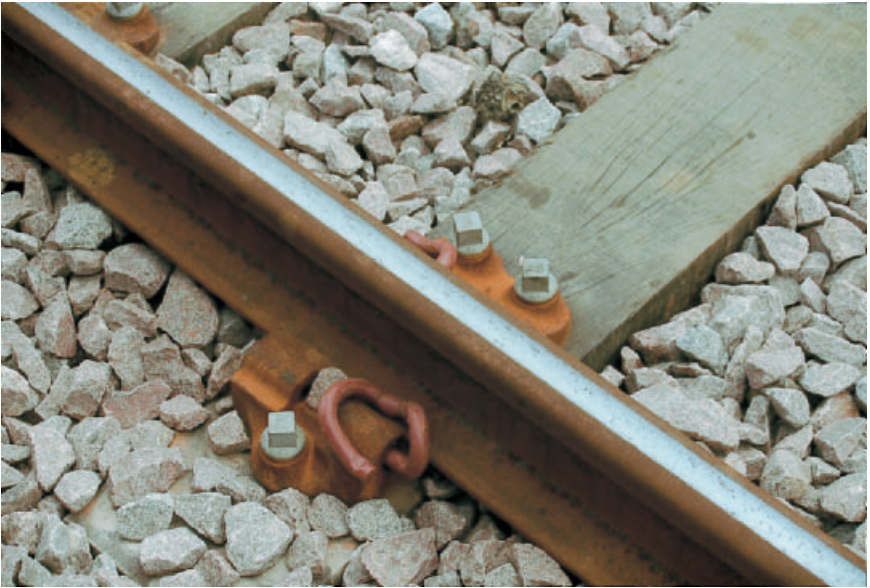
Fig. 5.6. The Pandrol clip and baseplate on timber sleeper (photo by Paul Walker).
