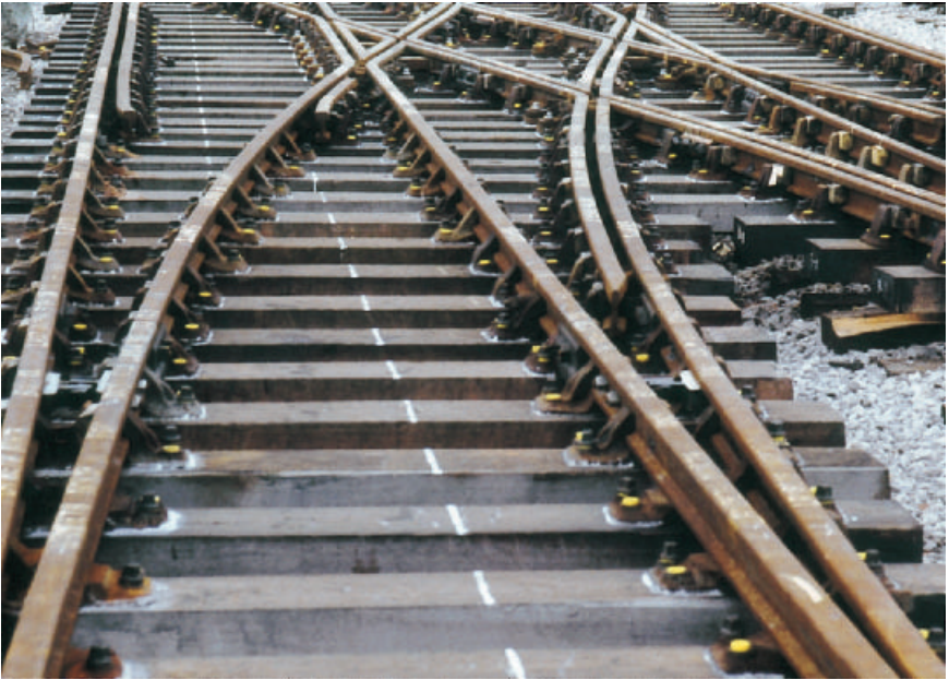
Fig. 5.8. A crossover layout in BH rail.
