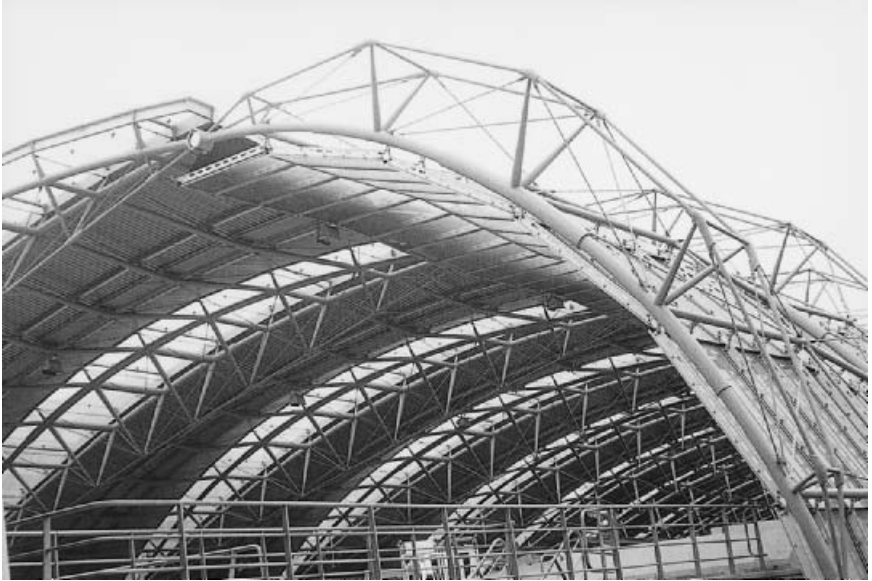
Fig. 7.6. Welded tubular station roof at Waterloo.
