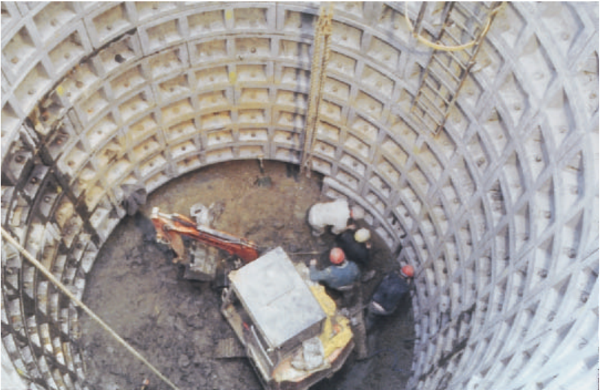
Fig. 8.4. Concrete lined vertical shaft.
