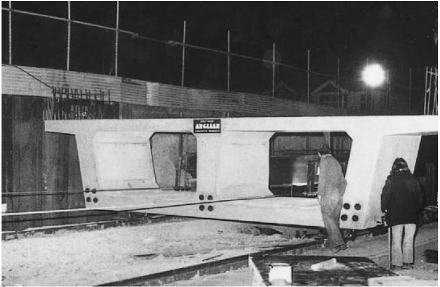
Fig. 7.8. Concrete segmental box girder units.
