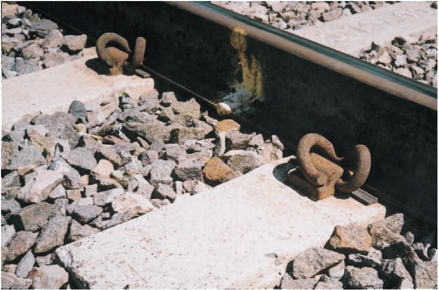
Fig. 5.4. Prestressed concrete sleepers, fastenings and rail weld.
