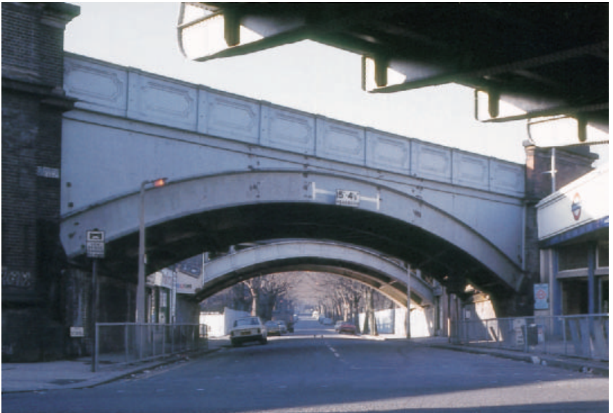
Fig. 7.2. Hundred year old cast iron arches at Kilburn.
