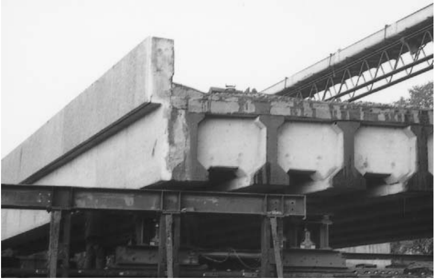
Fig. 7.7. Railway bridge reconstructed using pretensioned prestressed concrete beams.
