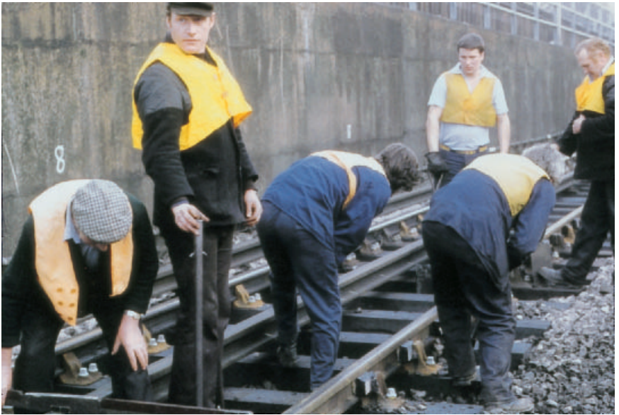
Fig. 5.11. Daytime track maintenance gang at work.
