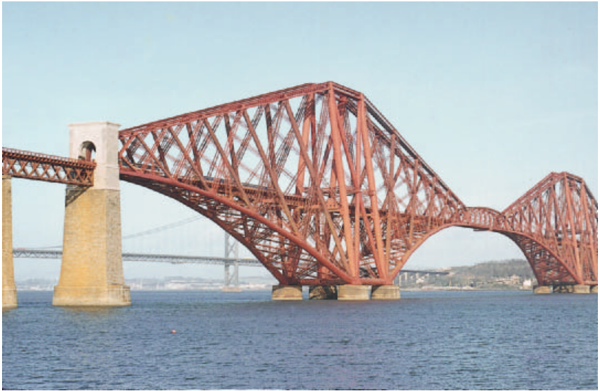
Fig. 7.3. Forth railway bridge — early rivetted steel (photo by Paul Walker).
