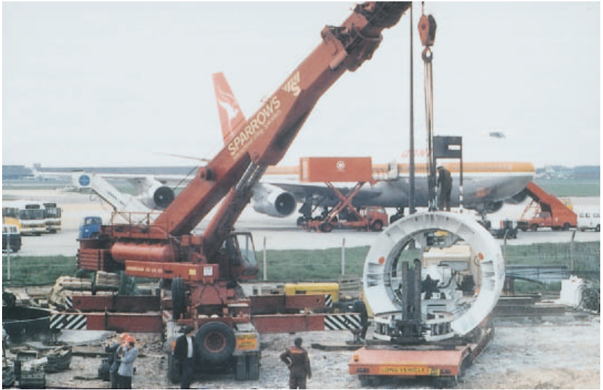
Fig. 8.2. Modern soft ground tunnel shield.
