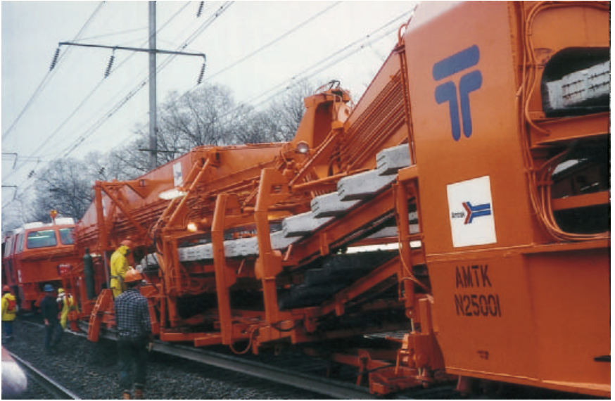
Fig. 5.10. Mechanised track laying.
