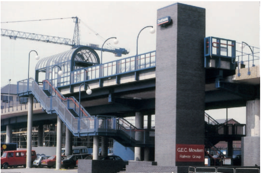
Fig. 2.8. Lift for the disabled, Docklands Light Railway.
