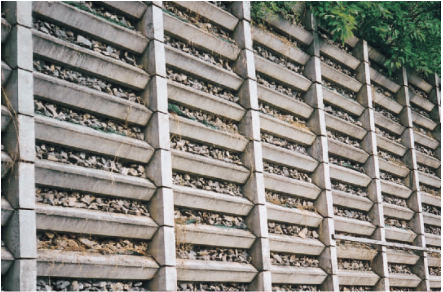
Fig. 6.4. Precast concrete units forming 'crib' retaining wall.
