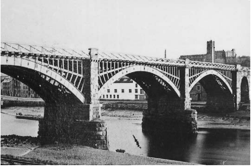
Fig. 7.1. Laminated timber arched bridge at Lancaster.
