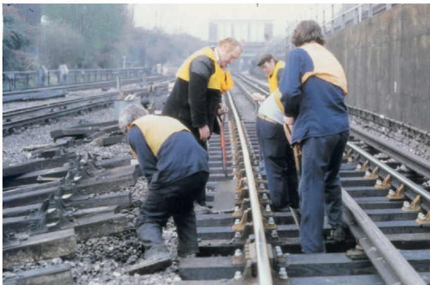
Fig. 5.3. Individual renewal of timber sleepers.
