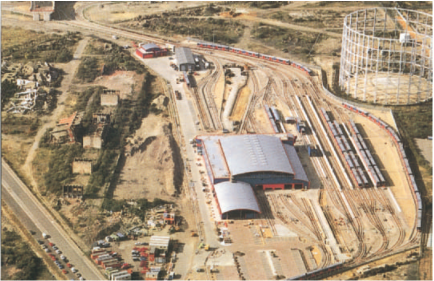
Fig. 4.3. Light rail depot.
