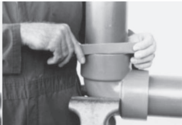
Remove excess cement residue at pipe joint and make sure the joining is moisture-free.
