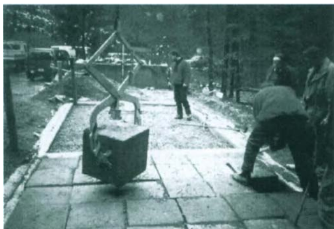
Fig. 1: The investigated field lysimeter during dismantling in December 1997
