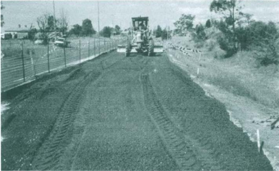
Figure 1. Field trial using low RAP/crushed concrete blends, a very homogeneous material with no signs of segregation.
