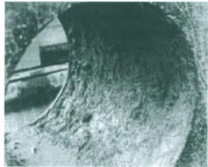
Figure 11. Sisal fiber distribution at the inner surface of the spun pipe
