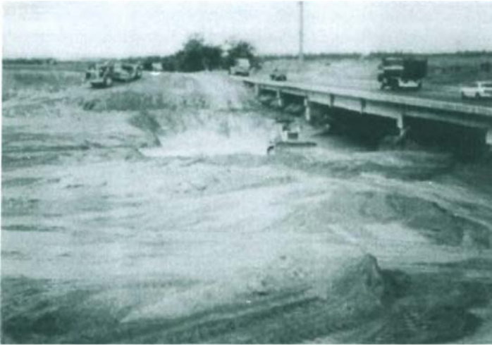
Figure 3 Pampanga sampling site in 1996, showing the extent of volcanic debris deposited under a bridge with former clearance height of 24 meters.
