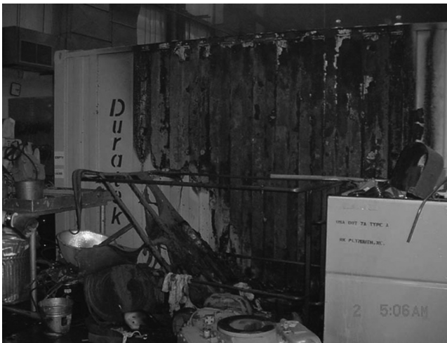
Figure 6.1 Fire-damaged area in multipurpose facility.
