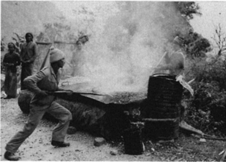
**Figure 19.4** Hand-mixing hot asphalt in India.
