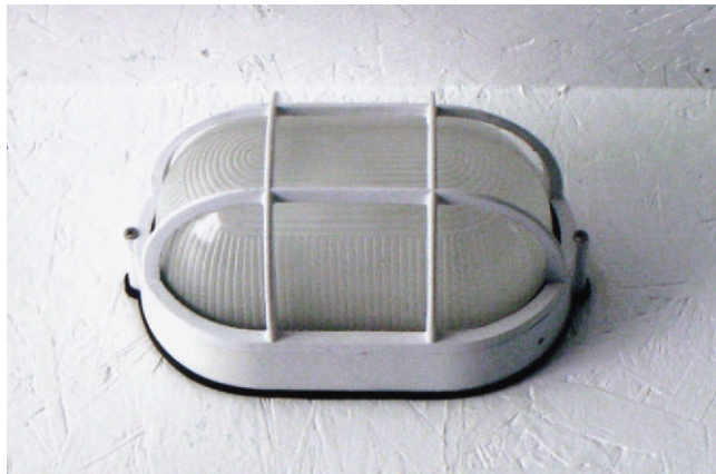
FIGURE 19-2 Waterproof, caged light fixtures that use incandescent lamps are best.
