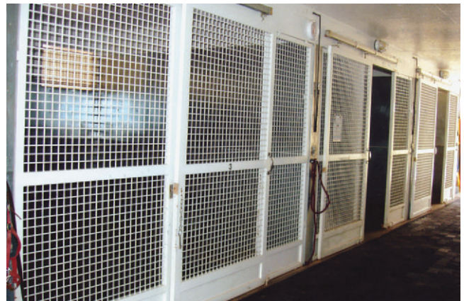
FIGURE 19-6 Full-length, heavy-duty mesh stall fronts allow an unobstructed view of the whole horse, including its feet.
