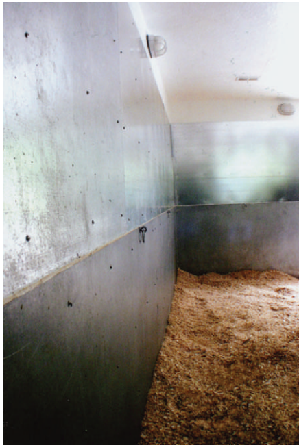
FIGURE 19-1 This stall wall is easy to disinfect, maintenance free, and safe for the horse.
