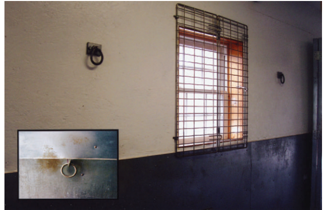
FIGURE 19-3 Anchor rings in the stall wall can be used to assist a recumbent horse to stand.
