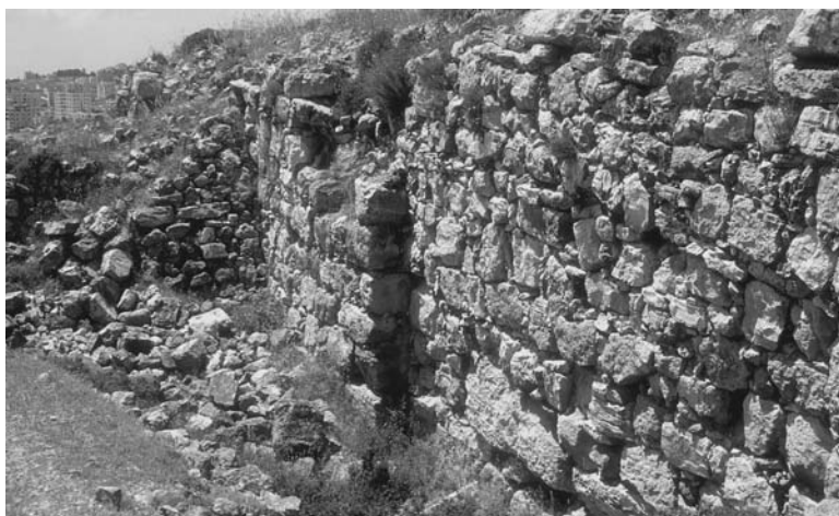
Figure 62 Mizpah, offset-inset wall.
