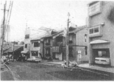
Photo 9 Houses with light roofs that survived in a severely damaged area
