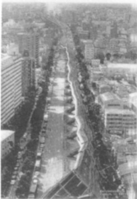
Photo 3 Cantilevered columns of the Hanshin Highway at Ashiya City
