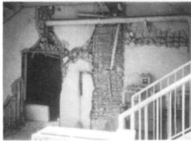
Photo 15 Building designed under new Code was not severely damaged
