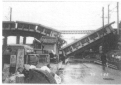
Photo 2 Damage to the Sanyo Shinkansen Railway near Nishinomiya
