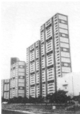
Photo 17 High rise steel apartment building damaged
