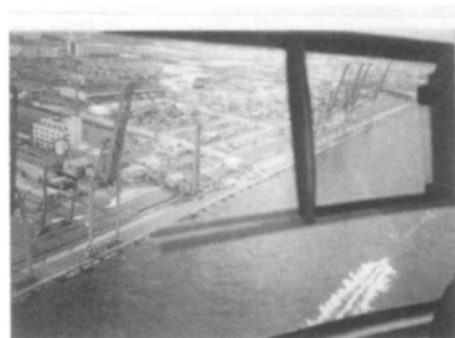
Photo 6 Damage caused by liquefaction on Port Island
