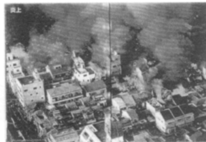
Photo 12 More than 7,000 houses were destroyed by fire
