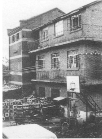
Fig. 2. Tangshan, China, 1976: survived building.
