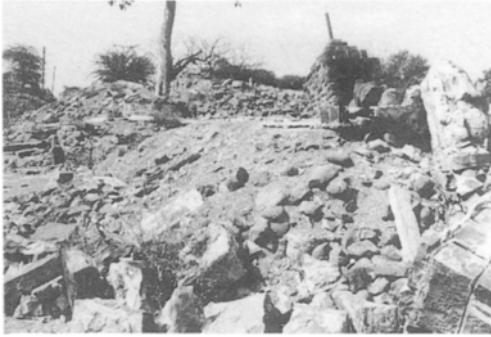
Fig. 1. Killari, India, 1993: completely destroyed village.
