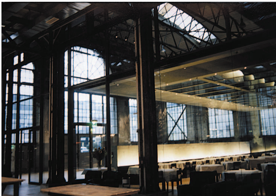
A ceiling suspended from the main structure defines the restaurant area. The inherited character of the building remains. Photo: Harold Lutz.
