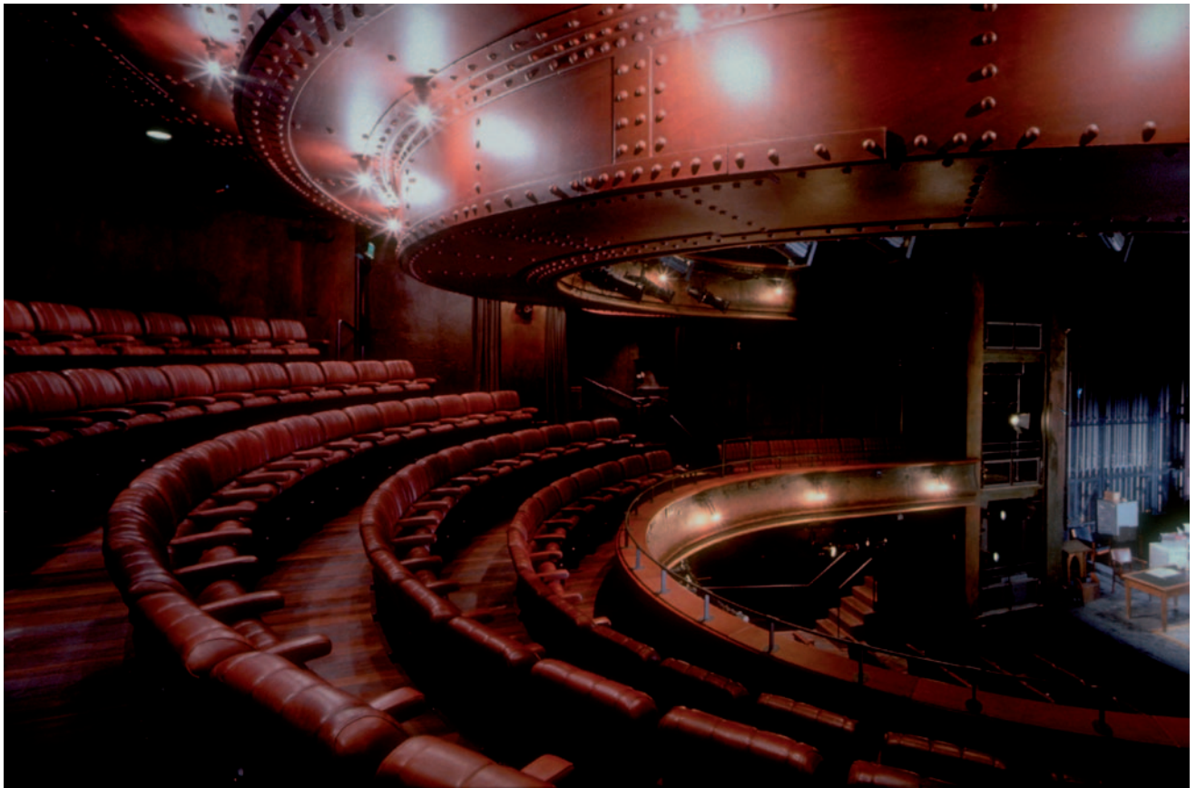
View from the main auditorium: functional expression as interior decoration. The proscenium opening is 'softened' to lessen the division between stage and auditorium: the zone accommodates the performance lighting and sound speakers.
