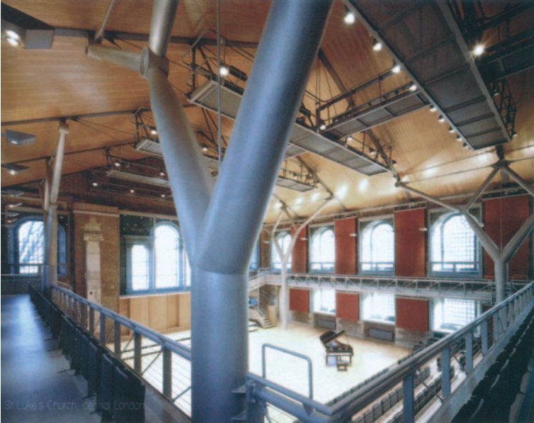
Figure 9.4 St Luke's, London A redundant church converted for rehearsals by a leading professional orchestra, with occasional public performances. An example of a close fit between existing building and new use. This re-use of an existing building also incorporates natural ventilation (using the spire as a stack and exhaust chimney, while the heating is assisted by geo-thermal bore-holes through the floor of the existing building. (Architects: Levitt Bernstein).
