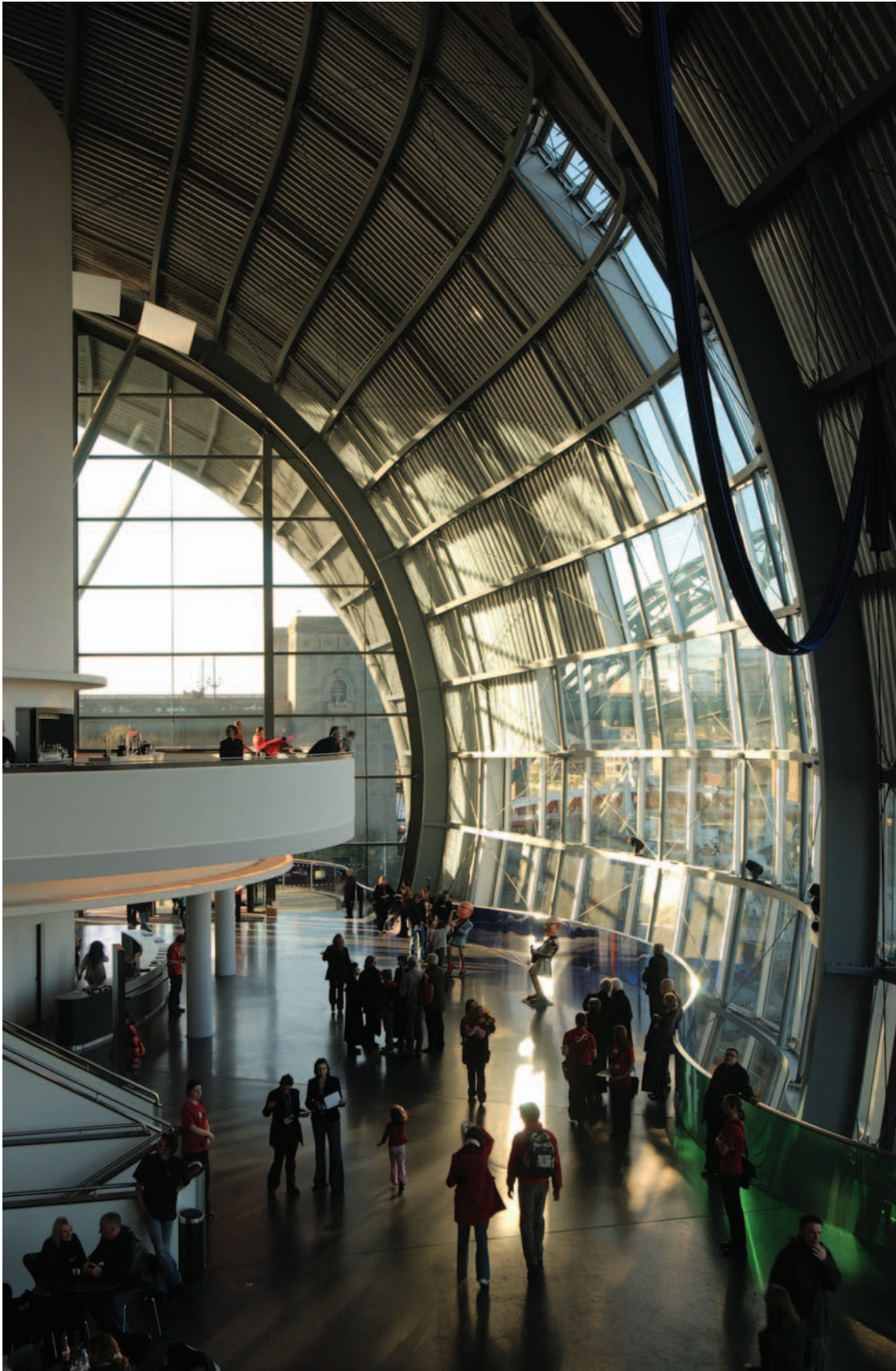
The concourse: a large circulation and gathering space, overlooking the river which links the three performance spaces. The undulating curved external enclosure sits independent of all internal enclosures.
