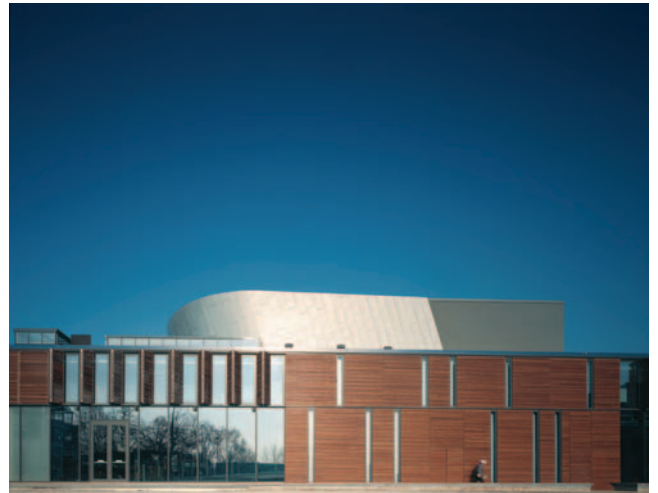
External view of theatre from the new landscaped open space. The façade consists of panels of glazing and timber screens. The slots are for Martin Rickman's light sculptures. Photo: Peter Cook.
