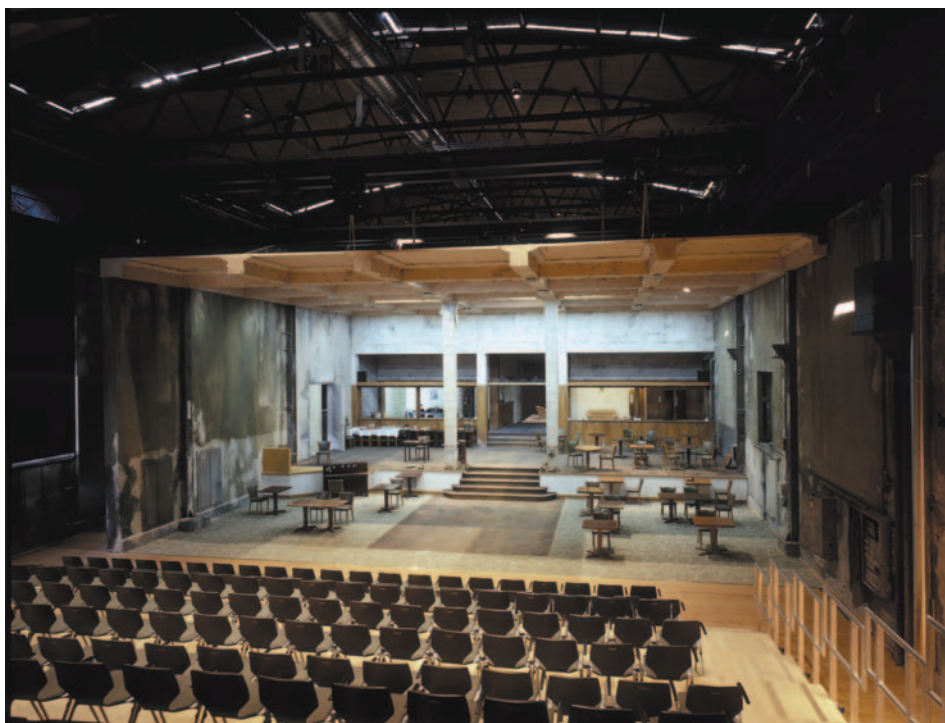
Theatre: a free-standing structure for the seating, with a canopy over the stage as part of the scenery suspended from the existing structure. Photo: Margherita Spiluttini.
