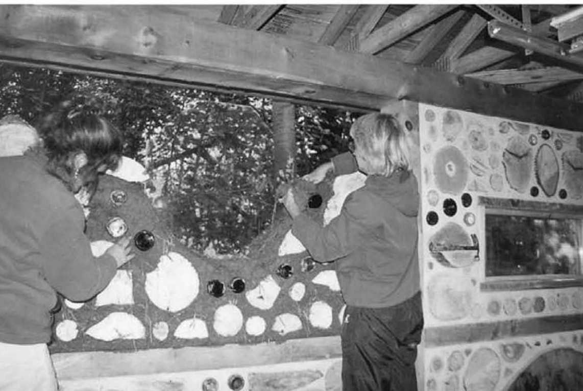
20.1: Linda Smiley (left) and Jaki Roy lay up cob in preparation for log-ends. Note that rubber gloves are not necessary for playing with “mud pies.” Panel at right is cordwood with mortar.
