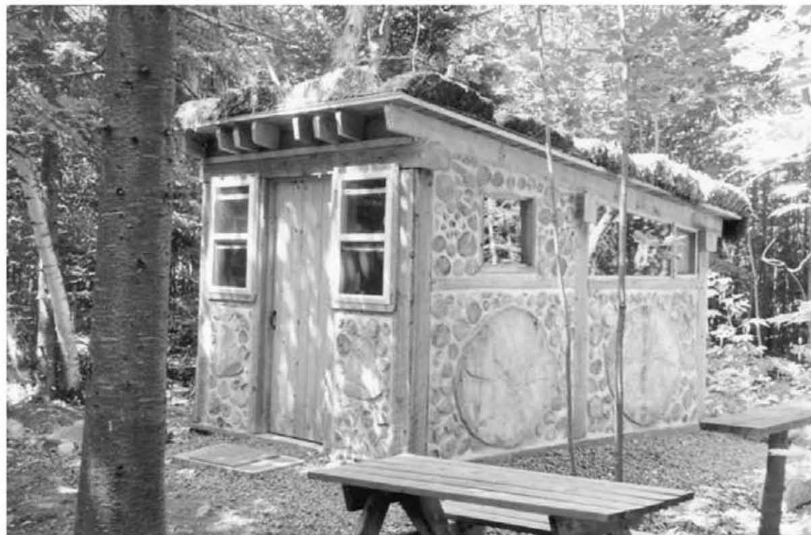
26.2: La Casita , a guesthouse at Earthwood, would make a good TS for a single person, while providing a lesson in simple post and beam framing.
