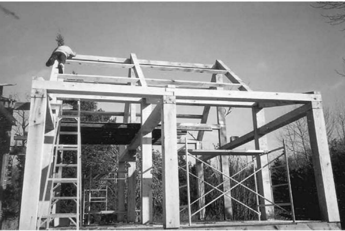
25.1: Our post and beam frame.
