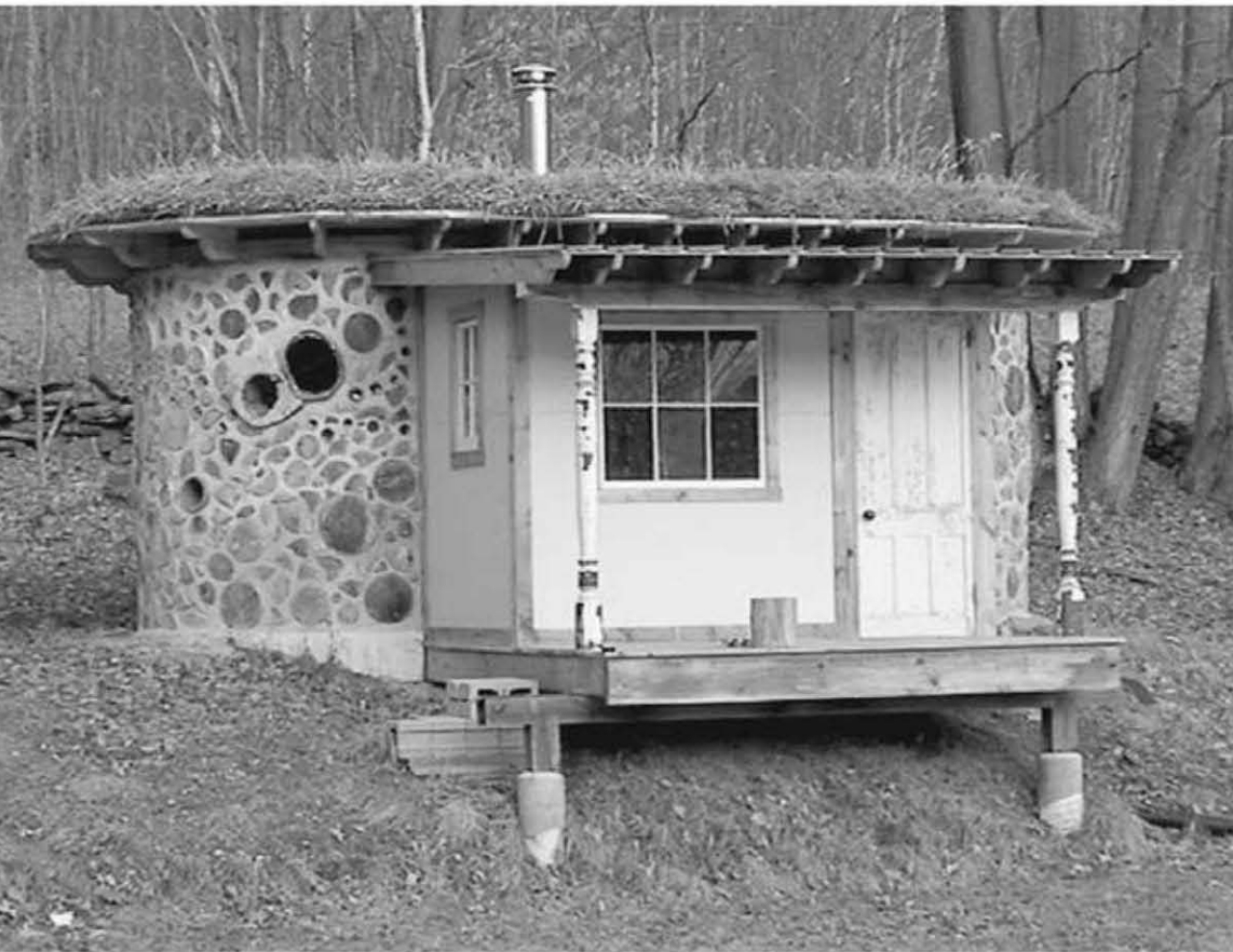
24.3: The new Pompanuck Community sauna. Note the ventanas naturales on the left, inspired by Hans Hebel of Chile. Credit: John Carlson.
