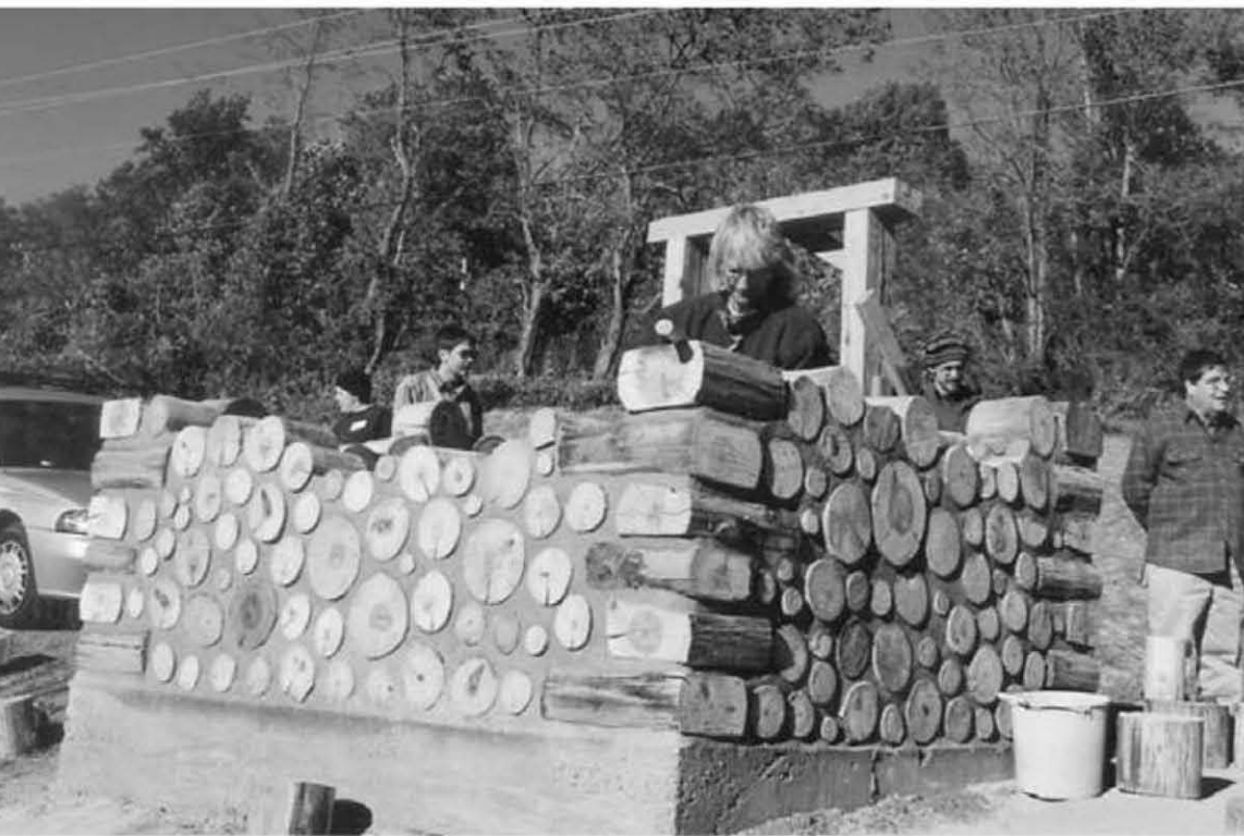
2.6: A cordwood masonry workshop conducted by Rob and Jaki Roy near Bakersville, North Carolina.
