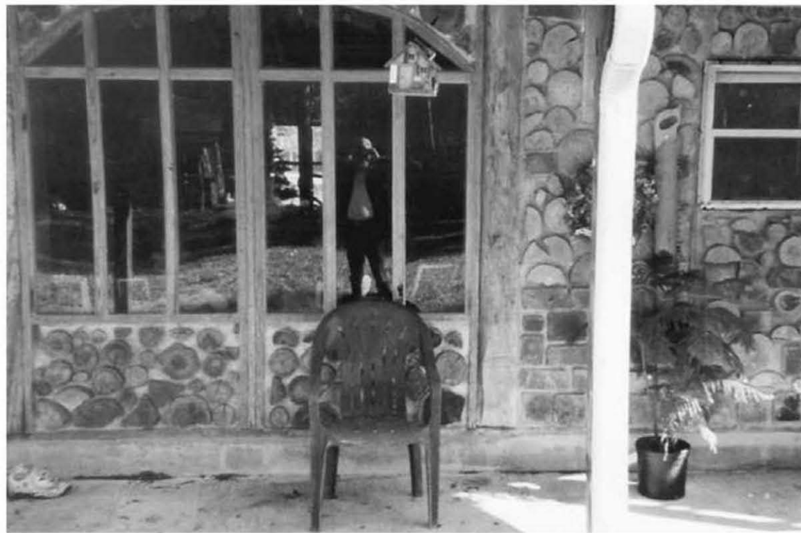
18.1: Part of our large “Texas porch.”
