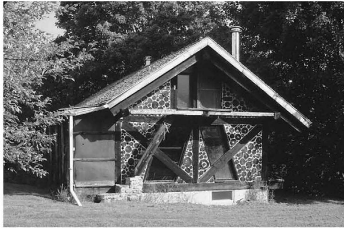
2.1: Log End Cottage, the author's first cordwood home, built in 1975–76 in West Chazy, New York.
