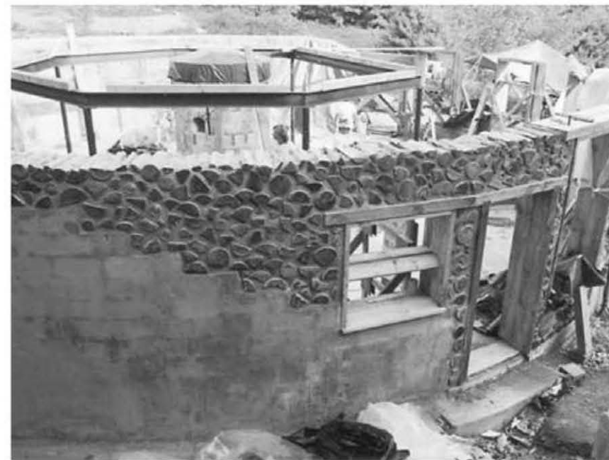
24.2: Lower storey construction of Pompanuck Round House, Cambridge, New York.
