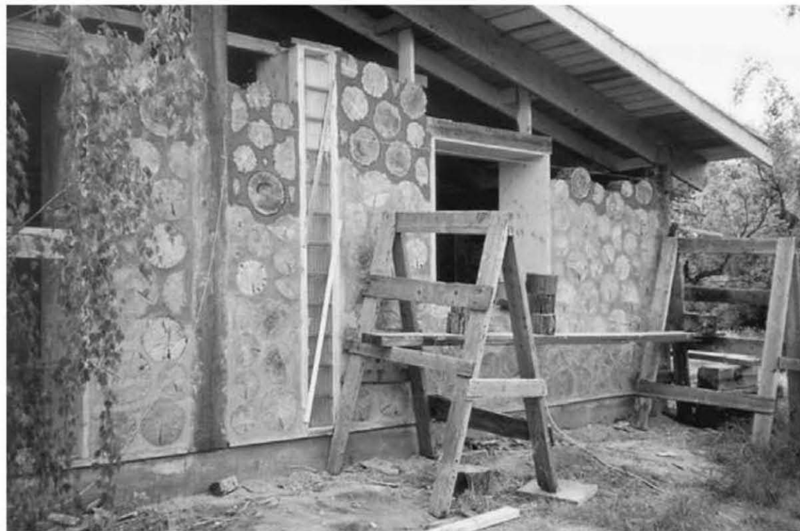
4.5: Cliff's addition, shown under construction, was built in 1990. Credit: Cliff Shockey.
