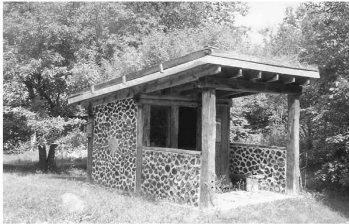
2.3: Log End Sauna, built by the Roys in 1979, is still used as a sauna today.
