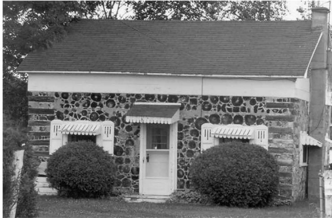
1.2: This stackwall cornered cottage is located on the Rideau River, County Road #19, outside of Kemptville, Ontario. The photographer was told that it is between 100 and 120 years old.
