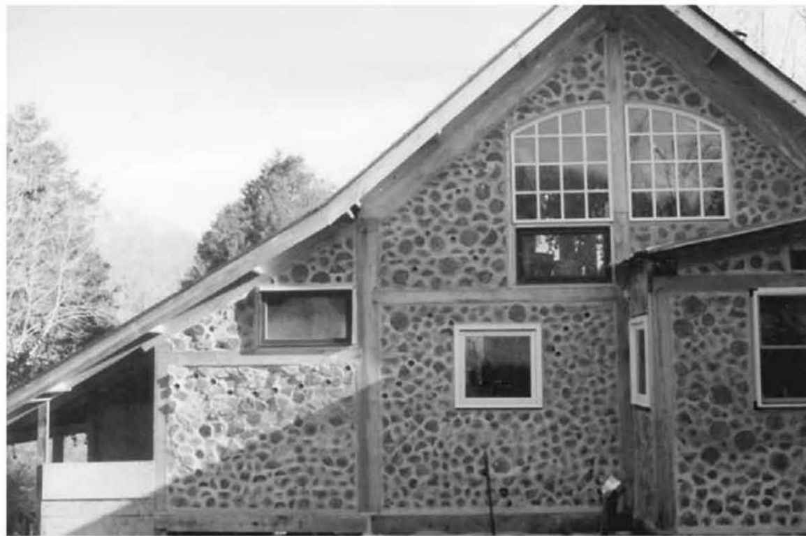
25.2: Our 9-inch-thick (23-centimeter-thick) red cedar cordwood walls fill all the panels framed by the posts and beams.
