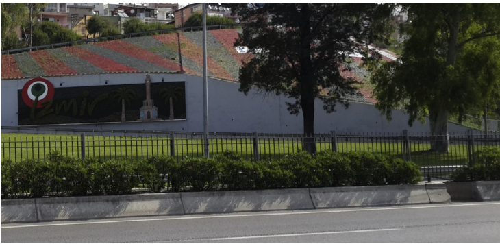
Figure 11.2 Greenwall as an urban element near a road depicting the famous clock tower at the city of Izmir-Turkiye. Courtesy of author.
