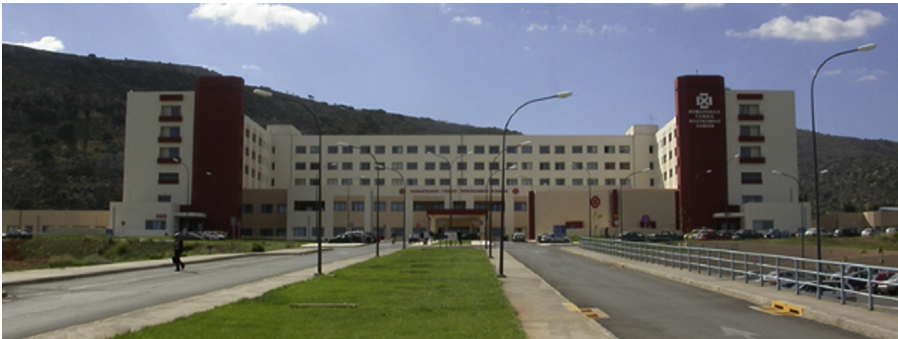
Figure 15.2 General hospital Chania Saint George, in Greece.
