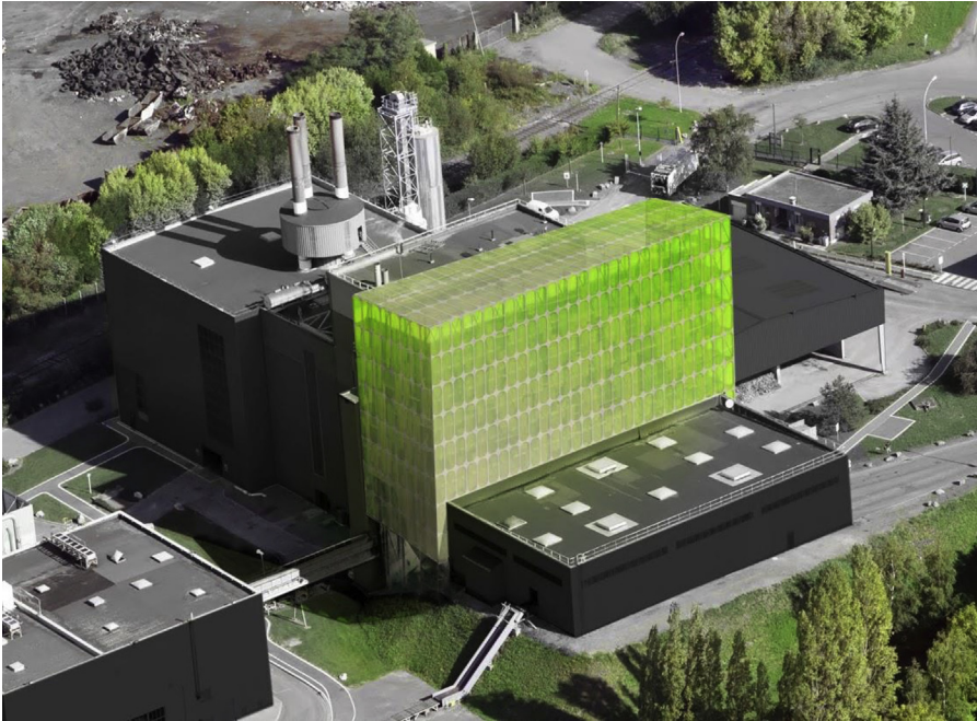
Figure 11.20 Concept of an industrial symbiosis between a waste incineration plant and microalgae biofaçades, using CO 2 and energy from the plant for microalgae cultivation. Courtesy of Olivier Scheffer, XTU Architects.
