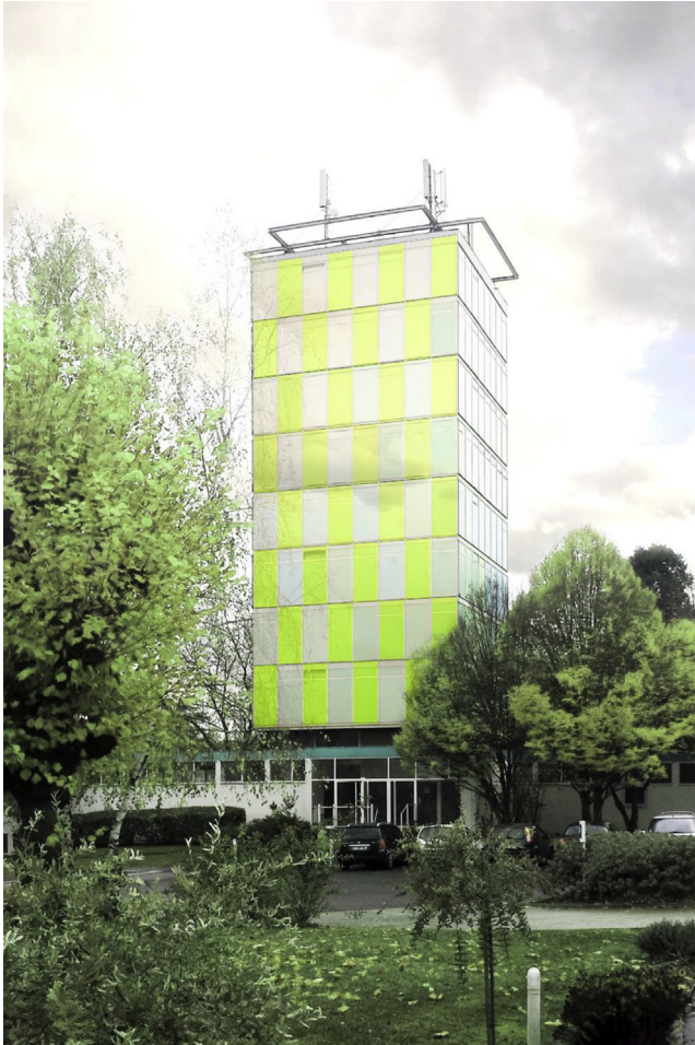
Figure 11.23 Pilot project for the first 200 m 2 biofaçade equipped with curtain-wall integrated PBRs, CSTB Headquarters, Champs-sur-Marne, France. Courtesy of Olivier Scheffer, XTU Architects/SymbIO2.
