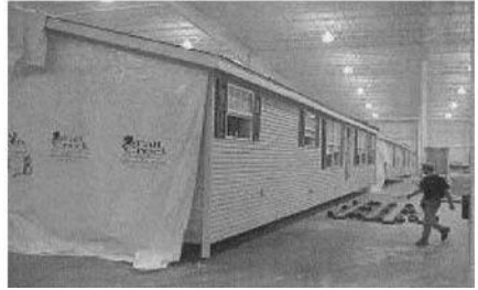
Picture (4): Finished Floor
