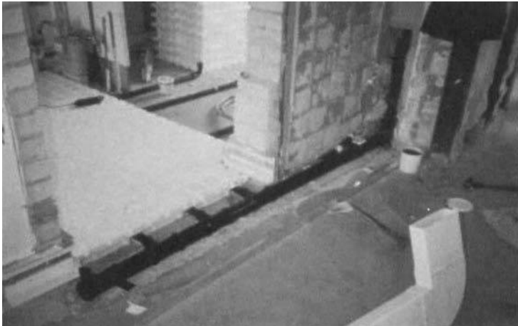
figure 8: Matura lower system during installation w/0-slope drainage piping in Matrix tile
