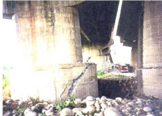
Fig. 8-4: Wushi Bridge - settlement and shear cracks at pier P3N
