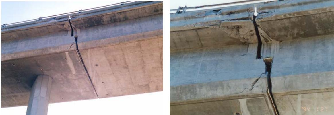
*Fig. 11-61: Damage of intermediate joint due to pounding (1994 Northridge earthquake)
