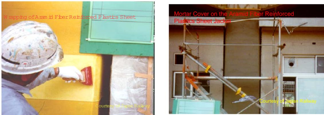
Fig. 11-30: Aramid fiber reinforced plastics jacketing for a railway viaduct [courtesy of JR Research Institute] (Figure available electronically on *fib* website; see production note on p. ii)
