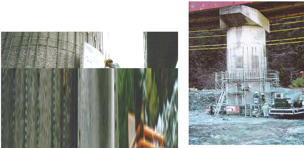
Fig. 11-35: Precast concrete segment jacket [courtesy of PS Concrete]
