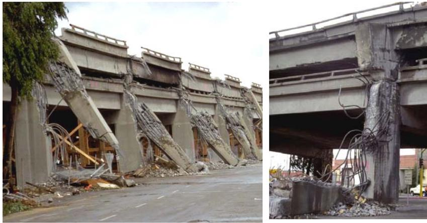
Fig. 10-8: Sliding shear at top columns of the Cypress viaduct in the 1989 Loma Prieta earthquake (after NISEE, 2000). (Figure available electronically on fib website; see production note on p. ii)
