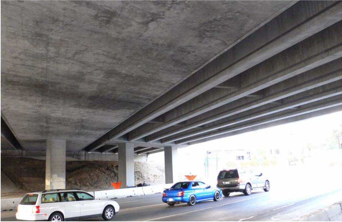
Fig. 4-10: Example of use of the use of precast I-girders on a highway bridge widening project in California (Courtesy of J. Restrepo)
