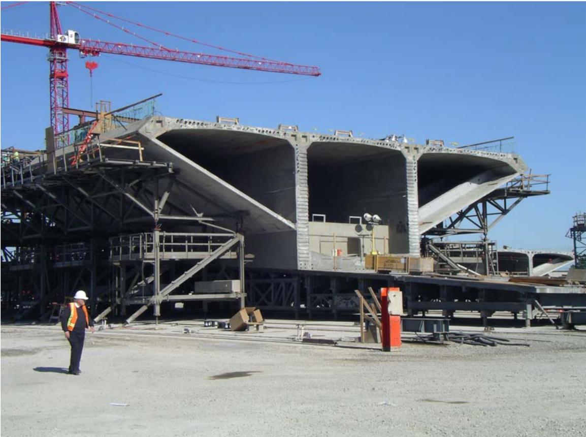
*Fig. 4-9: Precast segmental elements for the construction of the San Francisco-Oakland Bay Bridge Skyway Structure (Courtesy of F. Seible)
