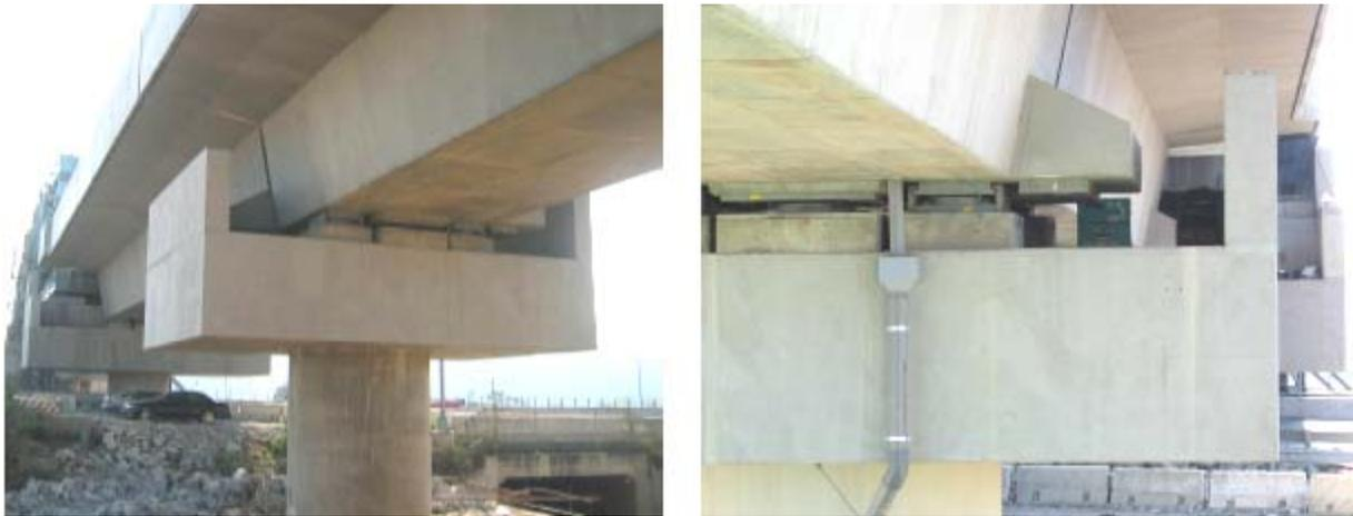
*Fig. 8-16: Piers with extended seating length and special bearings
