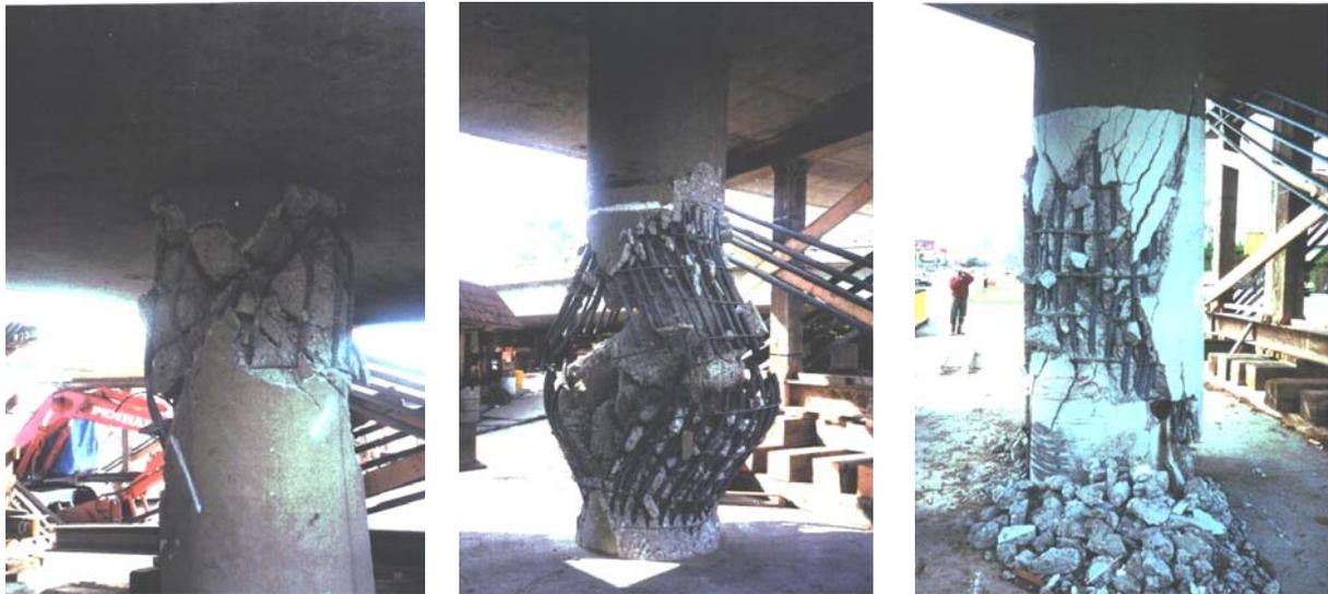
*Fig. 10-7: Different shear damage patterns for RC piers at the under-crossing of the Santa-Monica Interstate 10 during the 1994 Northridge earthquake: Piers # 5 with inadequate detailing for plastic hinge (left), Piers # 6 with symmetric buckling (middle) and Pier # 8 with typical shear failure (right) (after Broderick *et al.*, 1994). (Figure available electronically on **fib** website; see production note on p. ii)*
