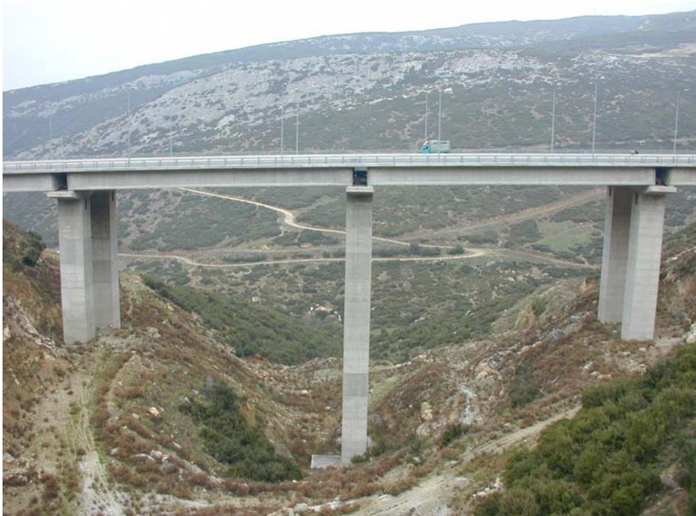
*Fig. 4-7: The G2 bridge near Kavala (NE Greece); the superstructure consists of precast post-tensioned beams connected through a cast in situ top slab (typical of older construction) (Courtesy of A. Kappos).
