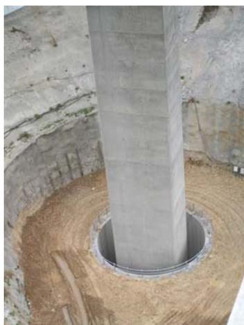
*Fig. 4-12: Use of a 'pre-shaft' to increase the pier length in an Egnatia bridge (Metsovitikos)
