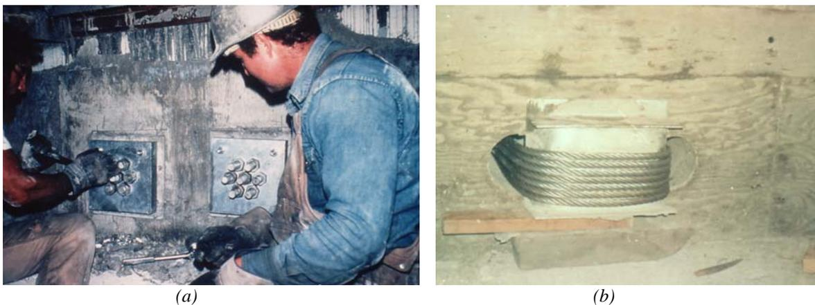
*Fig. 11-62: Installation of cable restrainers (courtesy of California Department of Transportation)
