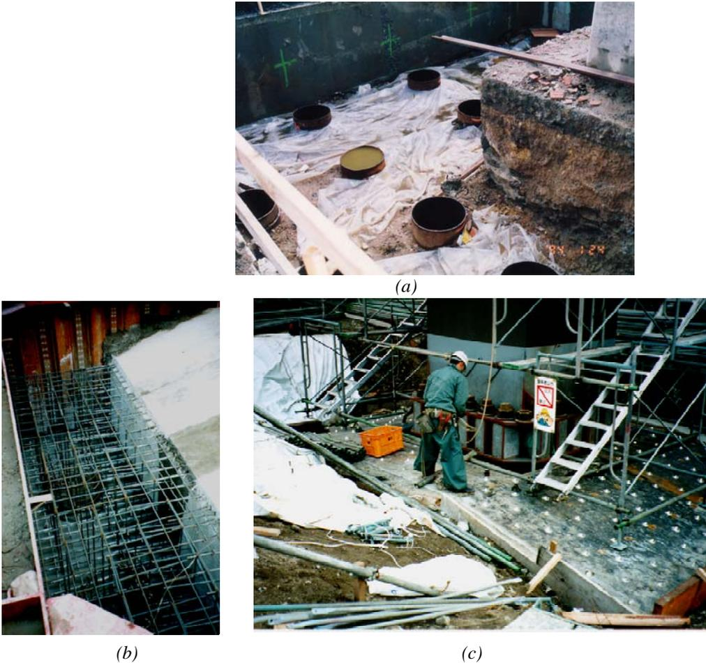
Fig. 11-52: Footing retrofit: (a) extension of footing and new piles (California, USA), (b) extension of footing and new piles (Japan), and (c) Overlay of footing (Japan)
