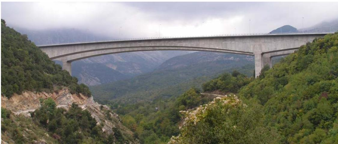
Fig. 4-2: The Votonosi Bridge near Metsovo (NW Greece); the superstructure consists of a post-tensioned single cell box girder (common in modern bridges), and its 230m central span, is the longest span so far in balanced cantilever construction in Greece (Courtesy of A. Kappos).
