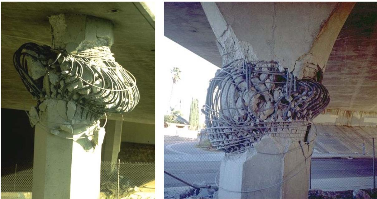
*Fig. 10-4: Confinement failure at bridge pier top during the 1994 Northridge earthquake (after NISEE, 2000).
