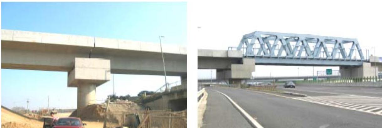
*Fig. 8-17: Steel bridge and in-situ concrete bridges
