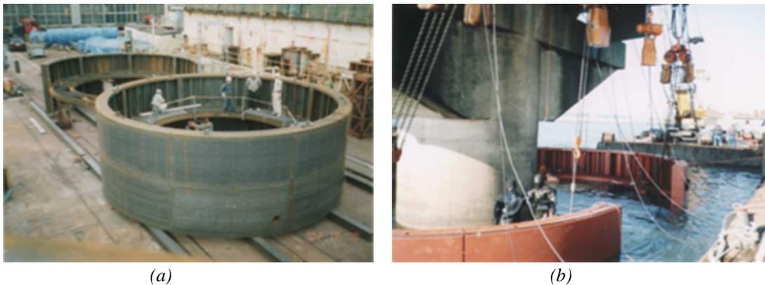
Fig. 11-55: Implementation of steel segment dry-up method: (a) assembling test, and (b) assembling the segments around the foundation [courtesy of Obayashi Construction]
