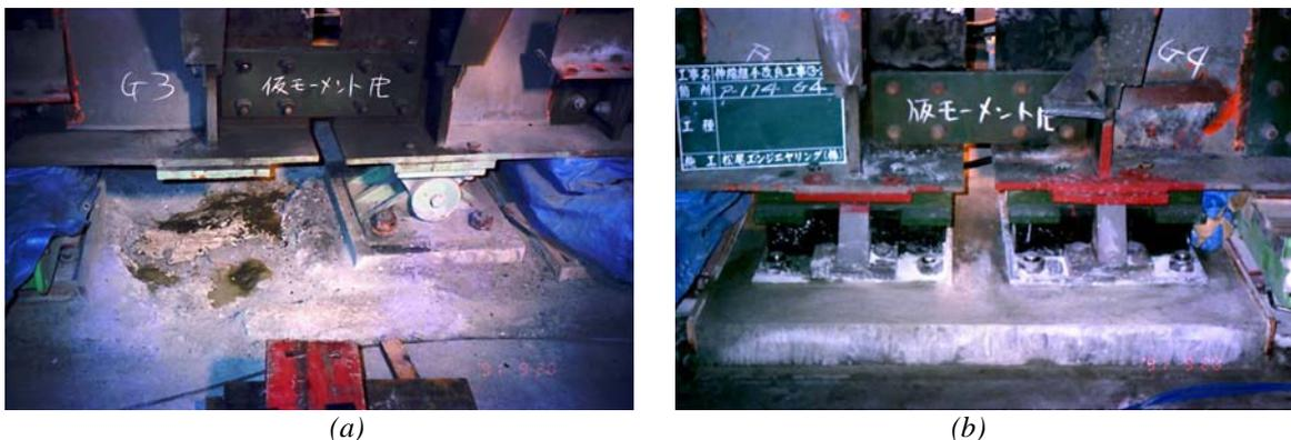
Fig. 11-68: Connection of decks and retrofit: (a) removal of existing steel bearings, and (b) set of new lead rubber bearing (courtesy of Hanshin Expressway Public Corporation)
