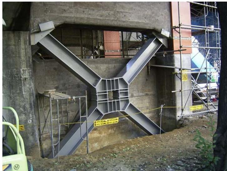
Fig. 11-73 Viaduct retrofitted using compression brace damper [Yoshida et al. (2005)]
