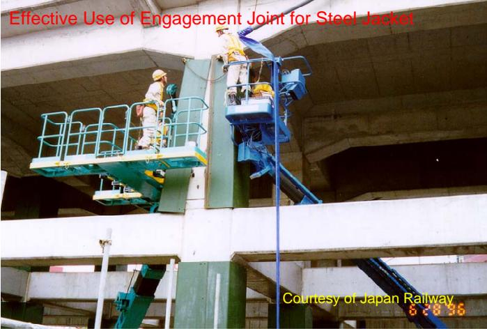
Fig. 11-14: Effective use of engagement joint for retrofit at a railway viaduct (JR Research Institute) (Figure available electronically on fib website; see production note on p. ii)
