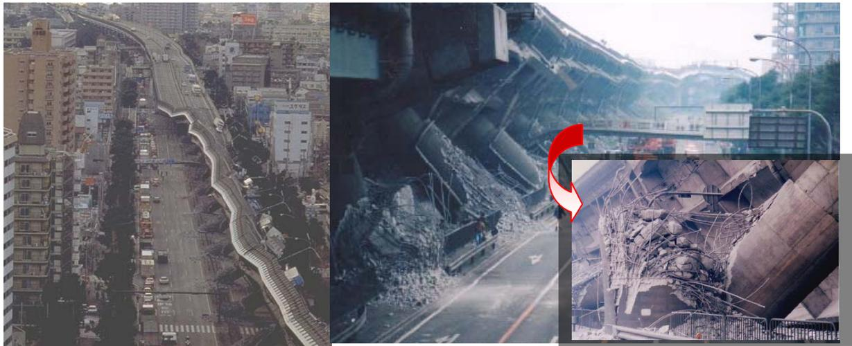
*Fig. 10-5: Flexural failure above column base of columns of the Hanshin expressway, due to premature termination of longitudinal reinforcement and inadequate confinement in the 1995 Kobe earthquake (courtesy of Kawashima). (Figure available electronically on **fib** website; see production note on p. ii)*
