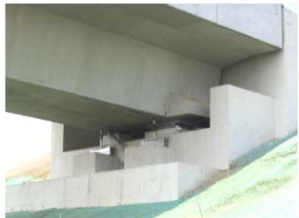
Fig. 8-15: Abutment with extended seating length and special bearings
