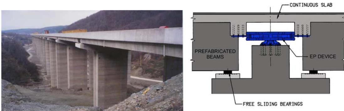
Fig. 6-19: View of the Bolu Viaduct (Priestley and Calvi, 2003) (left) and detail of the pier top (Marioni, ALGA S.p.A.) (right). (Figure available electronically on fib website; see production note on p. ii)
