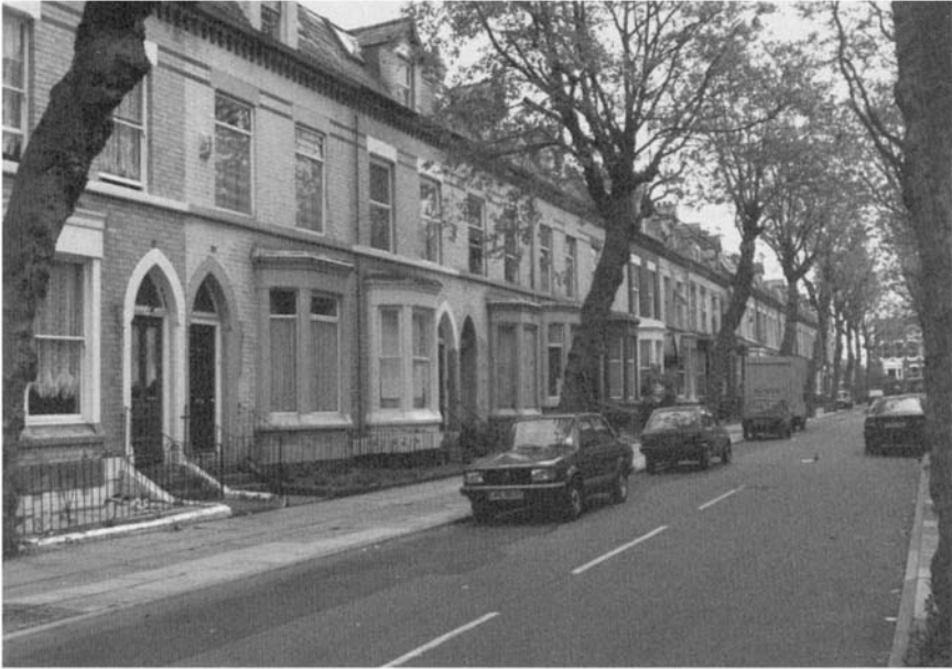
Figure 3.4 Shelter's Neighbourhood Action Project in Toxteth, Liverpool—the first to attempt the rehabilitation of urban housing in partnership with tenants and residents.
