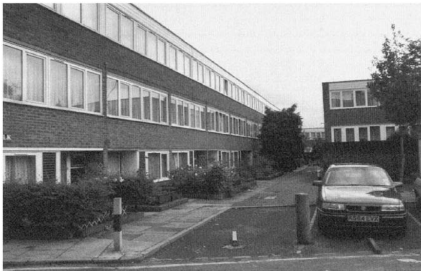
Figure 6.1 Popham Street estate, Islington, as dense as many high-rise developments. It is typical of the more sensitive, but still regimented, approach to council housing in the 1970s.
