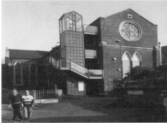
Figure 5.5 The Huddleston Centre in east London—part of a large church divided into several levels as a multipurpose community centre. A project designed and built by collective Building and design.
