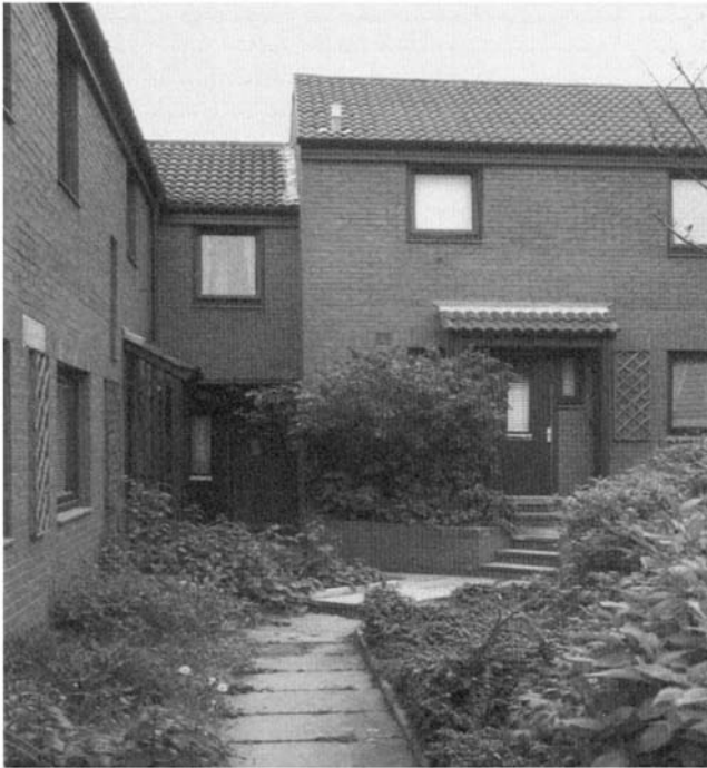
(b, right) The new housing—a simple but attractive traditional design with generous landscaping.
