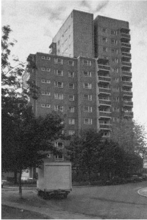
Figure 2.10 West Kentish Town estate, north London, one of the first housing developments built using heavy panel prefabricated systems.
