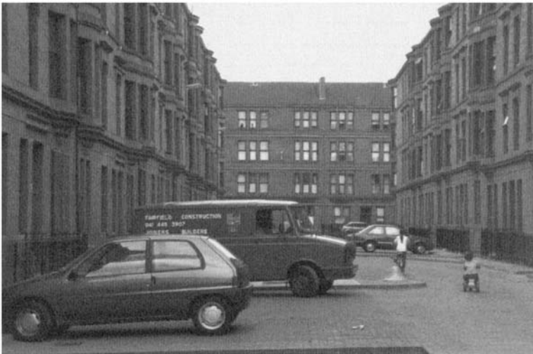
Figure 5.1 (top) Assist's improvements to the Taransey Street tenements. New bathrooms built in and three small flats combined to make two of reasonable size. (foot) 20 years after improvement, a lasting and successful alternative for many Glasgow tenements otherwise scheduled for demolition.
