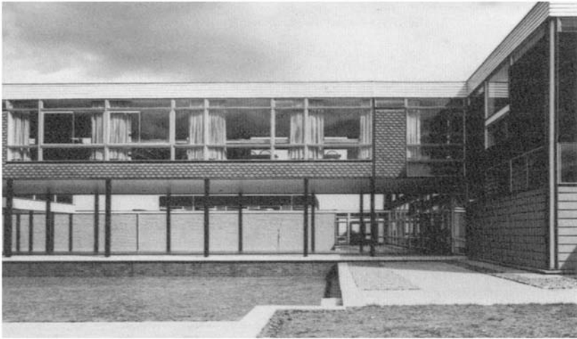
Figure 2.7 West Bridgford Grammar School designed by Nottingham County Architects Department. A typical product of the CLASP system.
