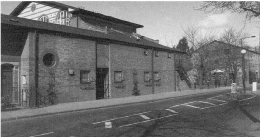
The closed public face of the family houses, with the four-storey block behind and the shared houses to the right.
