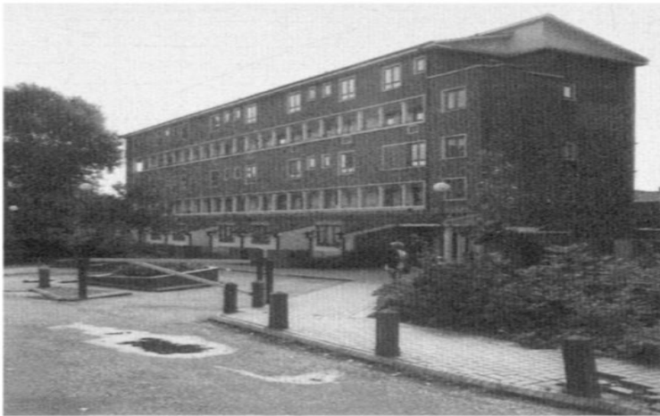
The five-storey block before and after modernization. Improvements included a new roof, improved insulation, new windows and inter-com security to the upper floors.
