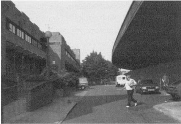
The “barrier” block turns its back on the motorway. Flats are planned so that only utility rooms face the motorway. Living rooms and bedrooms face away. Residents of the block are protected from the noise just as the block itself protects the rest of the site.
