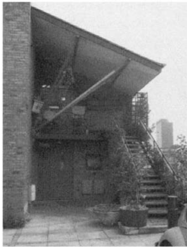
Entrance to the single person flats at the side of the four-storey block.
