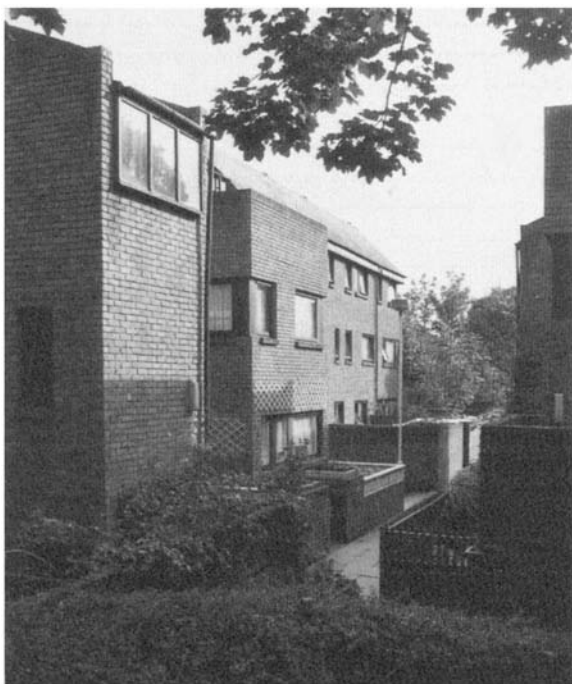
Figure 6.2 psshak housing at Adelaide Road, Camden. The first serious attempt in Britain to apply Habraken's ideas on design participation proved only moderately successful
