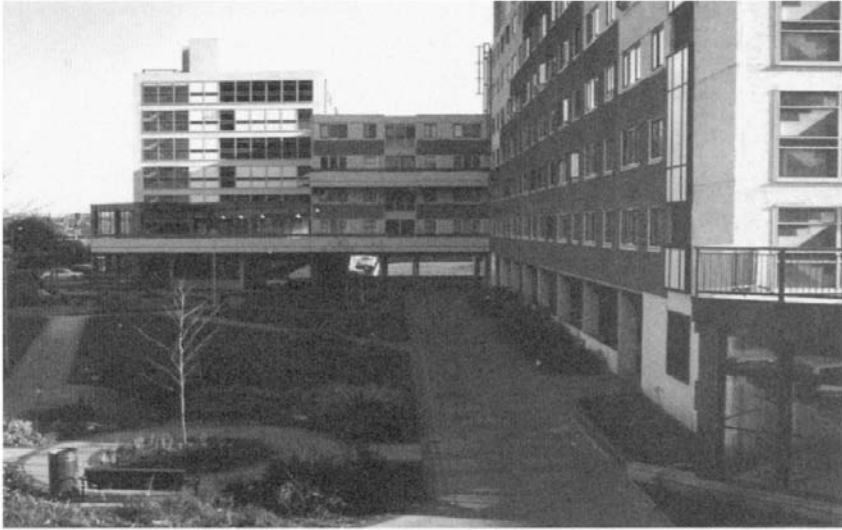
Improvements to the two blocks in the pilot scheme included new windows, recladding and landscaping, transforming their appearance.
