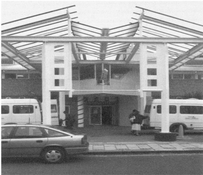
Main entrance. The arrival of ambulances and patients can be observed from the window to the nurses' office on the first floor—nicknamed "the crow's nest".
