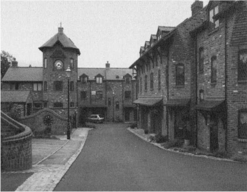
Figure 4.5 Roan Court, Macclesfield New housing built by those who had learned new skills through community self-build.
