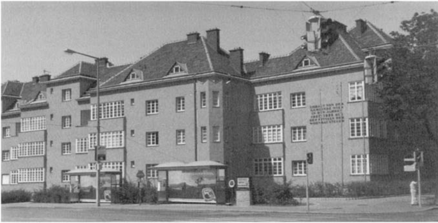
Figure 2.3 George Washington Hof, Vienna. One of the many social housing developments of the 1920s which so inspired visitors from Britain
