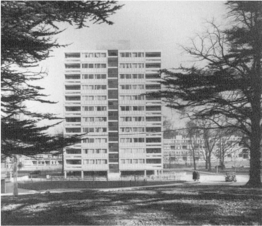
Figure 2.6 The LCC's Alton West Estate, Roehampton, gave credibility to modernist high-rise housing, but its mature landscape set a standard that proved unattainable elsewhere.
