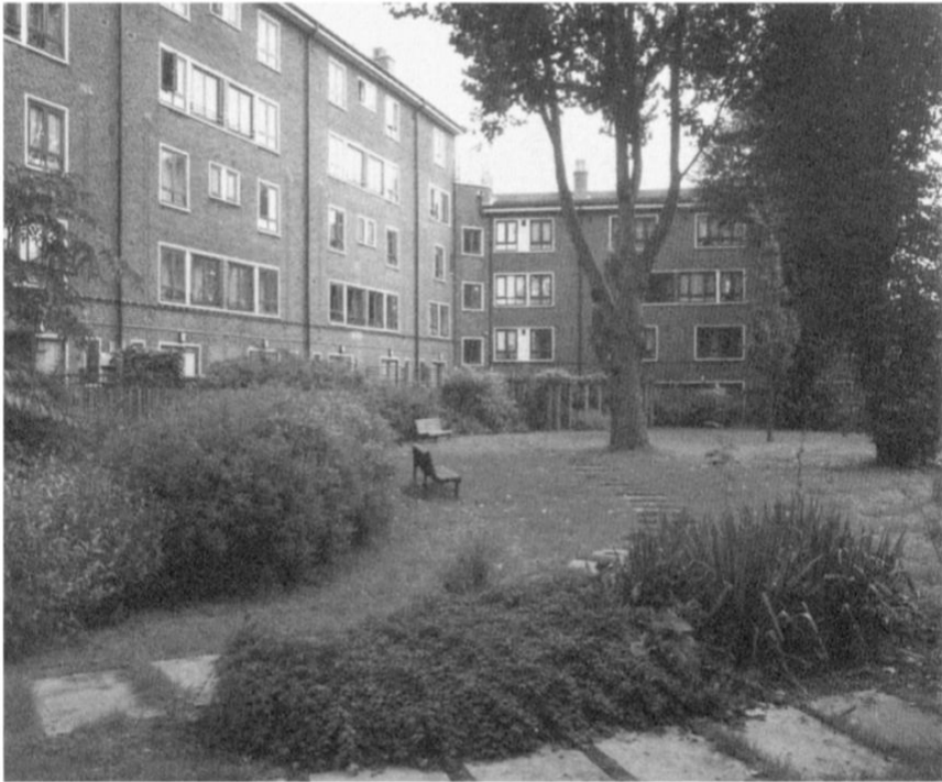
The communal garden to the lower blocks, secured against intruders and accessible only to tenants in the blocks. Adjoining the building are private gardens for the disability flats and lower maisonettes.
