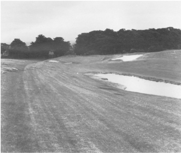
Fig. 2.8 No. 12 green, Mortonhall, Edinburgh, lies on a strong slope away from the approach. Build-up was reduced by limiting front to back measurement and by slight 'cut' at the front edge. (Courtesy of S.R.Jamieson, Edinburgh.)
