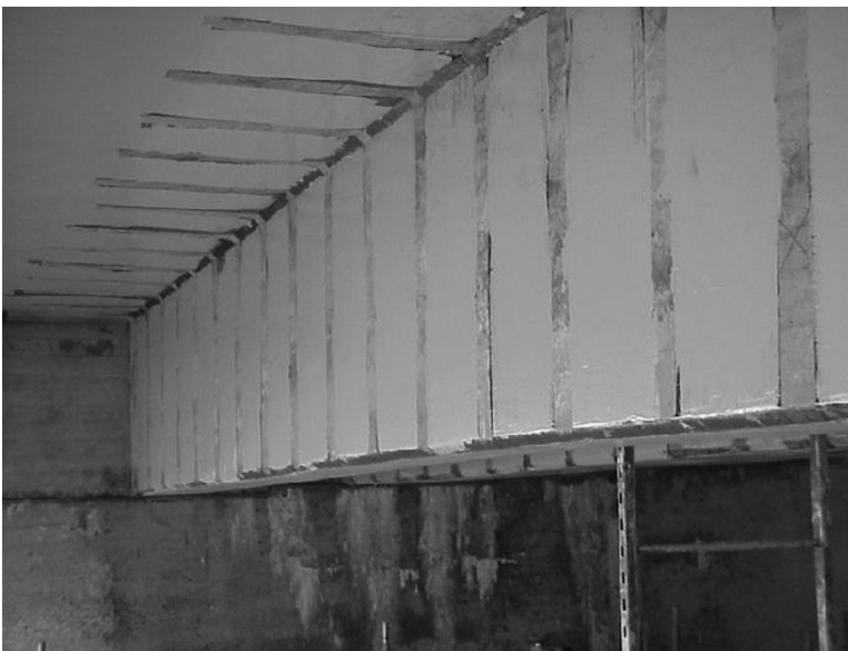
FIGURE 36.11 FRP wrapping of beams to increase flexural strength of bridge T-beams.
