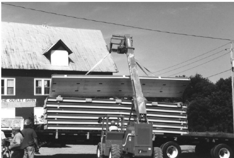
FIGURE 36.9 Sections of FRP deck delivered to construction site on a truck.
