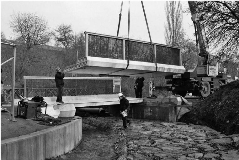
FIGURE 11.11 Installation of Klipphausen Bridge. (Courtesy of Fiberline Composites, Middelfart, Denmark.)
