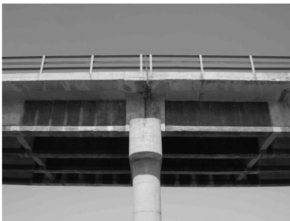
FIGURE 14.8 Shear strengthening using fabrics. (Photo courtesy of Sika Services AG, Pfäffikon, Switzerland.)
