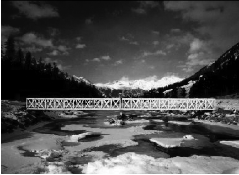
FIGURE 11.14 Pontresina Bridge, Switzerland. (Courtesy of ETH, Zurich, Switzerland; Fiberline Composites, Middelfart, Denmark.)
