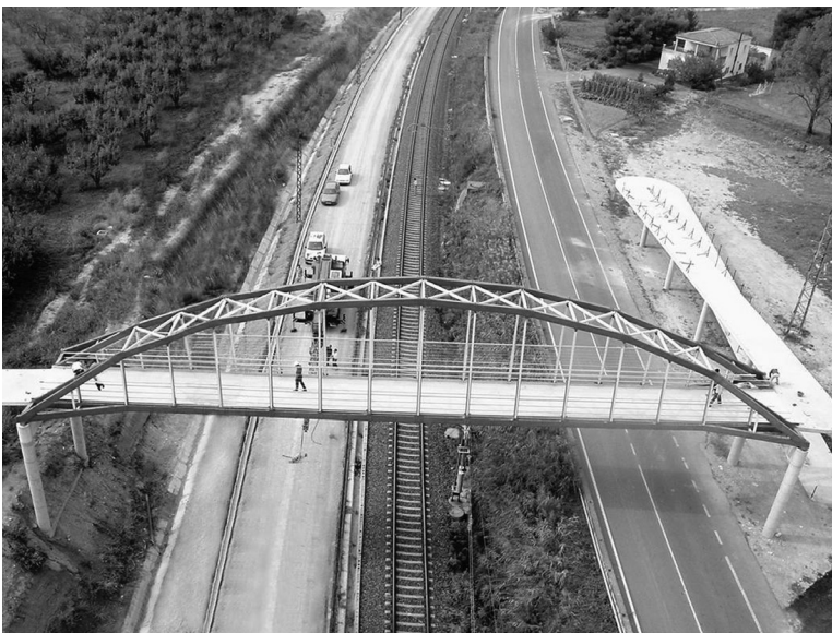
FIGURE 11.15 Lleida Bridge, Spain. (Courtesy of Pedelta, Barcelona, Spain; Fiberline Composites, Middelfart, Denmark.)
