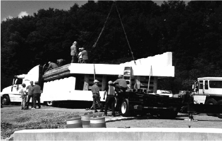
FIGURE 36.5 FRP superstructure delivered to site before installation.
