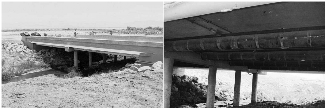
FIGURE 34.6 Kings Stormwater Channel Bridge, San Diego, California.
