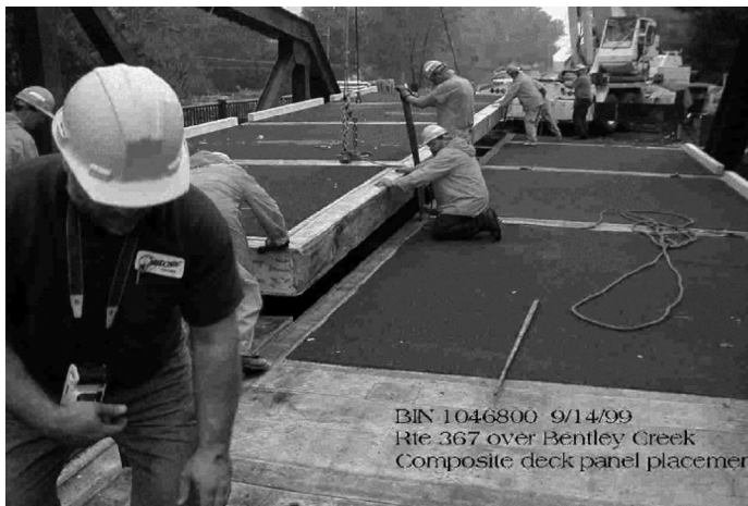
FIGURE 36.4 FRP bridge deck in New York State during installation.
