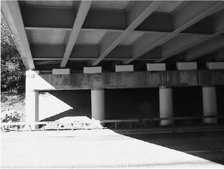
FIGURE 36.10 FRP wrapping to reduce exposure to road salt and inhibit corrosion.
