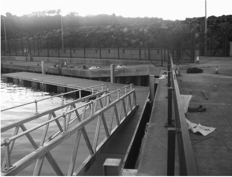
FIGURE 11.31 Jetty walkway, Ireland. (Courtesy of Pipex px ® , Plymouth, U.K.)
