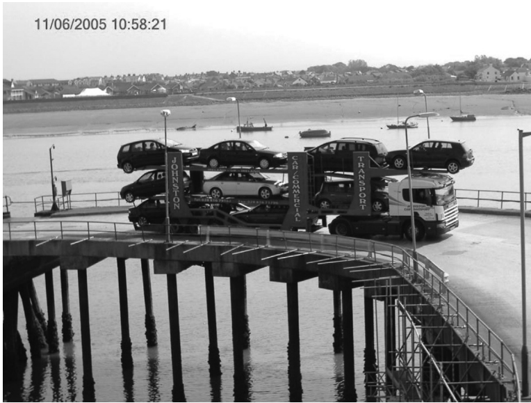
FIGURE 11.27 General view of jetty. (Courtesy of Mouchel Parkman, Leicester, U.K.)
