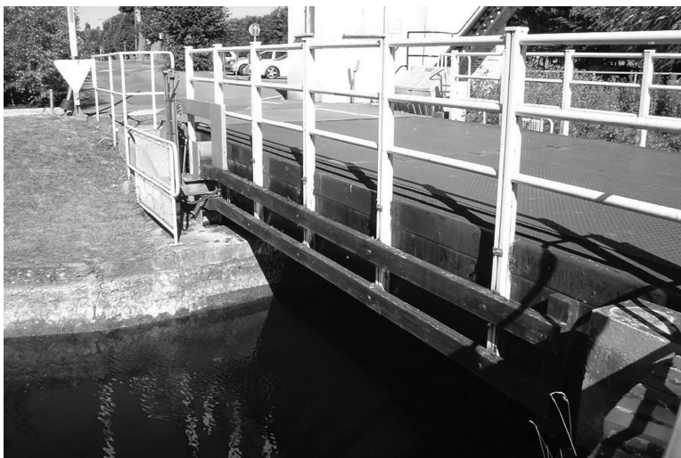
FIGURE 11.8 Bonds Mill Lift Bridge.
