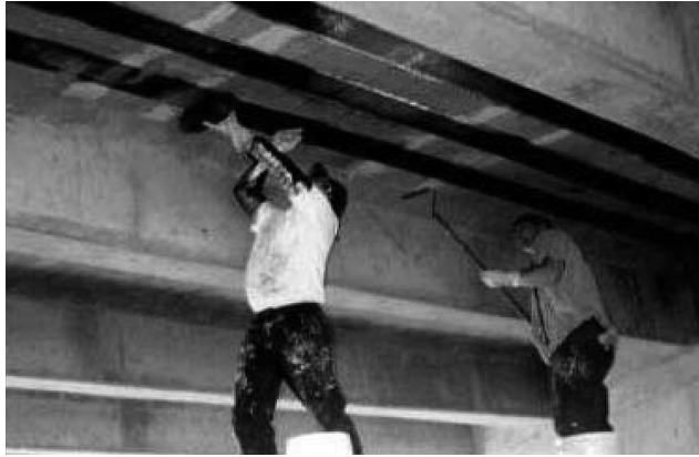
FIGURE 2.2 Bonding of FRP composites to a reinforced concrete bridge deck.
