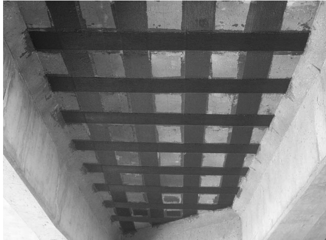
FIGURE 19.1 Bridge deck rehabilitation with externally bonded CFRP composites.
