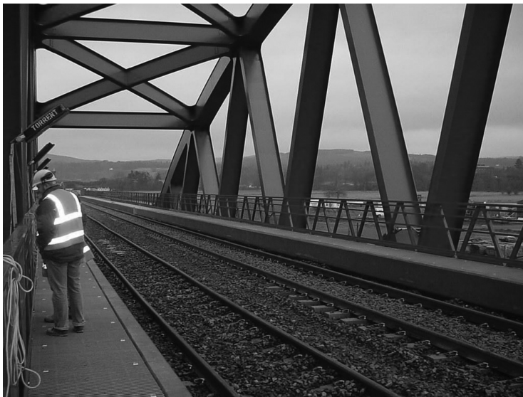
FIGURE 11.30 Parapet walkways for maintenance/inspection access on the railway. (Courtesy of Pipex px®, Plymouth, U.K.)
