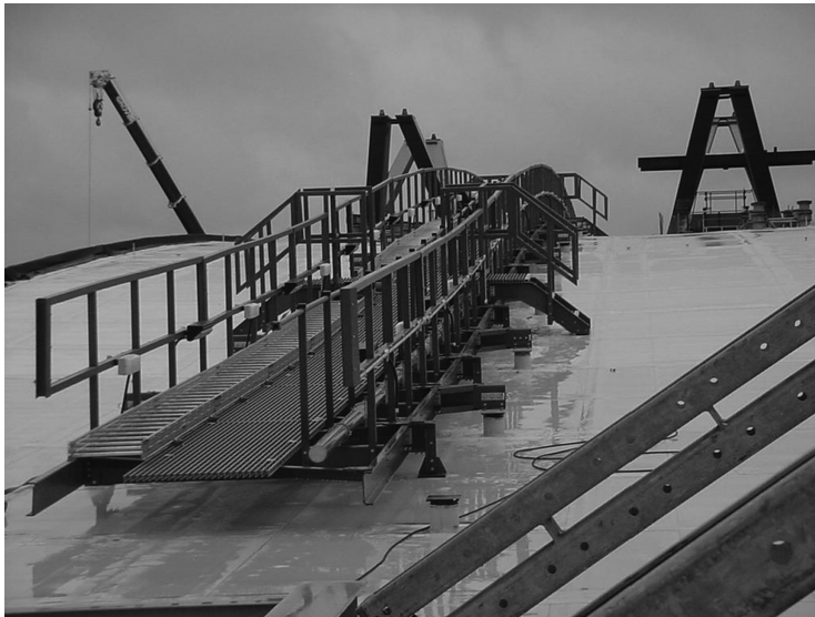
FIGURE 11.32 Roof access walkway, Gatwick Airport. (Courtesy of Pipex px ® , Plymouth, U.K.)
