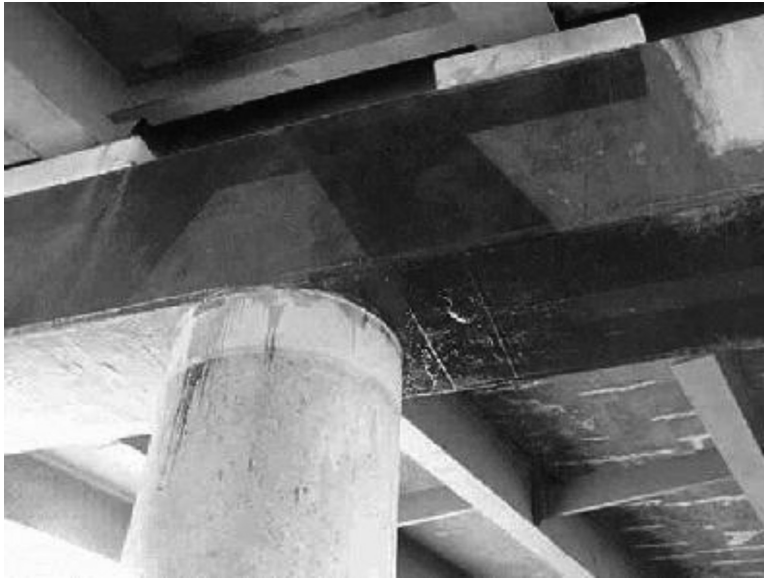
FIGURE 36.12 FRP laminates to increase stiffness of cap beams.
