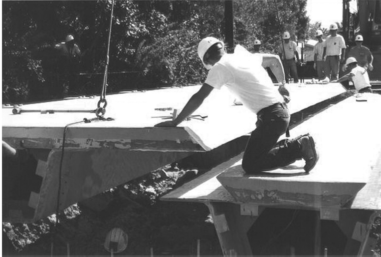
FIGURE 11.25 Construction of “Tech 21” Bridge. (Courtesy of Martin Marietta Co., Bethesda, MD.)
