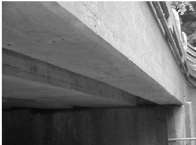
FIGURE 40.6 T-beam bridge side view.
