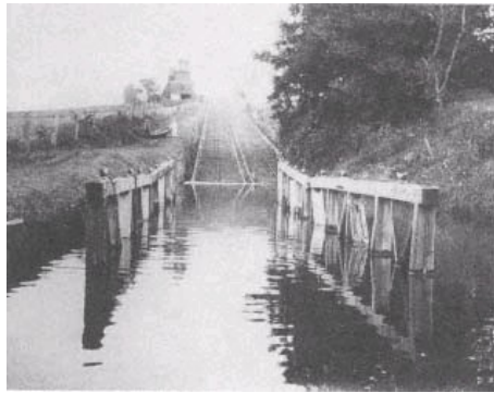
Morris Canal Plane No. 9 West, ca. 1900 with Scotch turbine located in the building at the top of the hill. Library of Congress Collections
