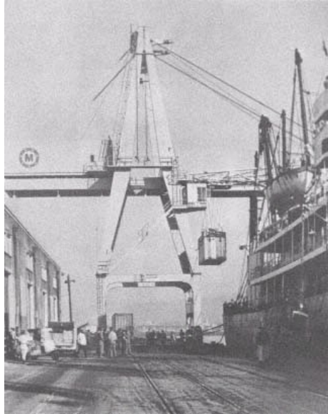
PACECO container crane at Encinal Terminals, Alameda, California, the site of its original installation.
