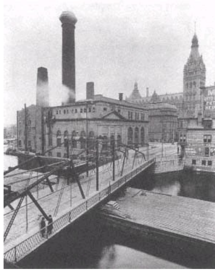
Early twentieth-century view of the Oneida Street Power Plant, site of the first successful use of pulverized coal in utility boilers.
