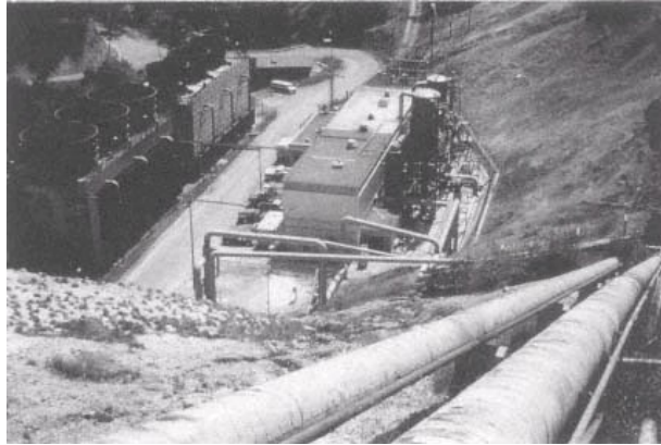
The Geysers Unit I. Courtesy Pacific Gas & Electric Company.
