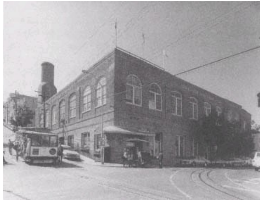
Powerhouse and car barn, Ferries and Cliff House Railway, San Francisco, 1981. Photograph by Jet Lowe, Library of Congress Collections.
