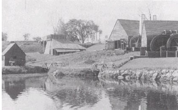
The Saugus Ironworks National Historic Site is a reconstruction of the successful integrated ironworks in North America.
