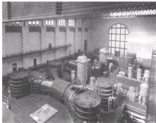
Interior view of the State Line power plant. Courtesy Commonwealth Edison Company.
