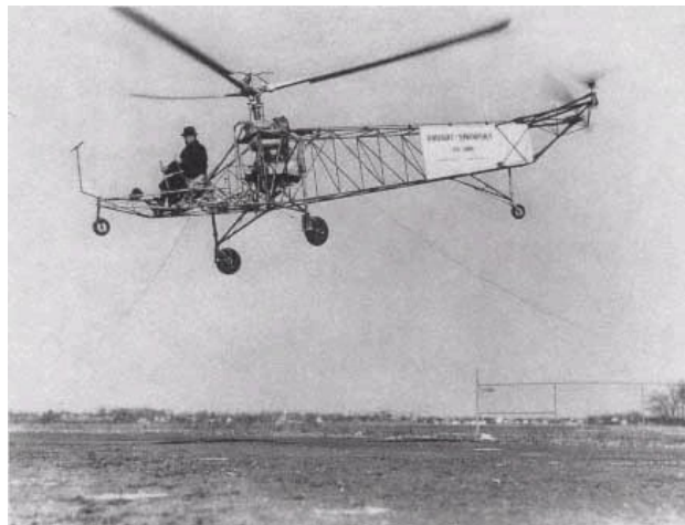
Tethered to the ground, Igor Sikorsky tests his VS-300 helicopter. Courtesy Smithsonian Institution.
