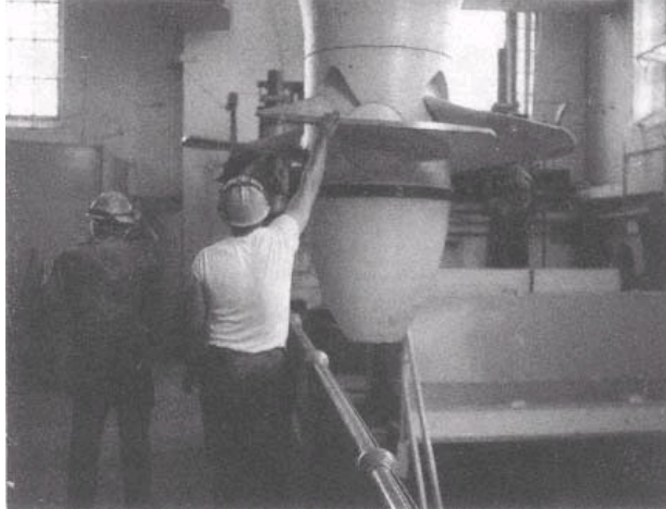
The Kaplan turbine, which resembles a ship's propeller, is shown temporarily removed from its housing for maintenance in 1973.
