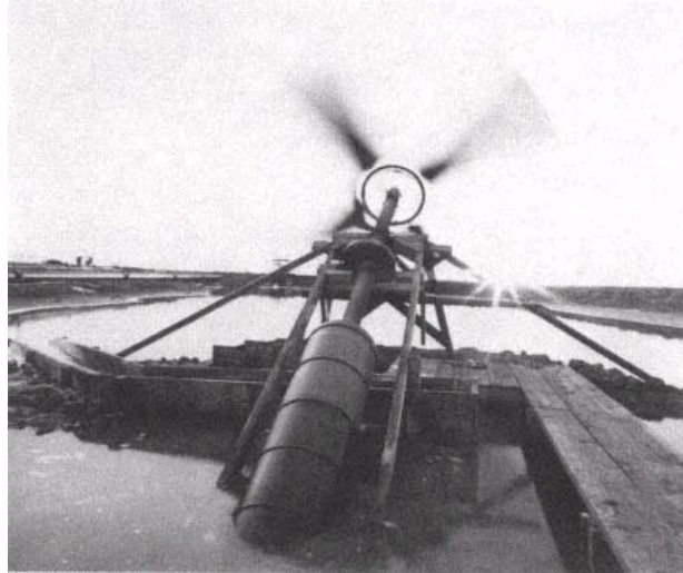
Wind-powered Archimedean screw pumps once served San Francisco Bay salt producers by moving brine from one concentration pond to another.
