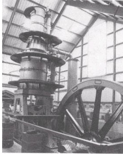
The Chapin Mine pumping engine, the largest steam-driven pumping engine ever built in the United States, was the work-horse of the Chapin Mine from 1892 until 1914.
