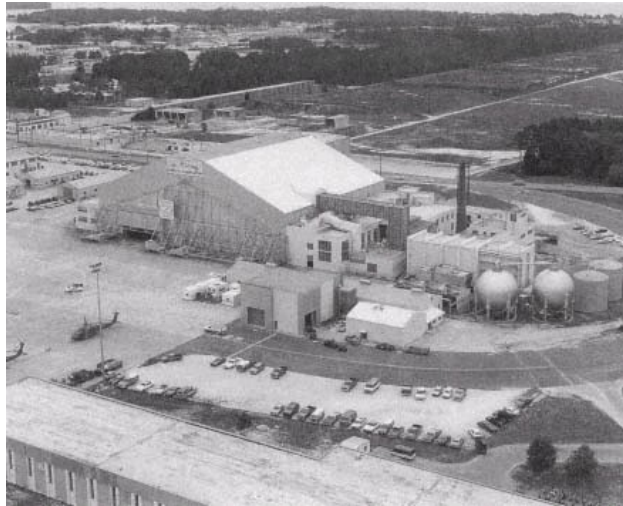
The McKinley Climatic Laboratory, located at Eglin Air Force Base, Florida, is a "weather wonderland," producing Arctic cold, desert heat, and tropical humidity to order. Courtesy Eglin Air Force Base.
