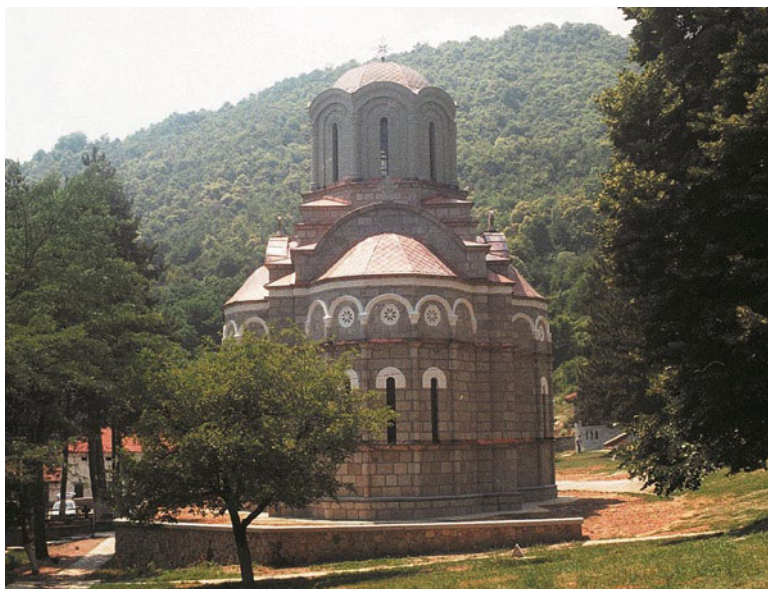
Fig. 12.17 The church after reconstruction
