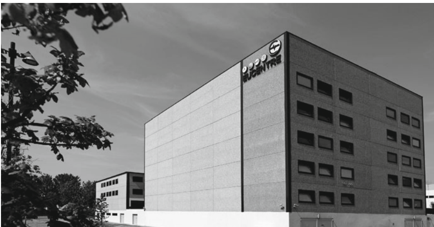
Fig. 4.1 European Centre for Training and Research on earthquake engineering
