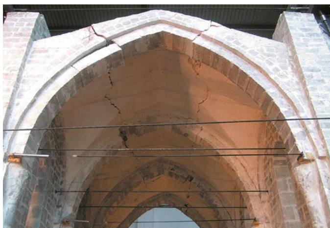
Fig. 12.14 Damage of the model after final test
