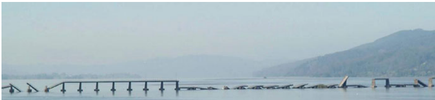
Fig. 8.2 Collapse of Bio-Bio Bridge during the 2010 Chile earthquake
