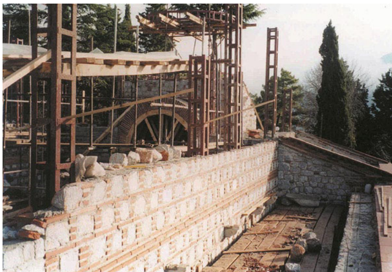
Fig. 12.18 The church during reconstruction
