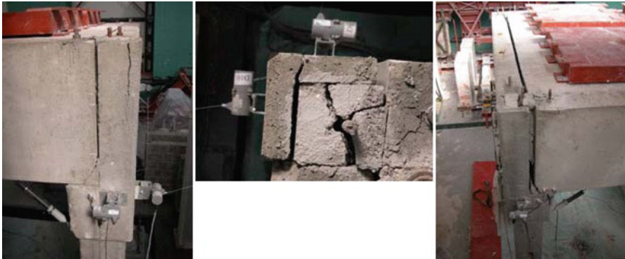
Fig. 18.3 First series of tests, specimens #2 and #3: typical damage at the joints
