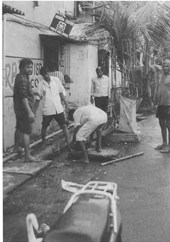
Unclogging the sewers in Sanjay Gandhi Nagar.
