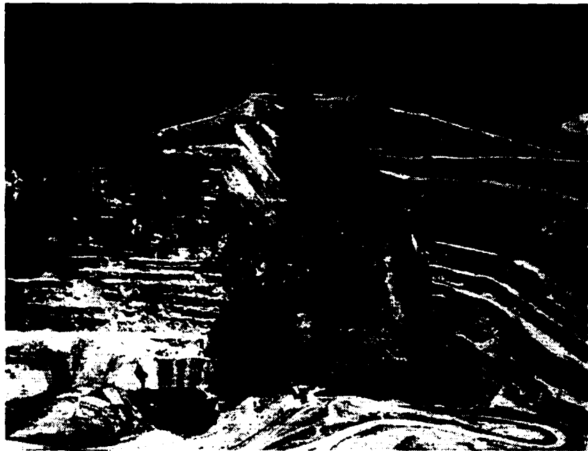
Figure 7.13: The open pit designer is concerned primarily with minimising the risk of overall slope failure. (Kennecott Copper photograph published by Broadbent & Armstrong 187 ).
