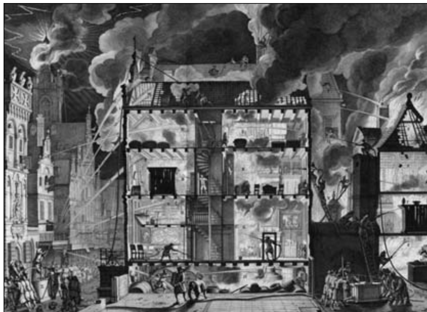
Figure 1.3. New firefighting equipment deployed within a burning townhouse. (Etching from Jan van der Heyden's Fire Hose Book , 1690, plate 2. Reproduced by permission of the New York Public Library, Astor Lenox and Tilden Foundations, Rare Books Division.)
