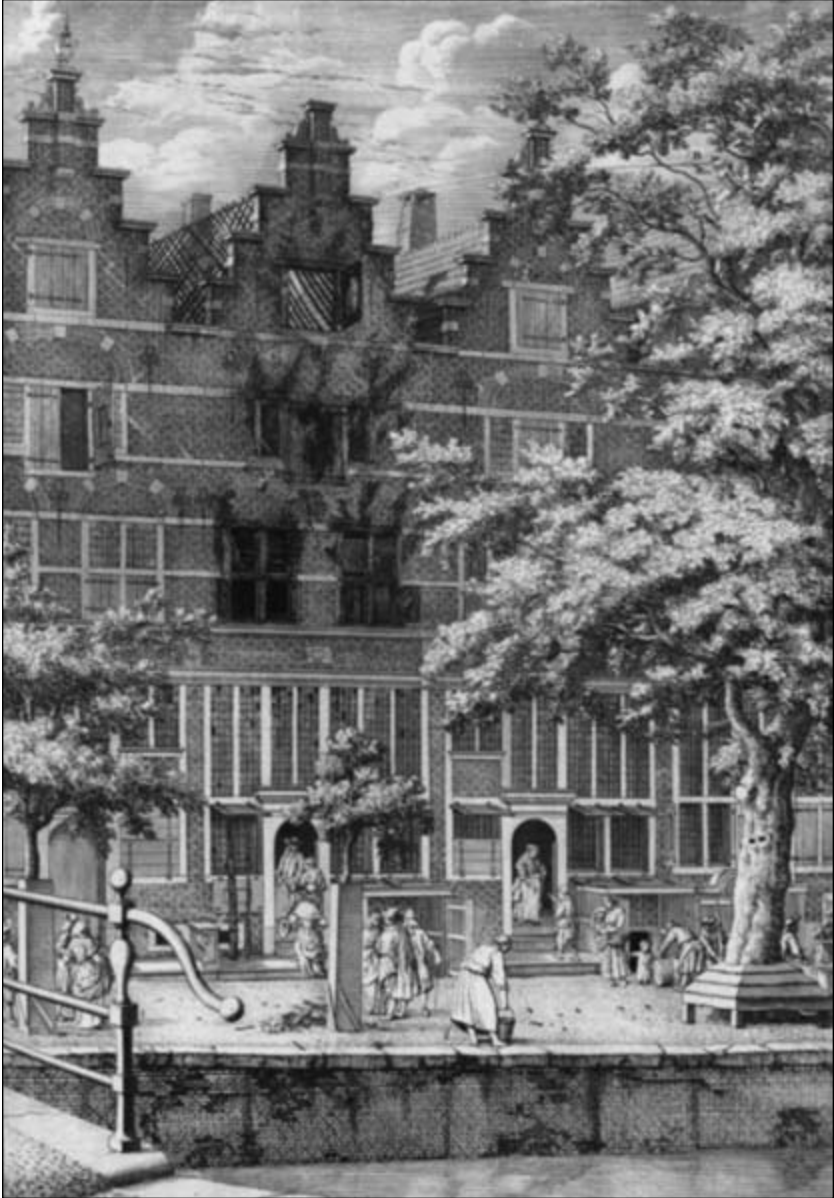
Figure 1.7. Aftermath of a fire in a townhouse on the Herengracht, April 25–26, 1683. (Engraving from Jan van der Heyden's Fire Hose Book , Amsterdam, 1690, plate 13. Reproduced by permission of the New York Public Library, Astor Lenox and Tilden Foundations, Rare Books Division.)
