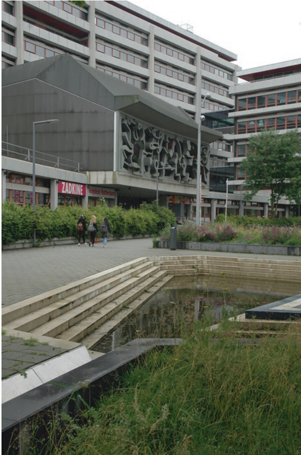
Figs. 2.6 and 2.7 Rotterdam has employed a variety of urban design strategies to retain and control water. Shown here is the Bethemplein—a so-called “water plaza” that serves to collect and retain rainwater, but on sunny days adds a public space to the neighborhood. Image credit: Tim Beatley
