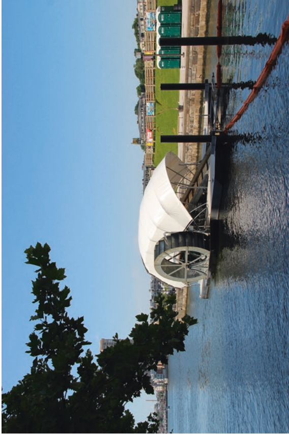
Fig. 2.3 Mr Trash Wheel, shown here, is located in the inner harbor of Baltimore, Maryland, where it utilizes river current and solar energy to collect waste and debris. Image credit: Adam Lindquist, Healthy Harbor Initiative
