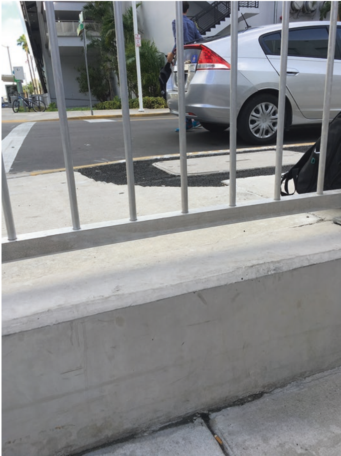
Figs. 2.4 and 2.5 Miami Beach has been elevating roads in neighborhoods such as Sunset Beach, shown here. It creates an interesting physical disconnect between street level and storefront entrances, and sometimes, as shown on the right, a sheltered seating area for customers. Image credit: Tim Beatley
